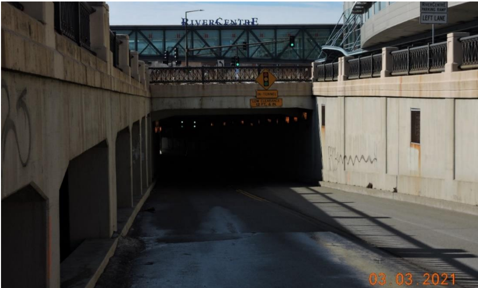
Existing Exchange Street viaduct and retaining wall - photo taken viewing west
