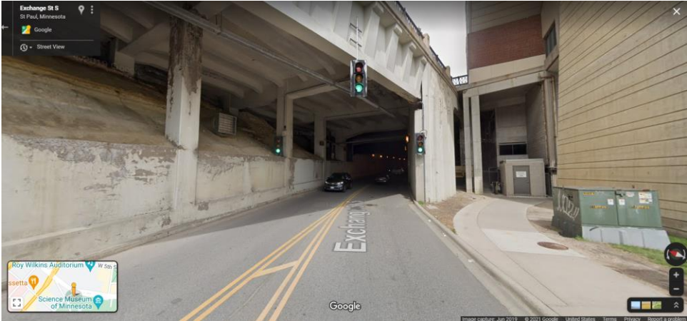
Currently, Exchange Street carries two vehicular lanes under Bridge No. 90378. The sidewalk on Exchange Street terminates right before entering the viaduct. The project will explore ways to improve pedestrian facility and safety through the viaduct. Image viewing east.
