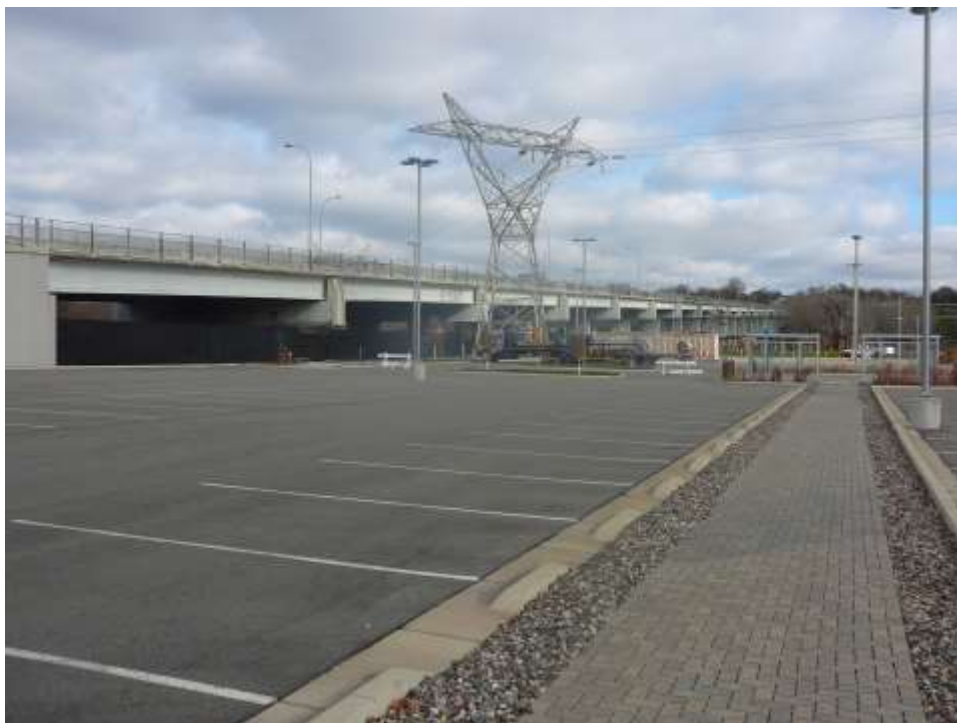
Existing Bridge – View from Union Depot Lot – Looking East
