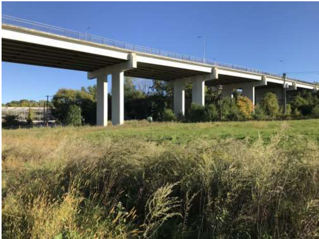
Existing Bridge Pier – View From Bruce Vento Sanctuary – Looking Northwest
