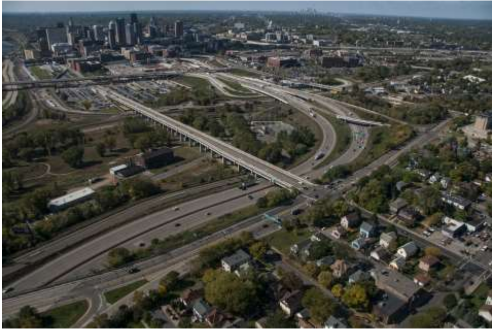
Existing Bridge – Looking West
