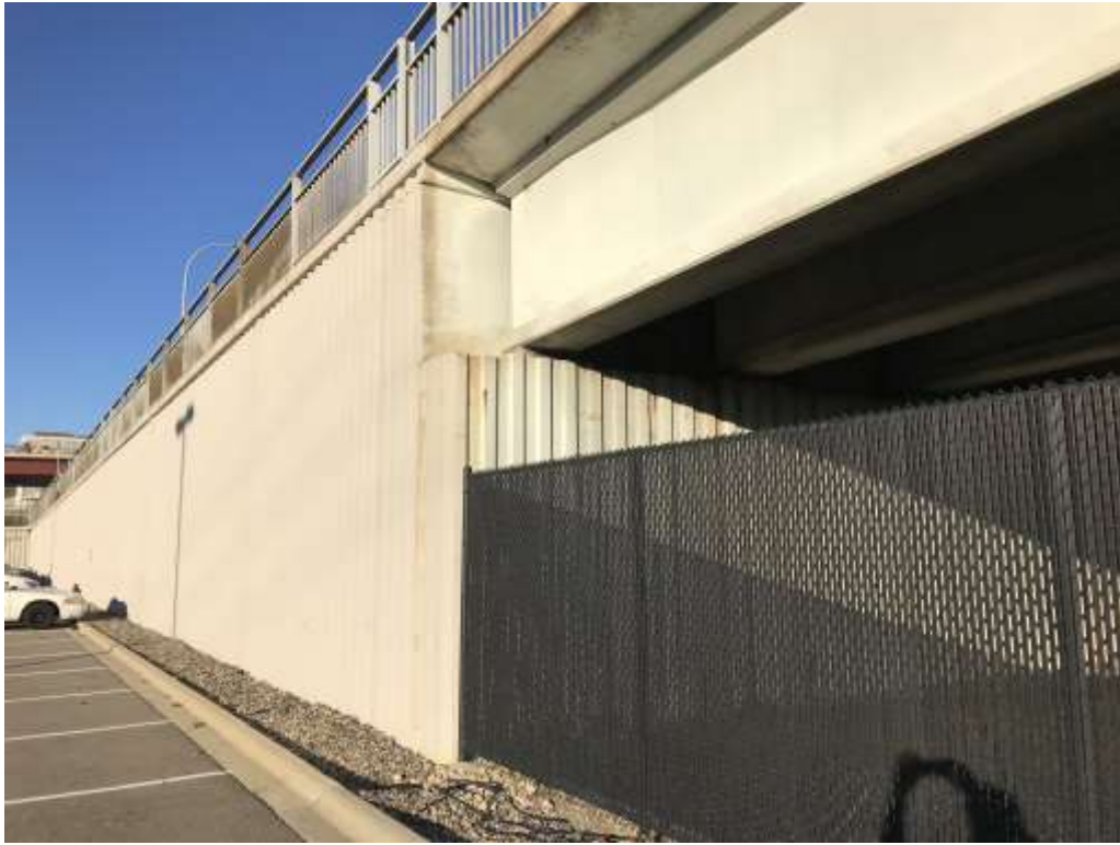
Existing Retaining Wall – View form Union Depot Lot
