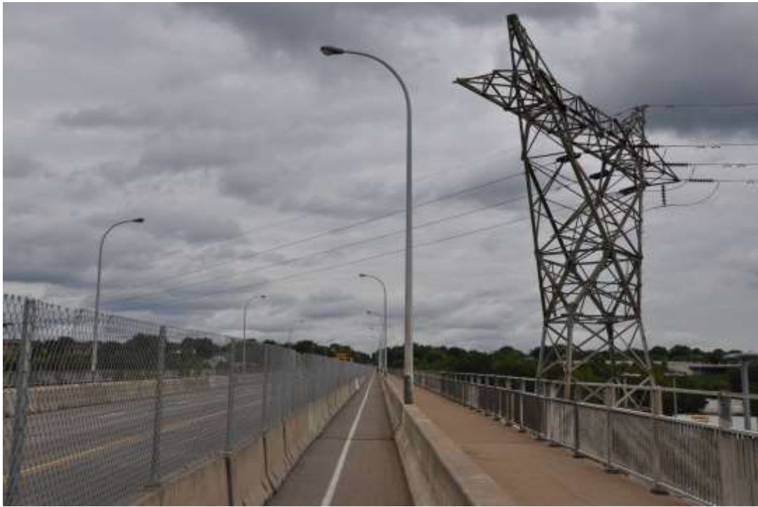
Existing Bridge Sidewalk – Looking East
