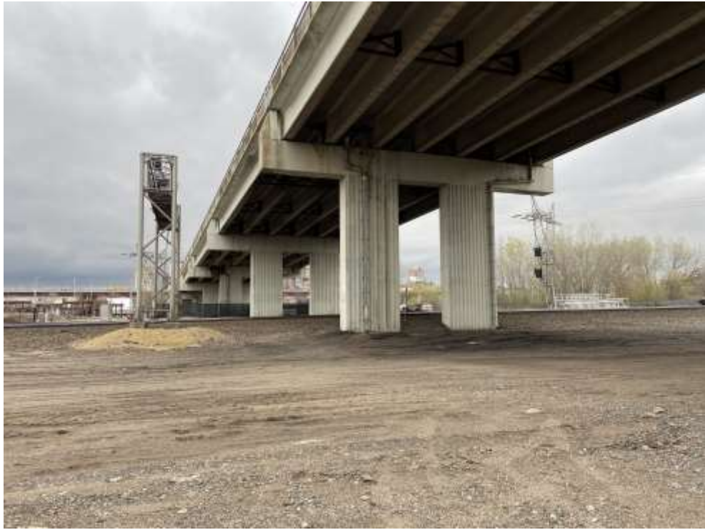
Existing Bridge Pier – View From Bruce Vento Sanctuary – Looking West
