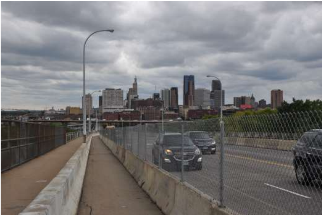
Existing Bridge Sidewalk – Looking West
