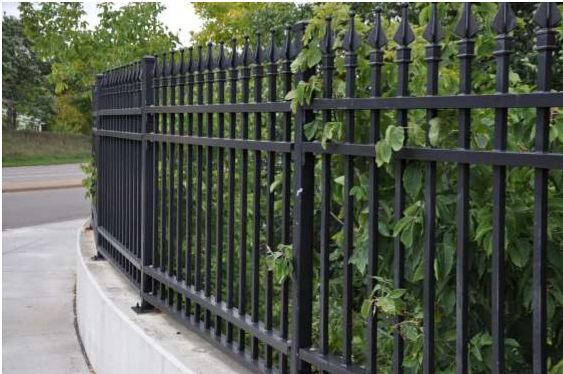
Existing Railing at Mounds Blvd. – Looking West
