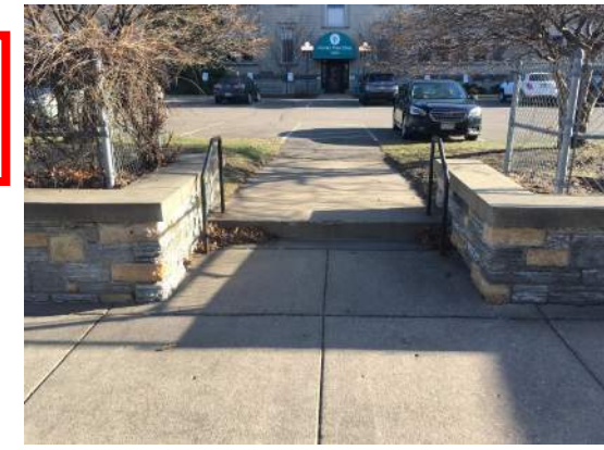
Existing Wall Opening @ North Elevation
