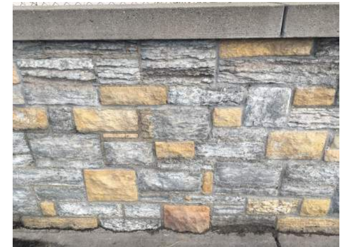
EXISTING WPA RETAINING WALL
