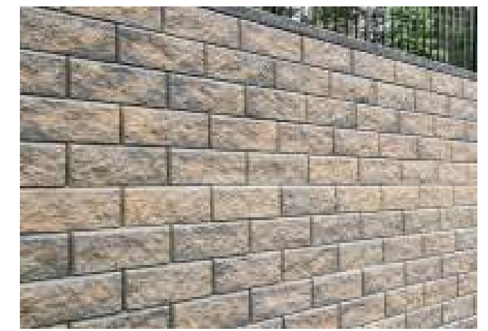
PROPOSED MODULAR BLOCK RETAINING WALL
