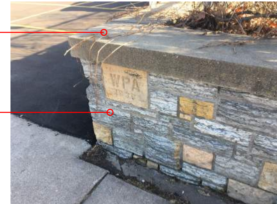
Existing Wall @ Northeast Corner
