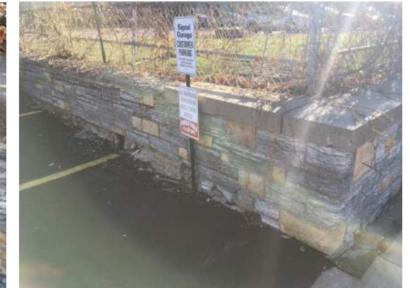
Existing Wall @ Northeast Corner
