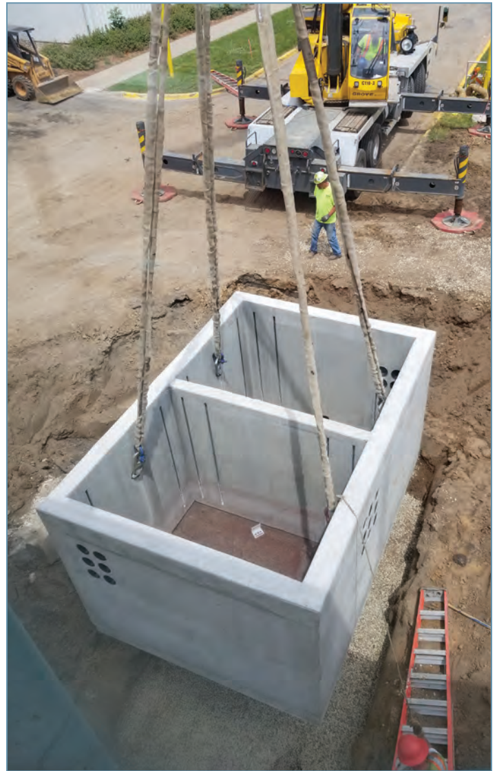
Photos: Above: Structures for the new electrical equipment go into place below ground.
