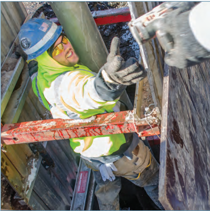
SPRWS workers repair a water main break..
