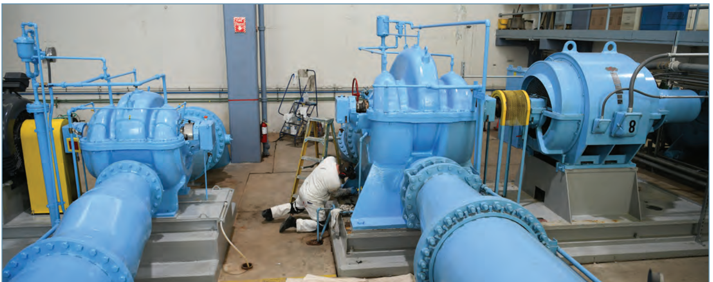
Below: Pumps being painted in the treatment plant.
