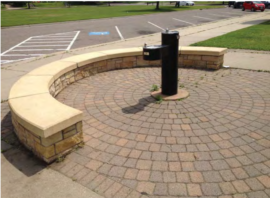
Kasota stone with cast stone cap seat wall and colored concrete pavers at Mounds Park Overlook
