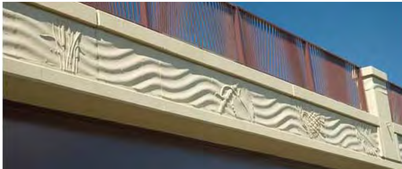
Cast concrete balustrade with sculptural railing by Myklebust + Sears
