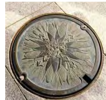
Cast bronze mile marker set in concrete sidewalk
