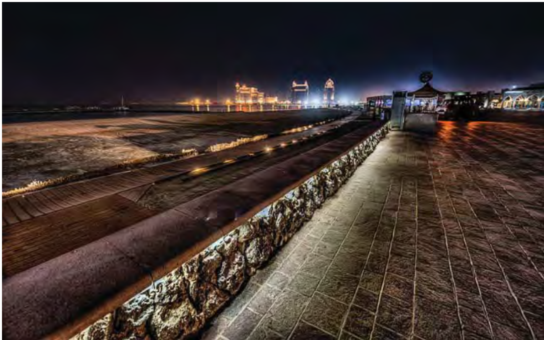
LED lighting under wall cap
