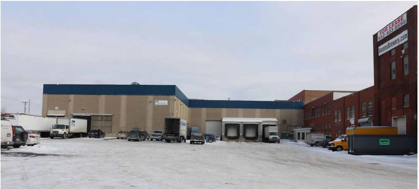
RA-SPC-2926, February 1, 2019, Building 65, west elevation, looking east.
