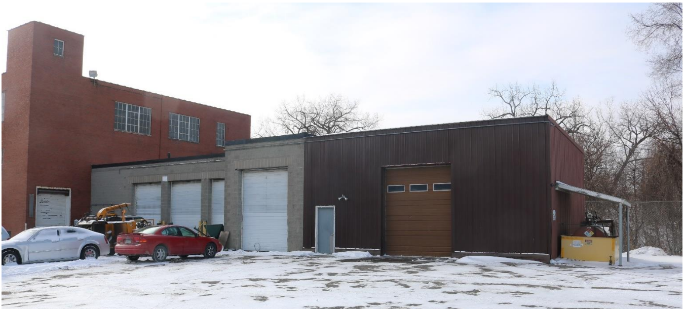
RA-SPC-2926, February 1, 2019, Building 69, east and north elevations, looking southwest.
