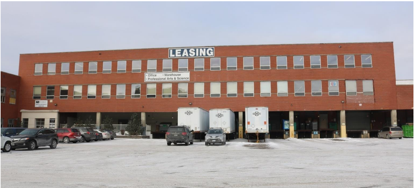
RA-SPC-2926, February 1, 2019, Building 38, south elevation, looking north.
