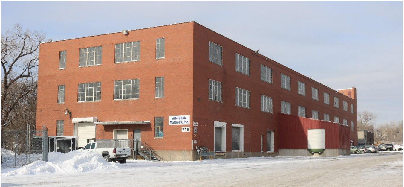
RA-SPC-2926, February 1, 2019, Building 45, south and east elevations, looking northwest.
