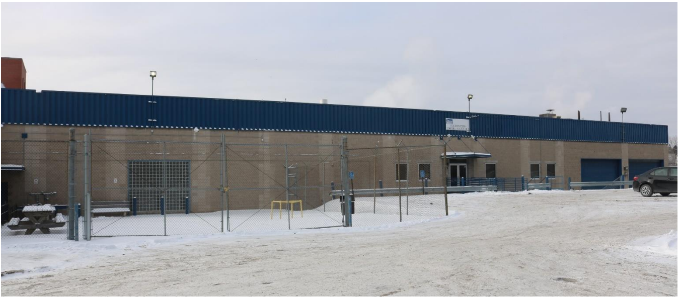
RA-SPC-2926, February 1, 2019, Building 65, east elevation, looking west northwest.
