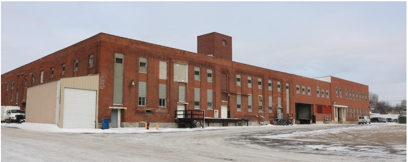
RA-SPC-2926, February 1, 2019, Building 41, south and west elevations, looking northeast.
