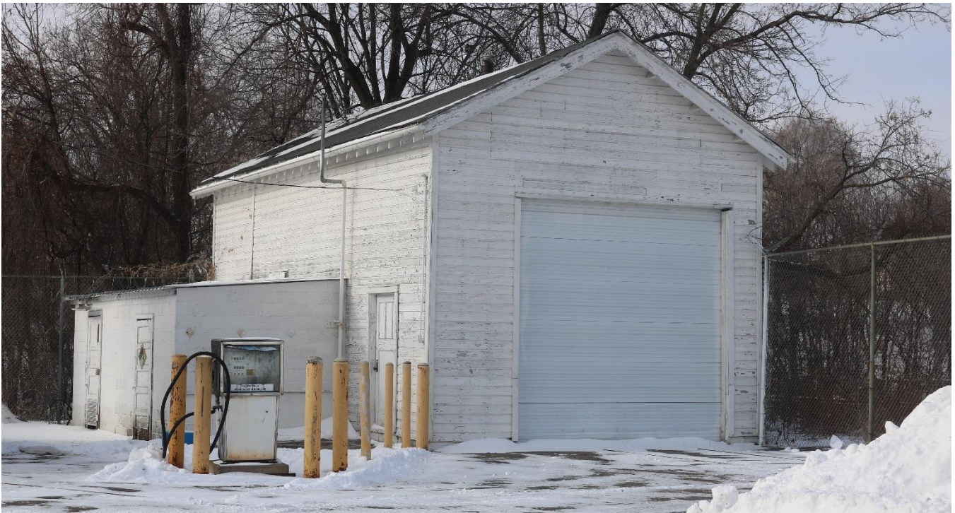
RA-SPC-2926, February 1, 2019, Building 40, south and west elevations, looking west.
