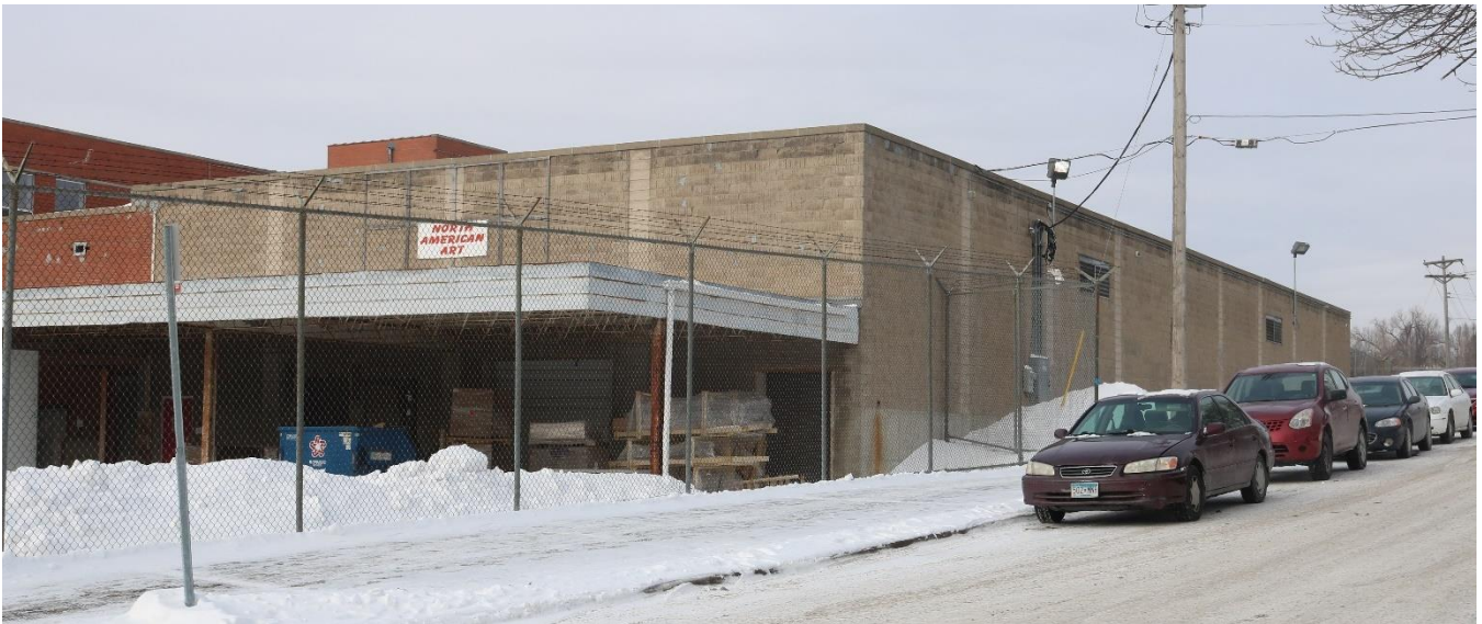
RA-SPC-2926, February 1, 2019, Building 67, south and east elevations, looking northwest.
