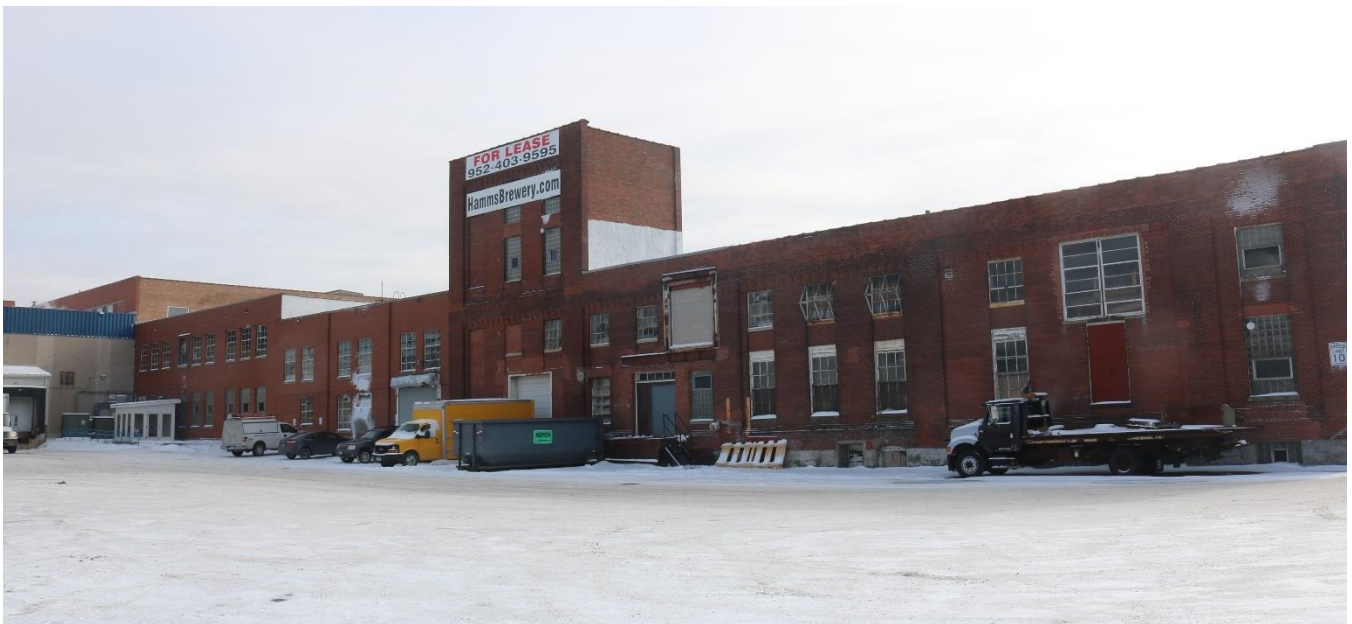
RA-SPC-2926, February 1, 2019, Building 41, north elevation, looking southeast.
