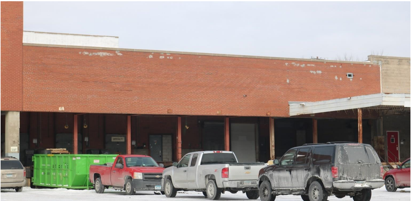
RA-SPC-2926, February 1, 2019, Building 61, south elevation, looking north northeast.
