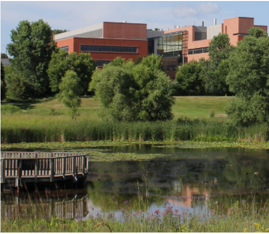
C : WETLANDS Three existing and two new wetland areas will provide flow and rate control for treated stormwater from the District Stormwater feature.
