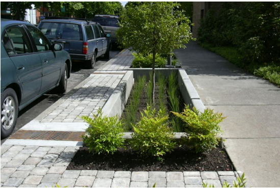
D: TREE TRENCH B Tree trenches are encouraged to be located between the public road and public sidewalk in the neighborhood node. In areas adjacent to medium and higher density residential development and/or in areas with adjacent parking, the tree trenches will be designed to support safe pedestrian circulation.
