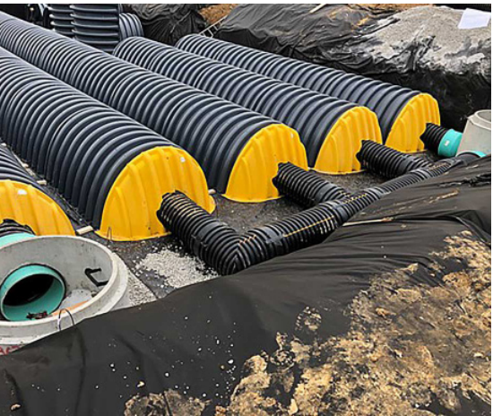
B : UNDERGROUND STORAGE Highly impervious light industrial and residential sites may use underground storage methods to effectively manage the sites' stormwater loads.
