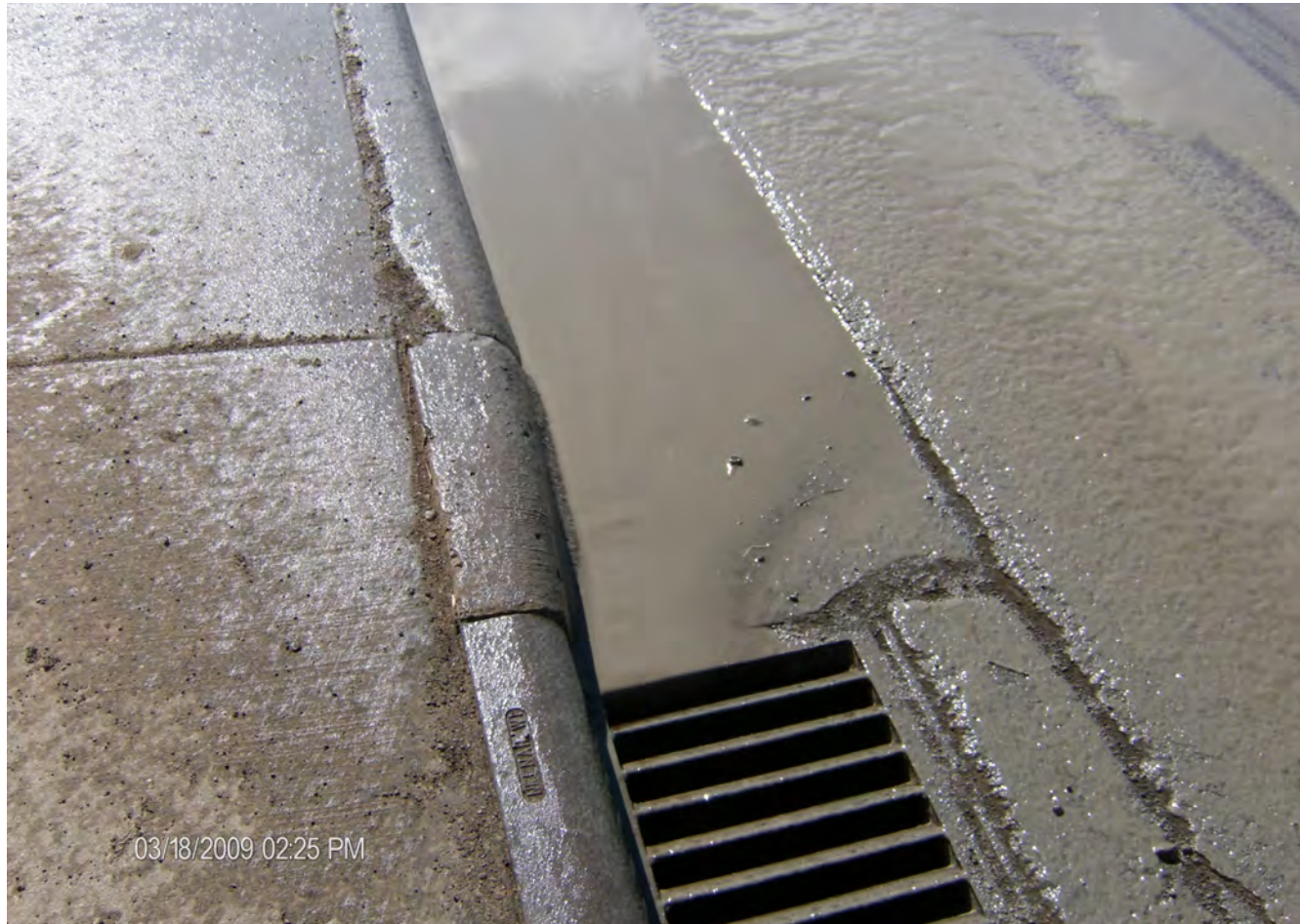
Discharge of Drilling Mud
