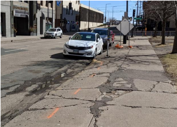
The pavement, sidewalks, curbs, and utilities need to be replaced. Photo taken in April 2021.
