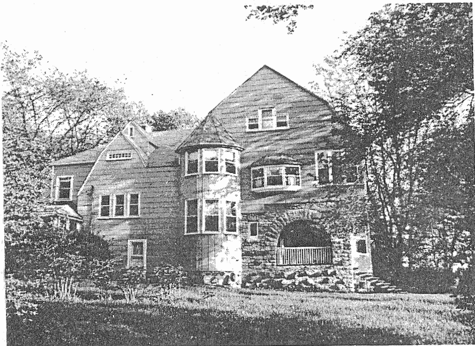
1. 882 S. Point Douglas Road, Charles E. Joy House, 1888, designed by Charles E. Joy. (Photo by Gary Phelps)
