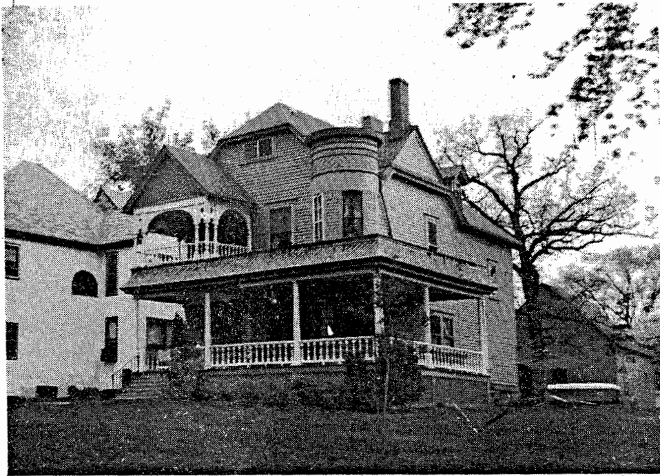
14. 1269 W. Como Boulevard, House built for Cary Warren of the Warrendale Improvement Company, 1886, designed by Augustus F. Gauger. (Photo by Gary Phelps)
