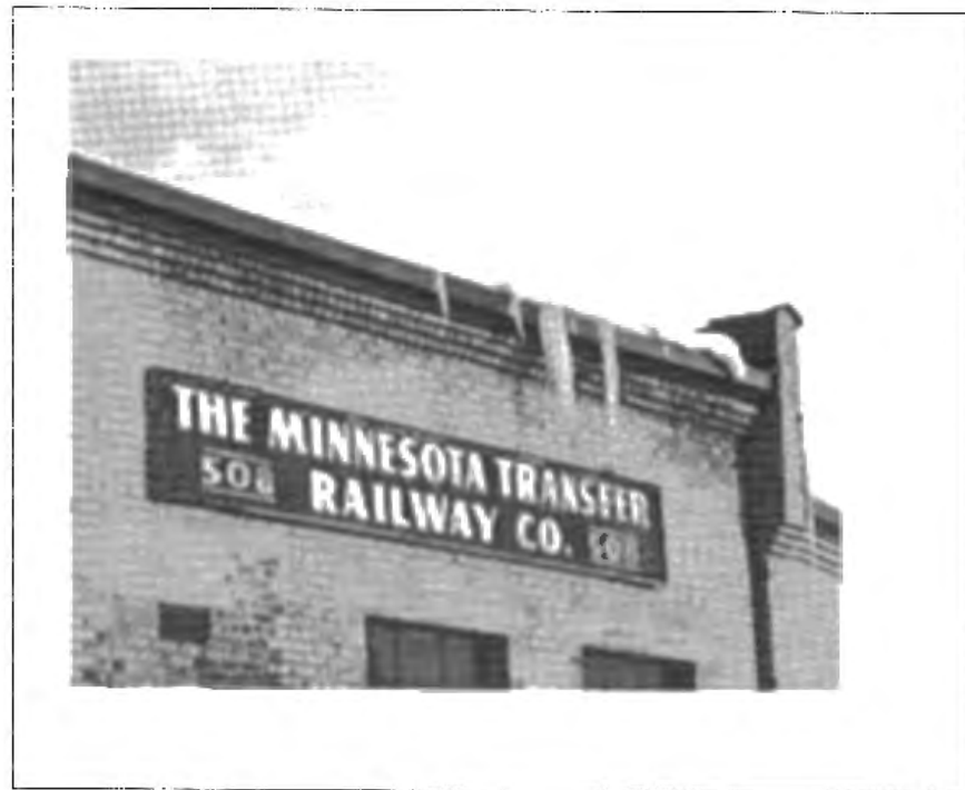
Minnesota Transfer Railway Co. Roundhouse, 508 Cleveland Avenue, 1891-1907
