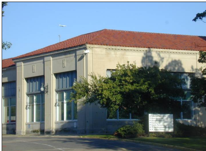
The northwest corner of the plant, which was the location of the historic salesroom, is relatively intact.
