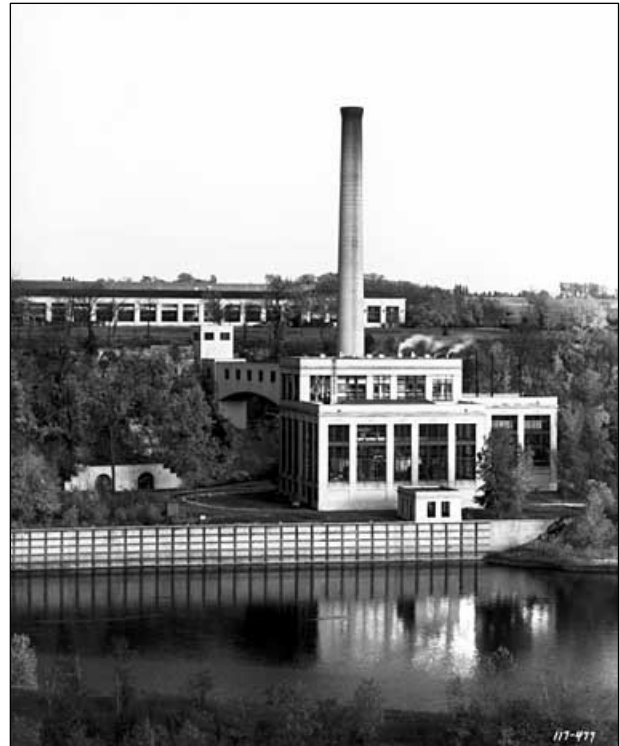
An enclosed bridge connected the steam plant to an underground conveyor that carried coal from the east side of the assembly plant. The tunnel entrance and barge dock are also shown in this 1936 photograph. (Minnesota Historical Society)
