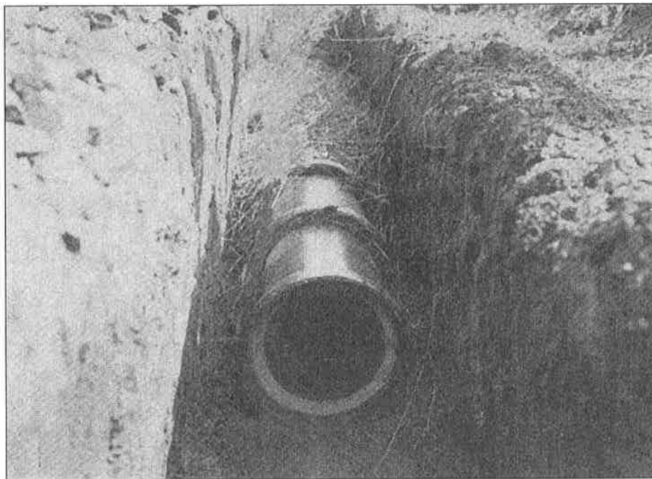
Figure 12. Tile pipe for drainage (Howson 1926:123)
