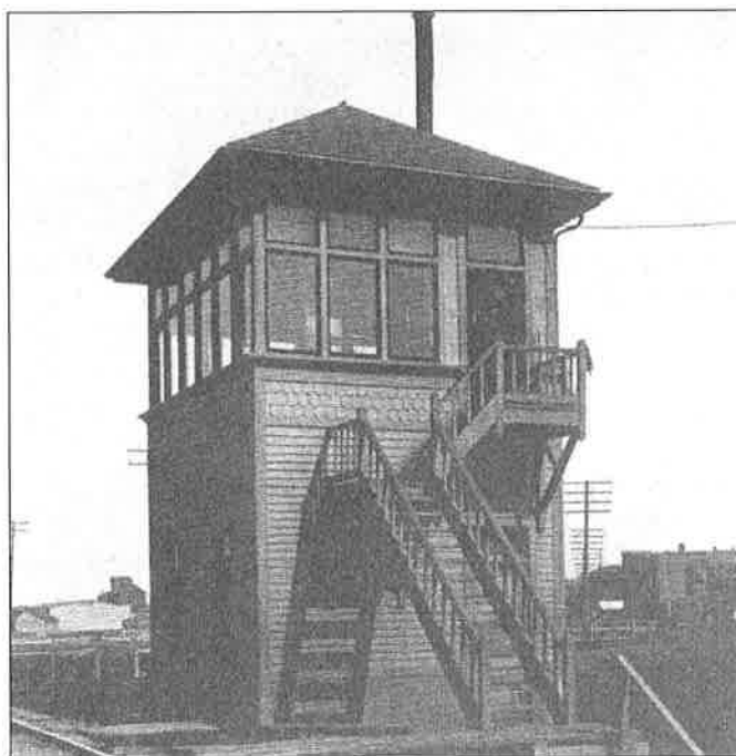
Figure 28. Interlocking tower (Howson 1926:792)
