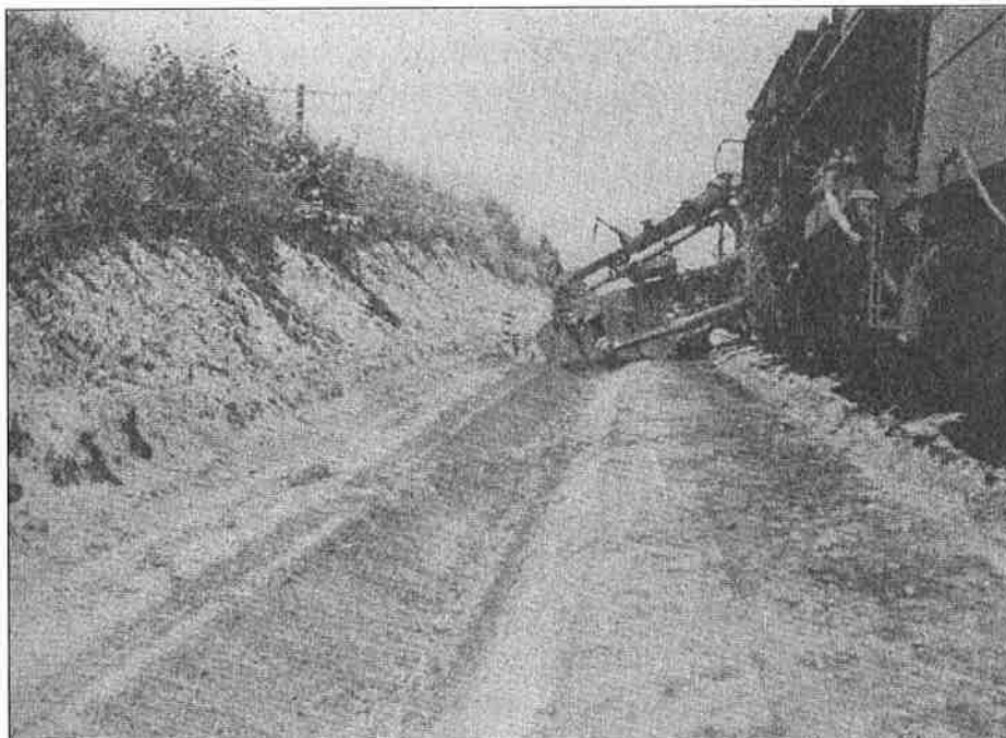
Figure 11. Construction of drainage ditches (Rench 1946:21)
