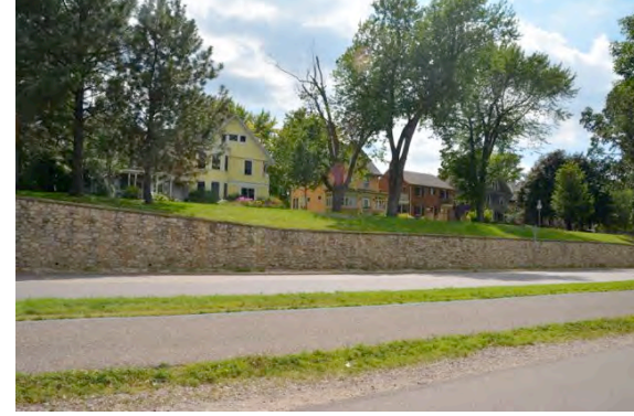
Figure 42. Residential block overlooking west side of Lake Como.
