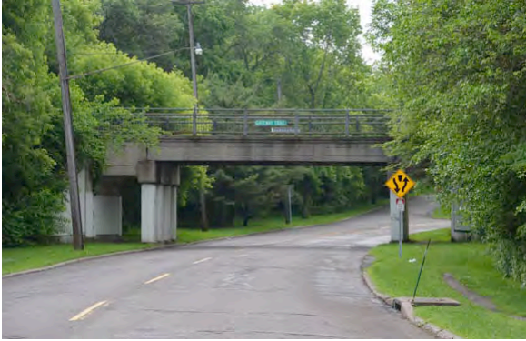
Figure 37. Soo Line Bridge, 1938 (Gateway Trail) facing east.
