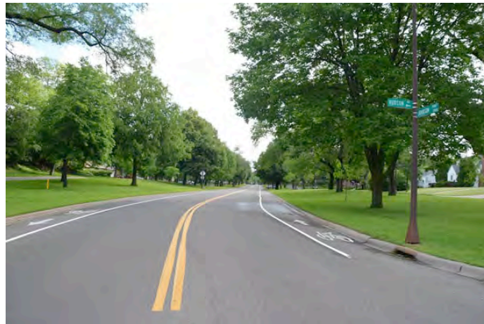
Figure 26. Johnson Parkway at Hudson Street, looking north.
