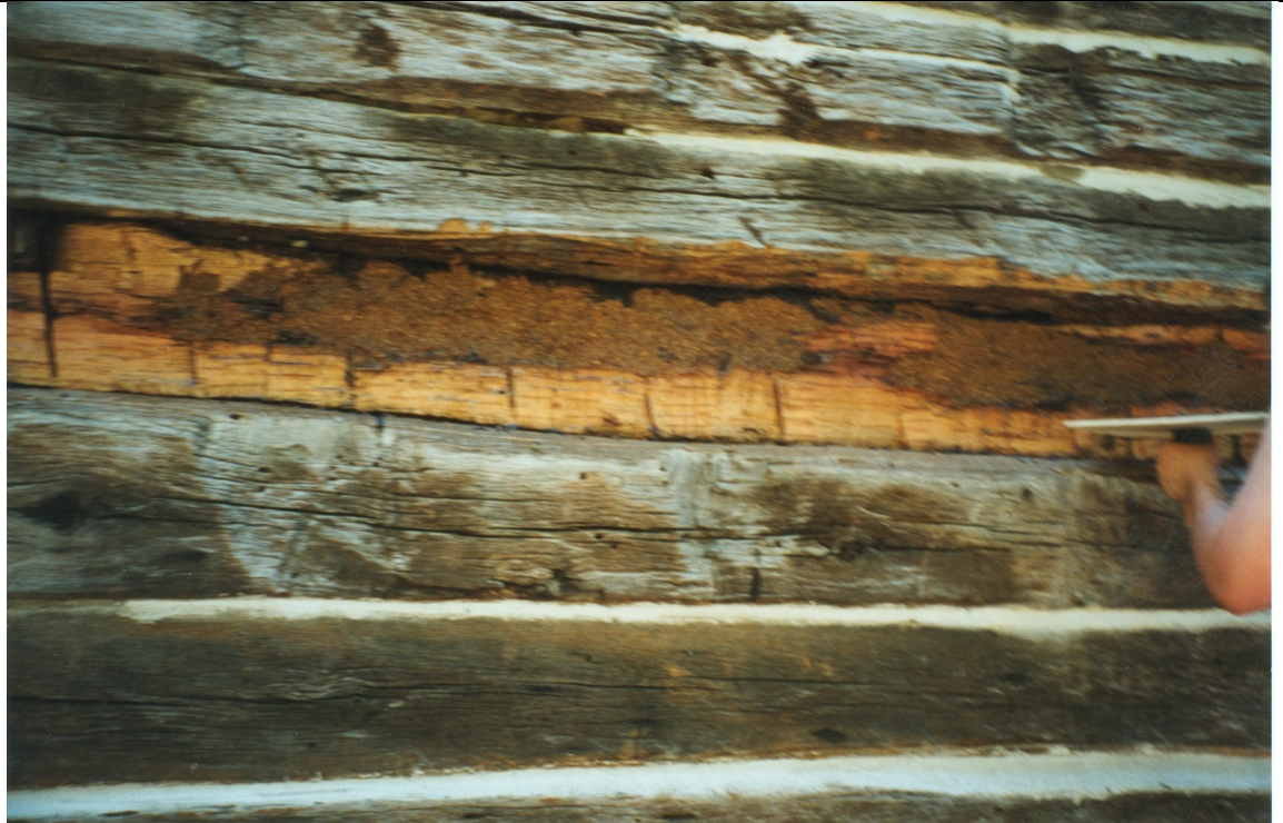
Exterior repairs, using log fill. 1994 Luther Seminary Archives.
