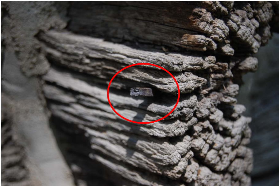
Figure 5. One of several square nails remaining embedded in the log structure.
