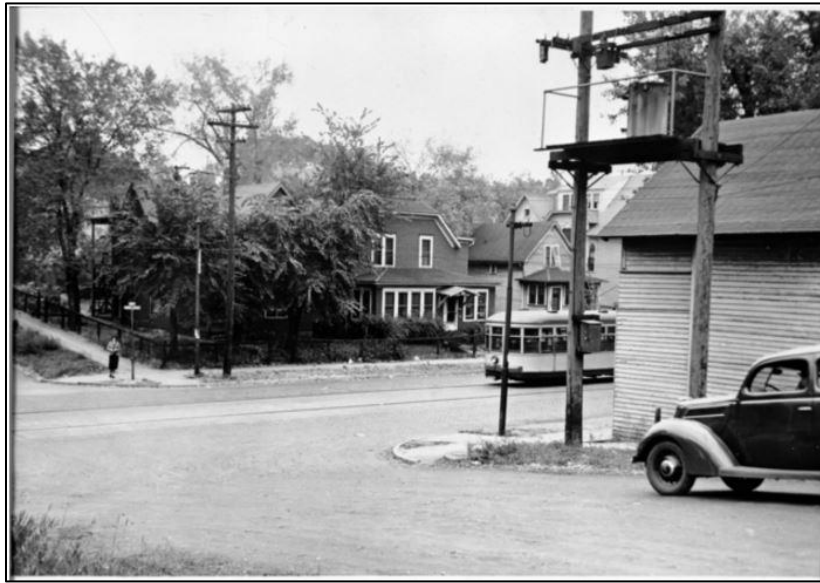
Figure 11. Rondo Avenue at Arundel Street, Rondo neighborhood c. 1940 (MNHS 1940a)
