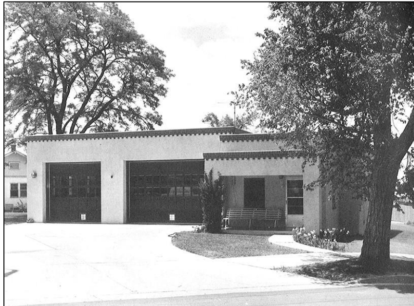
Figure 9. Fire Station 2, Albuquerque, New Mexico, built 1937 46
