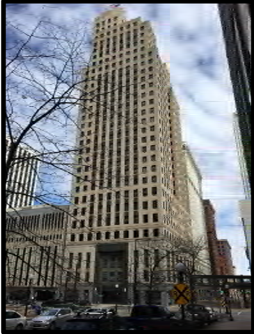
First National Bank Building, East
