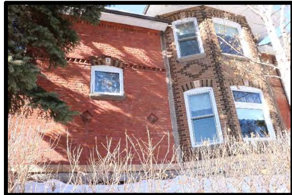
103 East King Street, Window Detail
