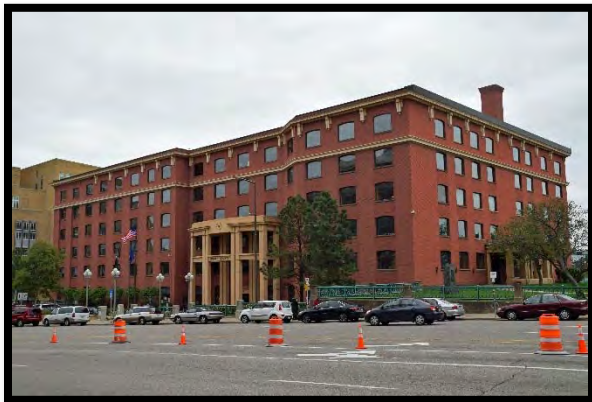
Farwell, Ozmun, Kirk and Co. Building, Southeast
