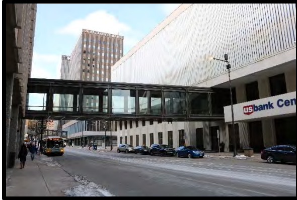
Bridge No. 91249, West
