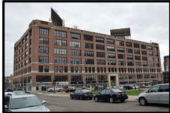
Foot Schulze Building, East
