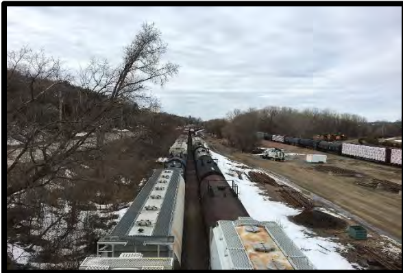
CGW RR Corridor at Butler Ave E, North
