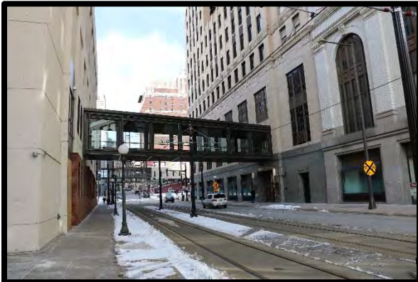
Bridge No. 91247, West
