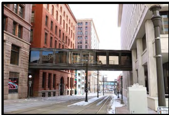
Bridge No. 92616, East
