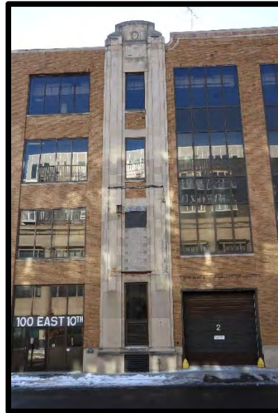
Tri-State Warehouse, South
