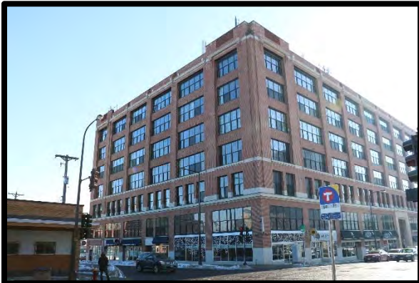
Foot Schulze Building, Southeast
