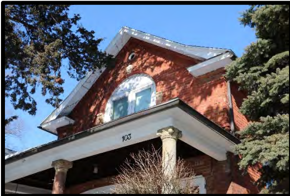
103 East King Street, Window Detail
