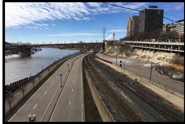
CM&StP Railroad Corridor, West
