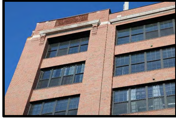
Foot Schulze Building, Window Detail
