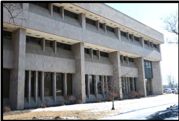
Minnesota State Bank of St. Paul, Window Detail
