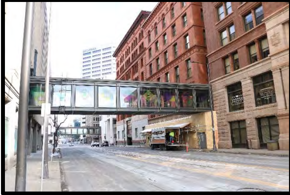
Bridge No. 92716, North
