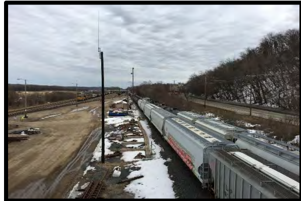
CGW RR Corridor at Butler Ave E, South
