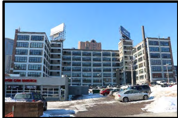
Foot Schulze Building, West
