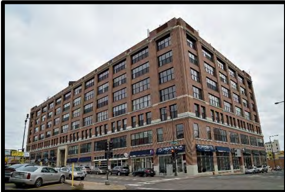
Foot Schulze Building, Northeast
