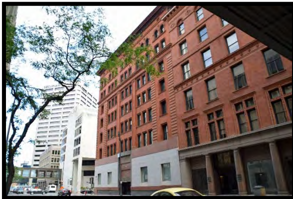
Manhattan/Empire Building, Northeast
