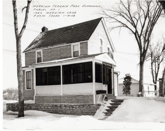
Figure 61. 1942 Merriam Lane, razed for park expansion, ca. 1968 (RCHS)
