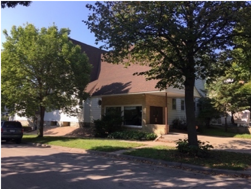
Figure 25. Merriam Park Presbyterian Church, 1982 Iglehart Avenue (1890).
