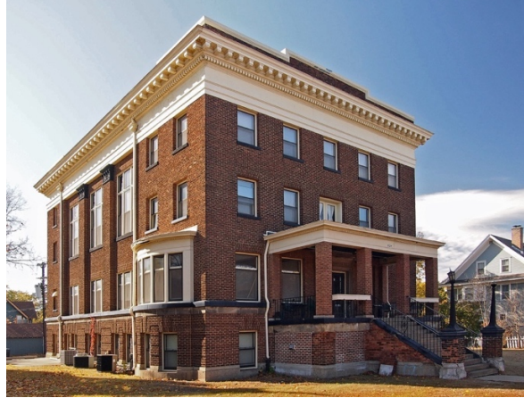
Figure 55. Charles Thompson Memorial Hall, 1824 Marshall Avenue (1916).
