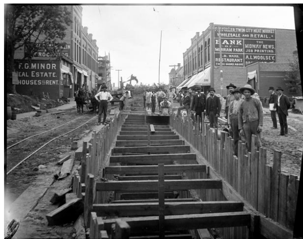
Figure 47. Prior Avenue construction, ca. 1900.
