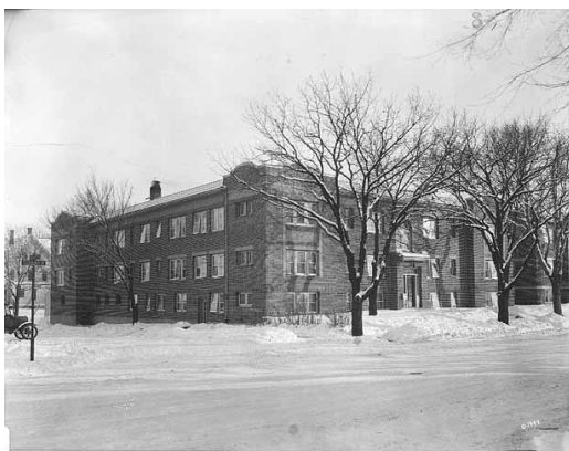
Figure 51. The Cleveland, 372 Cleveland Avenue (1925), facing southeast in ca. 1930.
