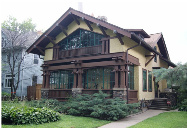
Figure 45. Den E. and Cornelius Lane House, 2000 Marshall Avenue (1910; Dean Nelson photo).
