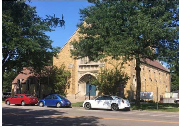
Figure 30. Trinity Methodist Episcopal Church, 1849 Marshall Avenue (1913).
