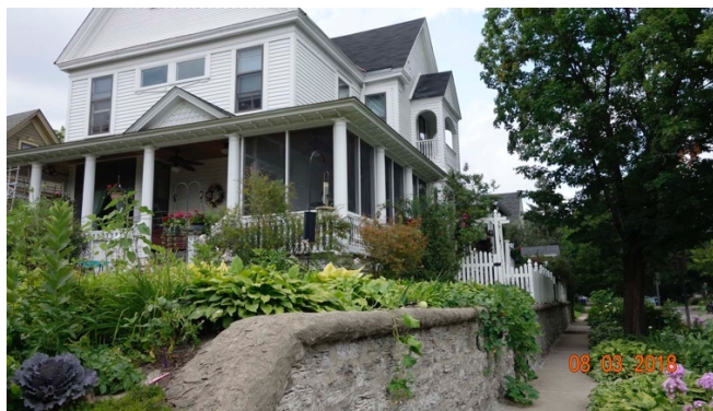
Figure 23a. 1919 Iglehart, detail of limestone wall.
