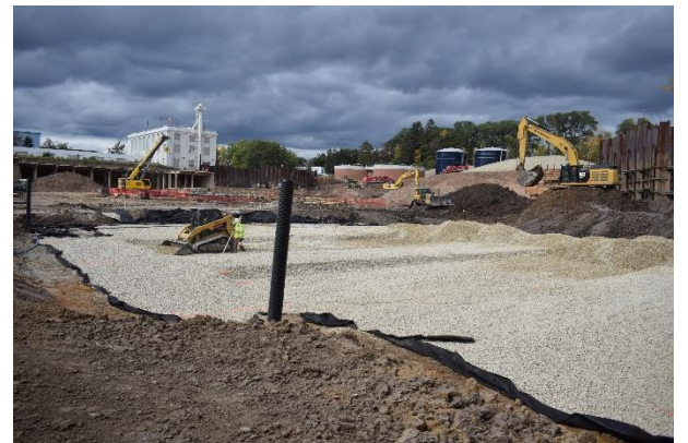
Preparation the base of the Ozone/Recarb area
