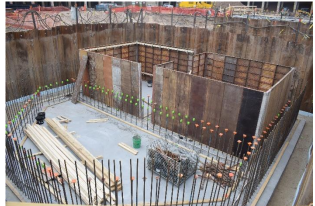
West Sludge Pit under construction
