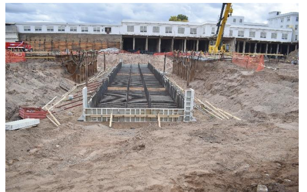
Preparation of 6 ft. diameter pipe bedding
