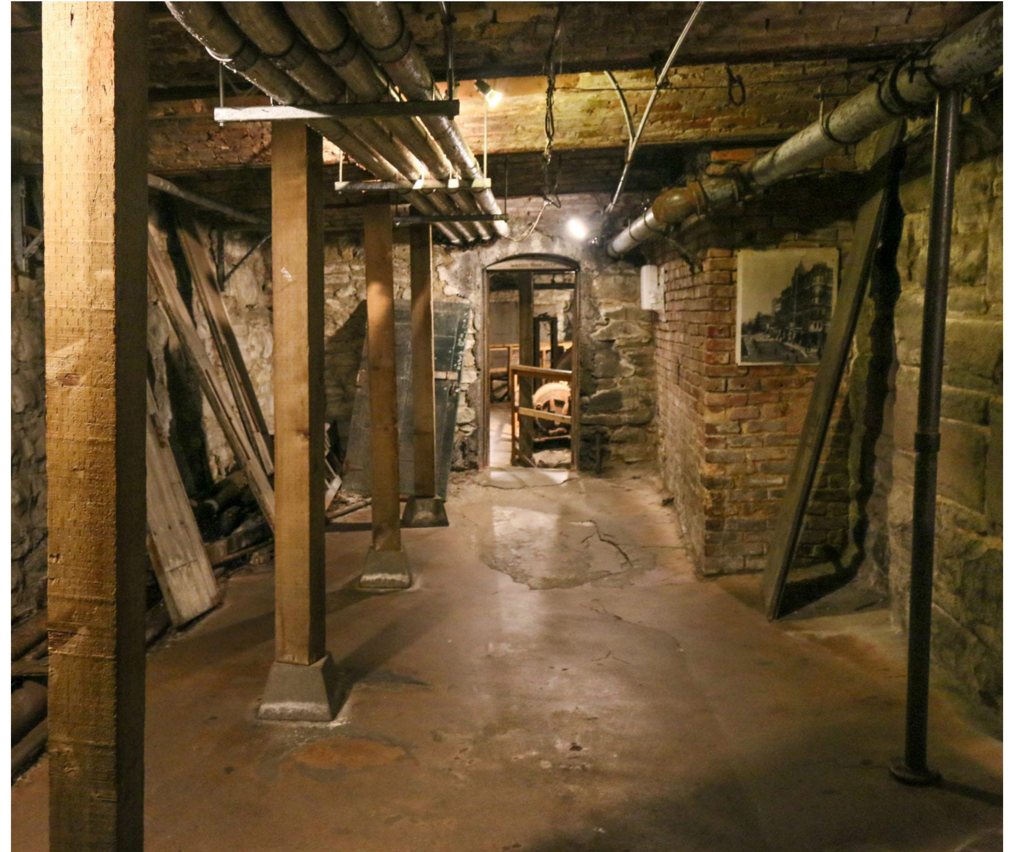
Example of an areaway. Photo source: SDOT
