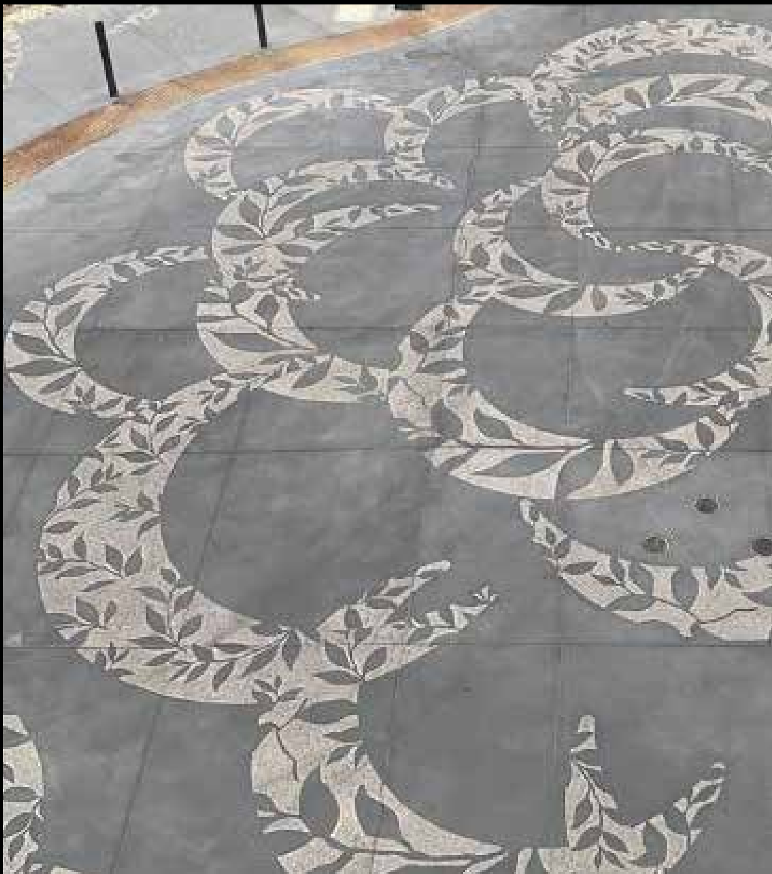
CONCRETE PLAZA WITH SANBLAST FINISH
