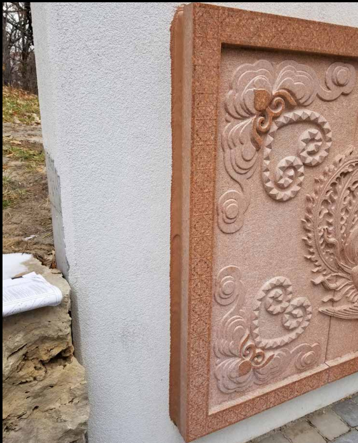
CONCRETE WALL WITH STUCCO FINISH
