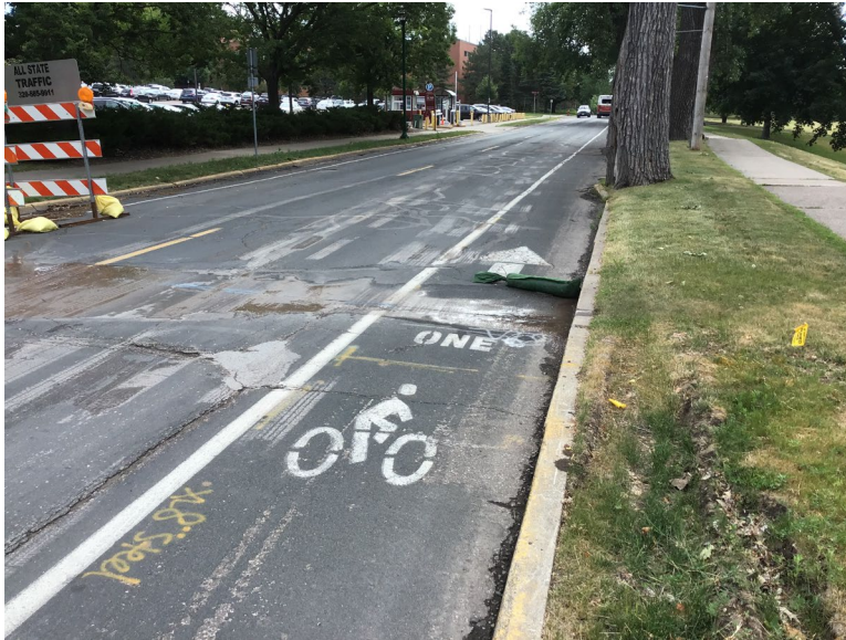
Inlet protection in place
