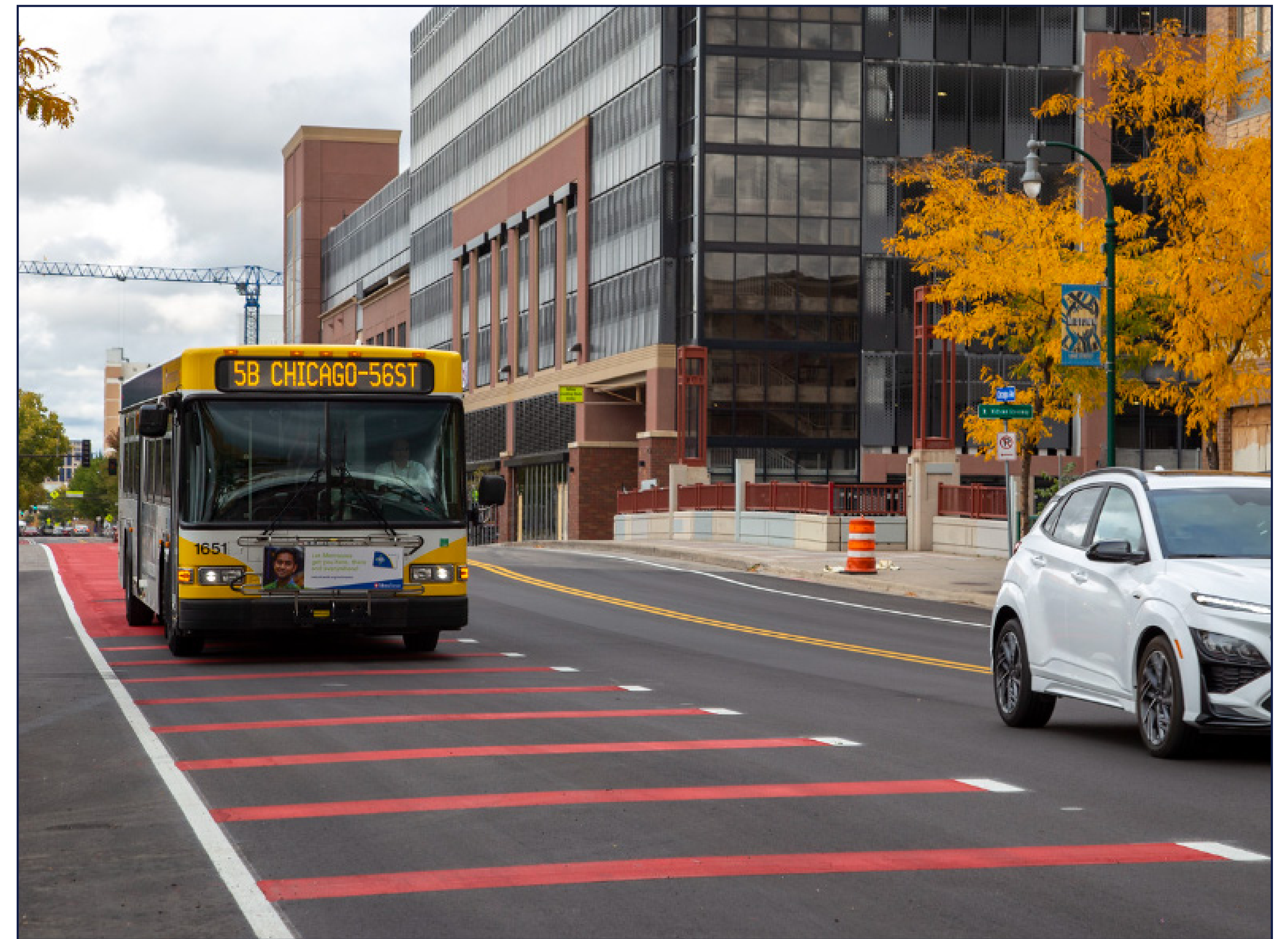
Example of one directional bus lane in Minneapolis.
