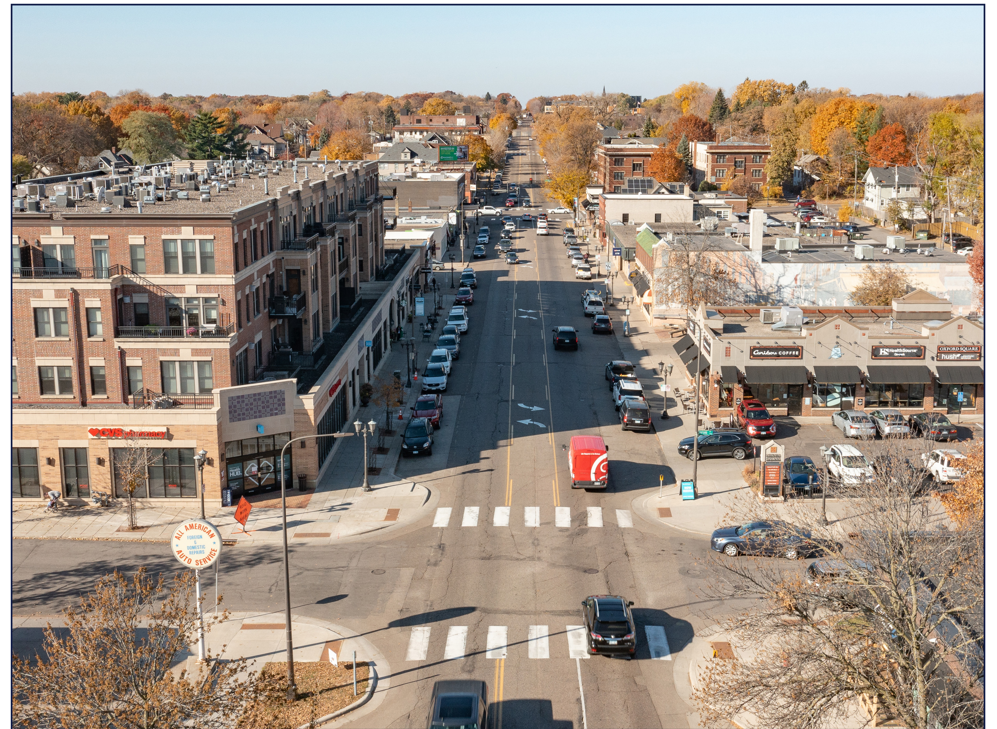
Example of two vehicle lanes with a center turn lane in Saint Paul.
