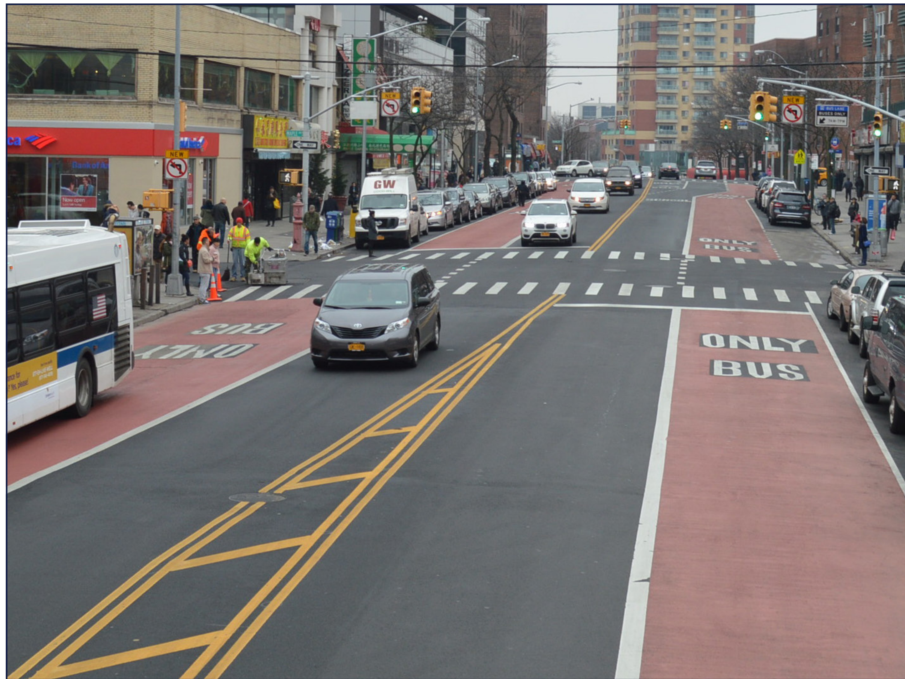
Example of two transit lanes and two vehicle lanes in New York City.
