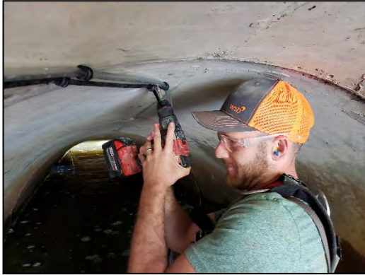
Photo 2-3: Flow Monitoring Module Install Process
