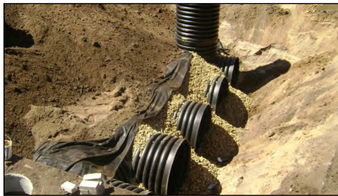
Photo 5-1: St. Albans 48" Perforated HDPE Installation
