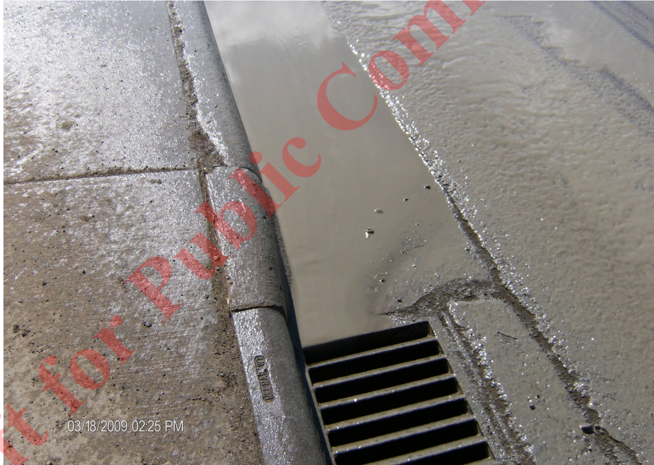
Discharge of Drilling Mud
