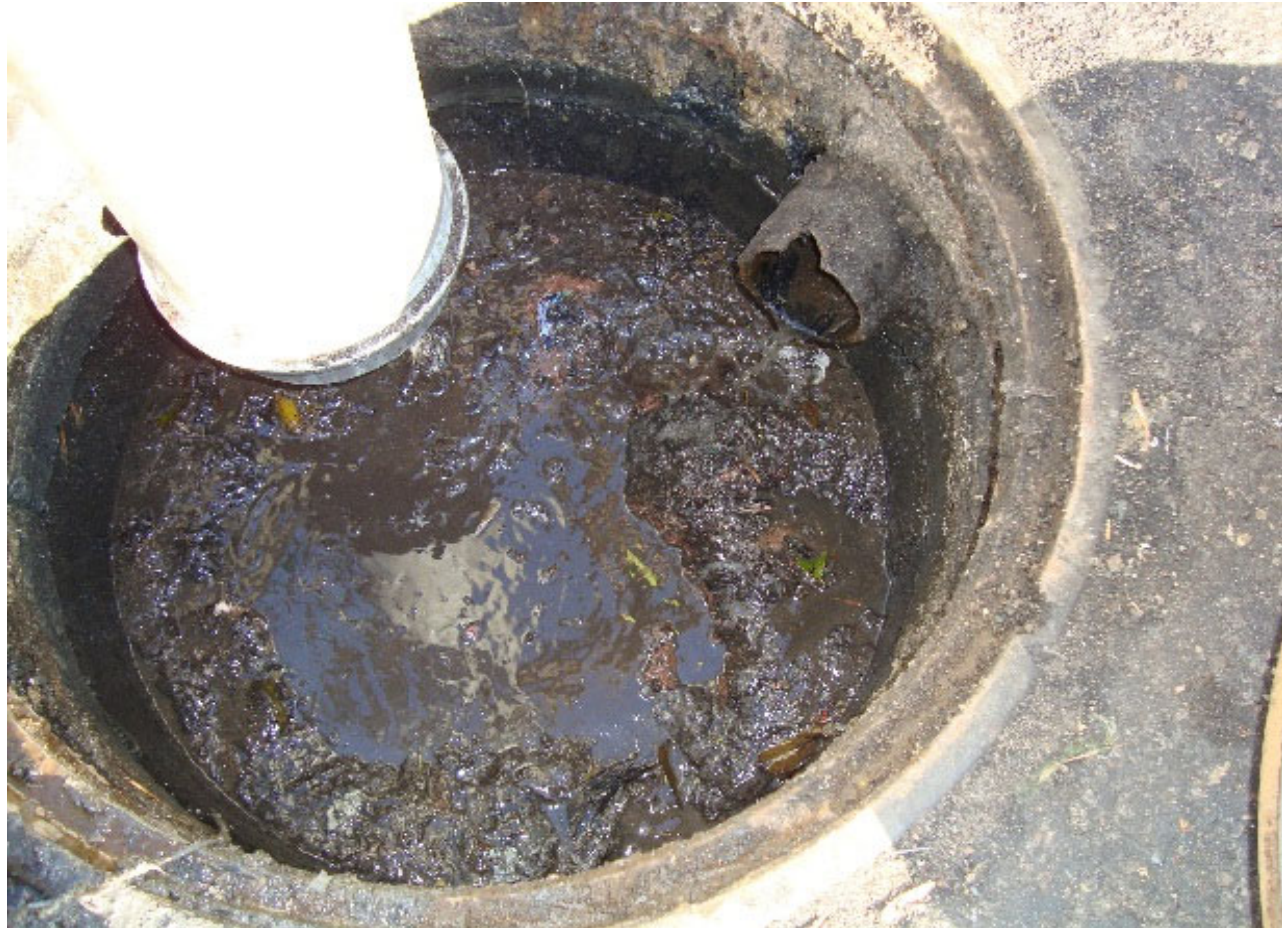
Sanitary Discharge, Private Storm Drain
