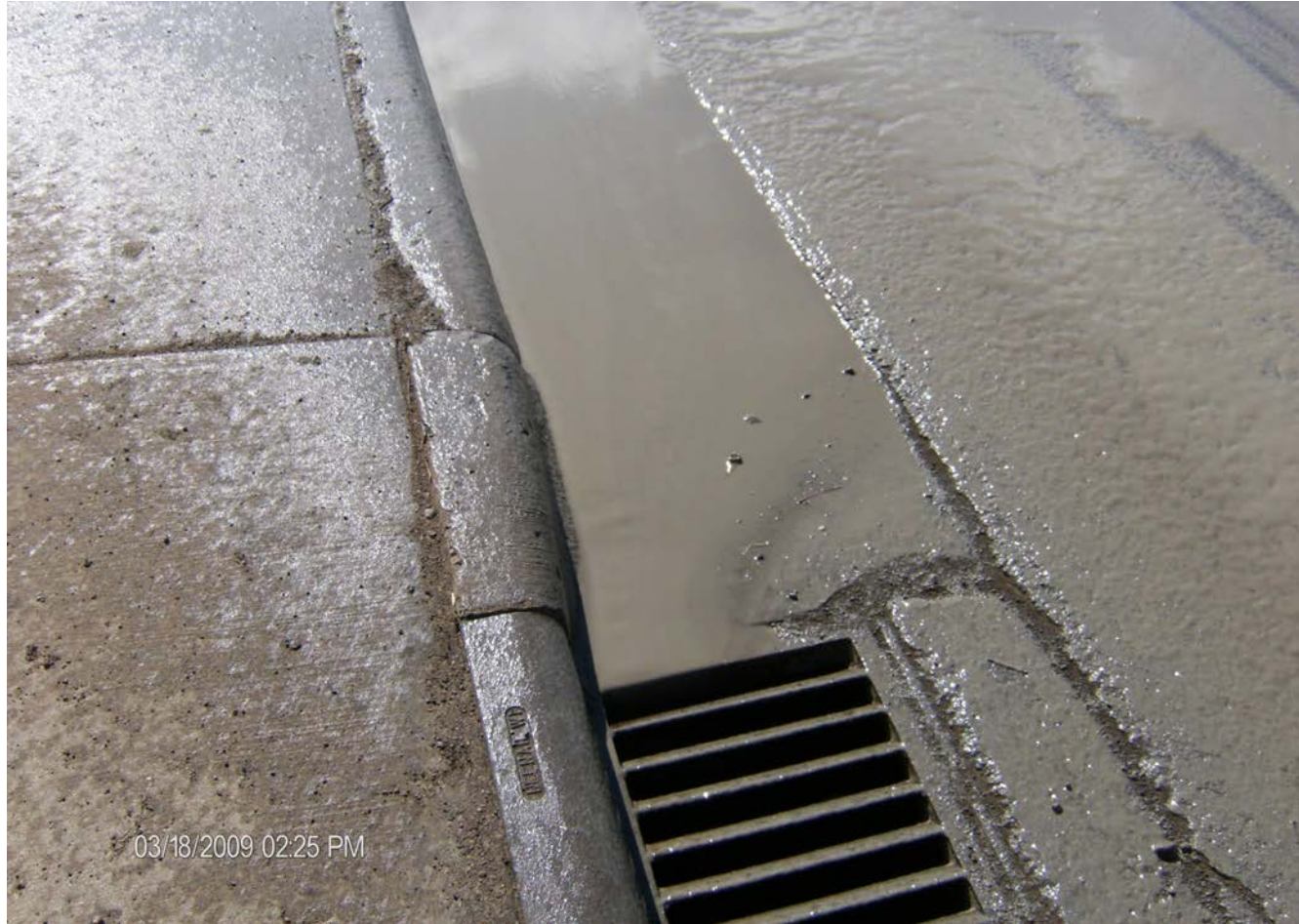
Discharge of Drilling Mud
