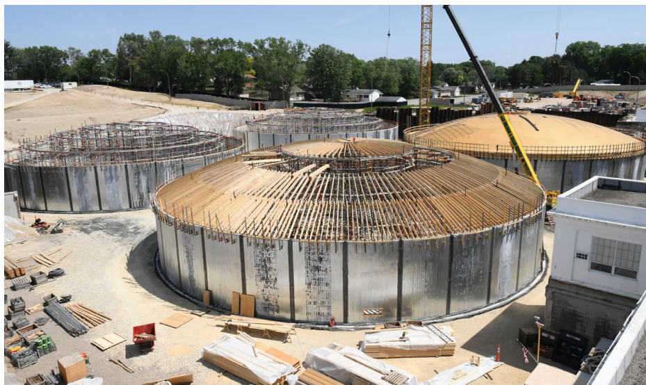
The side panels have been installed on four new clarifiers with the forms for the clarifier domes being built as of June 6. The southeastern most dome was scheduled for a concrete pour on June 8. The new facility will have four clarifiers.
