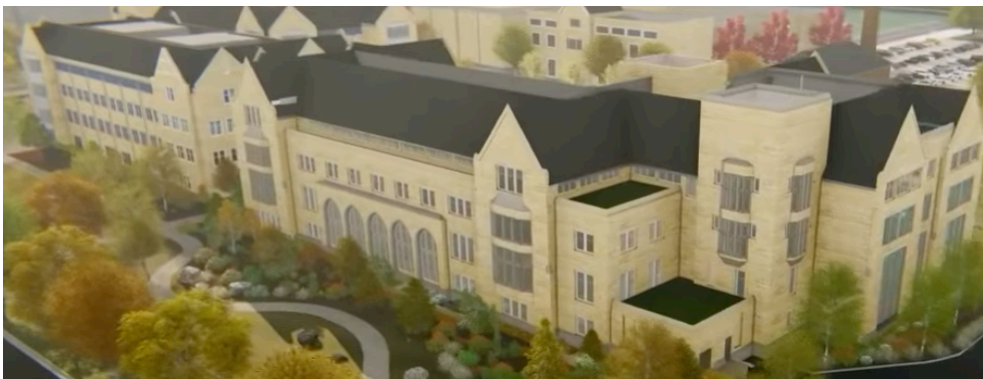
Fig. 2: O'Shaughnessy Science Hall and Schoenecker Hall
