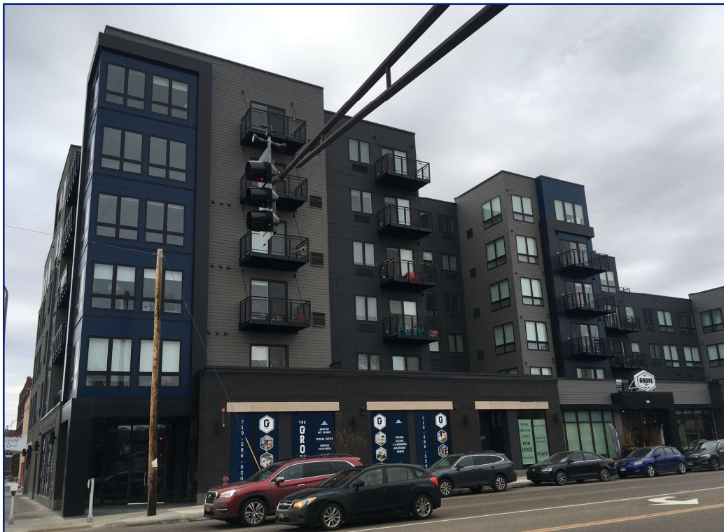
The Grove on Snelling Avenue, looking east
