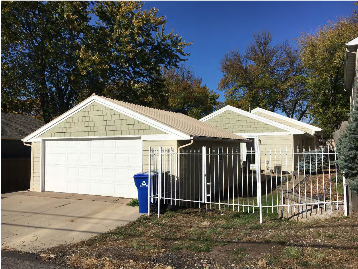
Garage at RA-SPC-11318, October 2021, south elevation, looking northwest.
