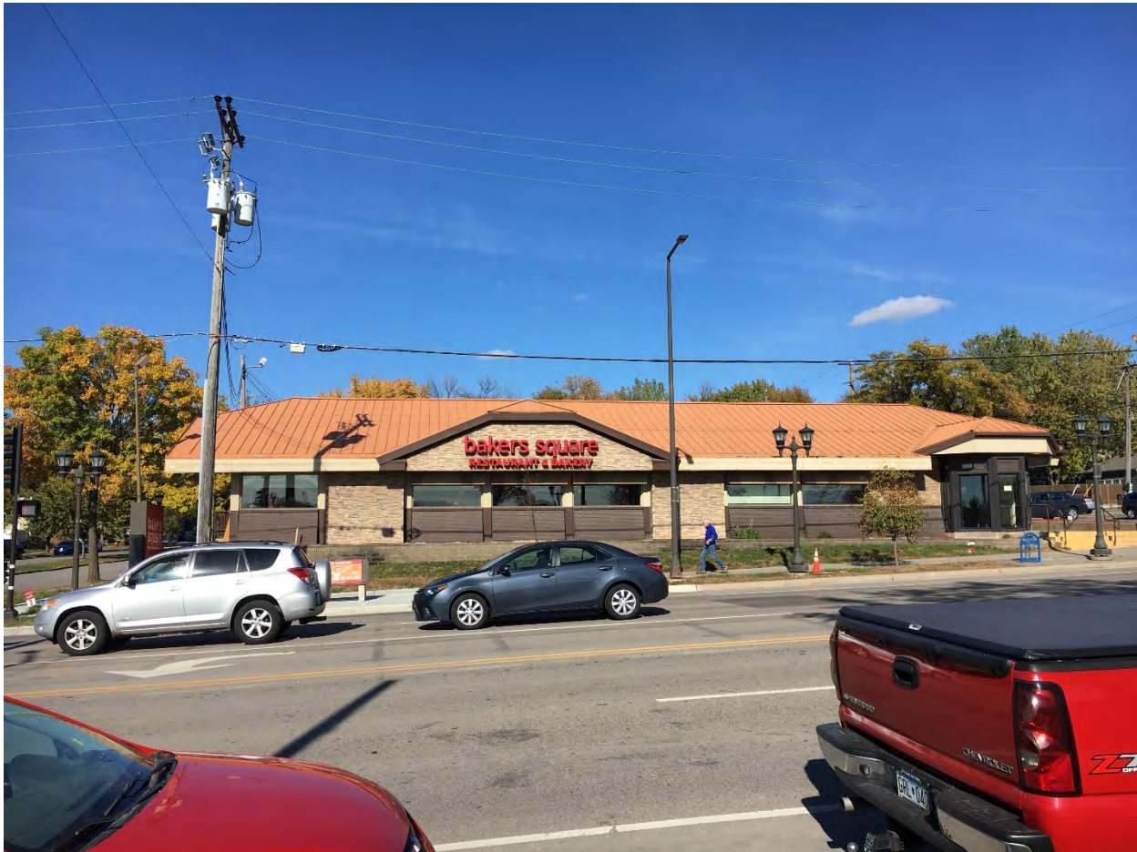
RA-SPC-11314, October 2021, south elevation, looking north.
