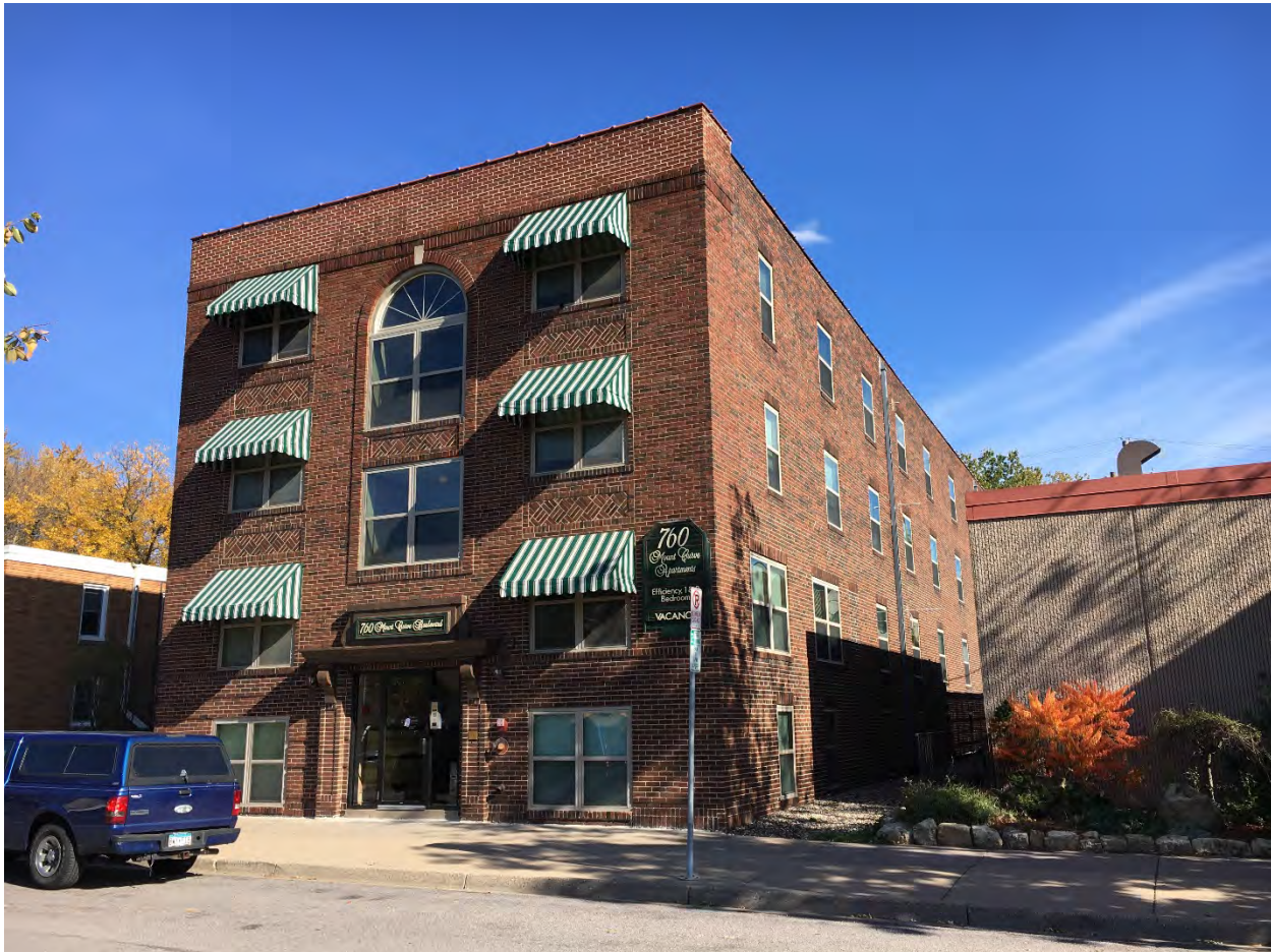
RA-SPC-11315, October 2021, south and west elevations, looking northeast.
