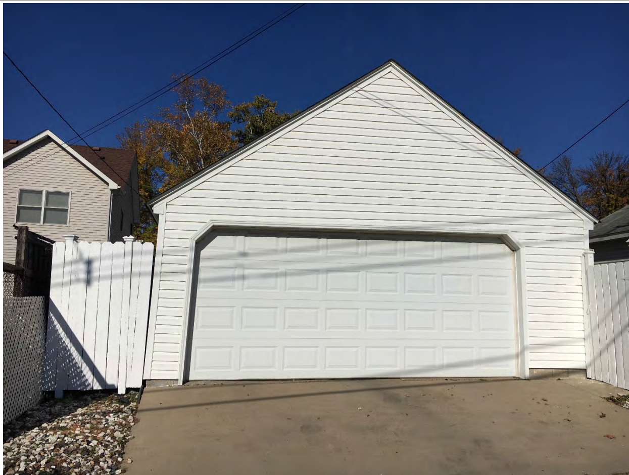
Garage at RA-SPC-11319, October 2021, south elevation, looking north.
