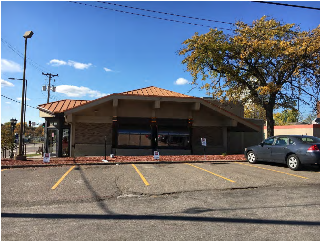
RA-SPC-11314, October 2021, east elevation, looking west.
