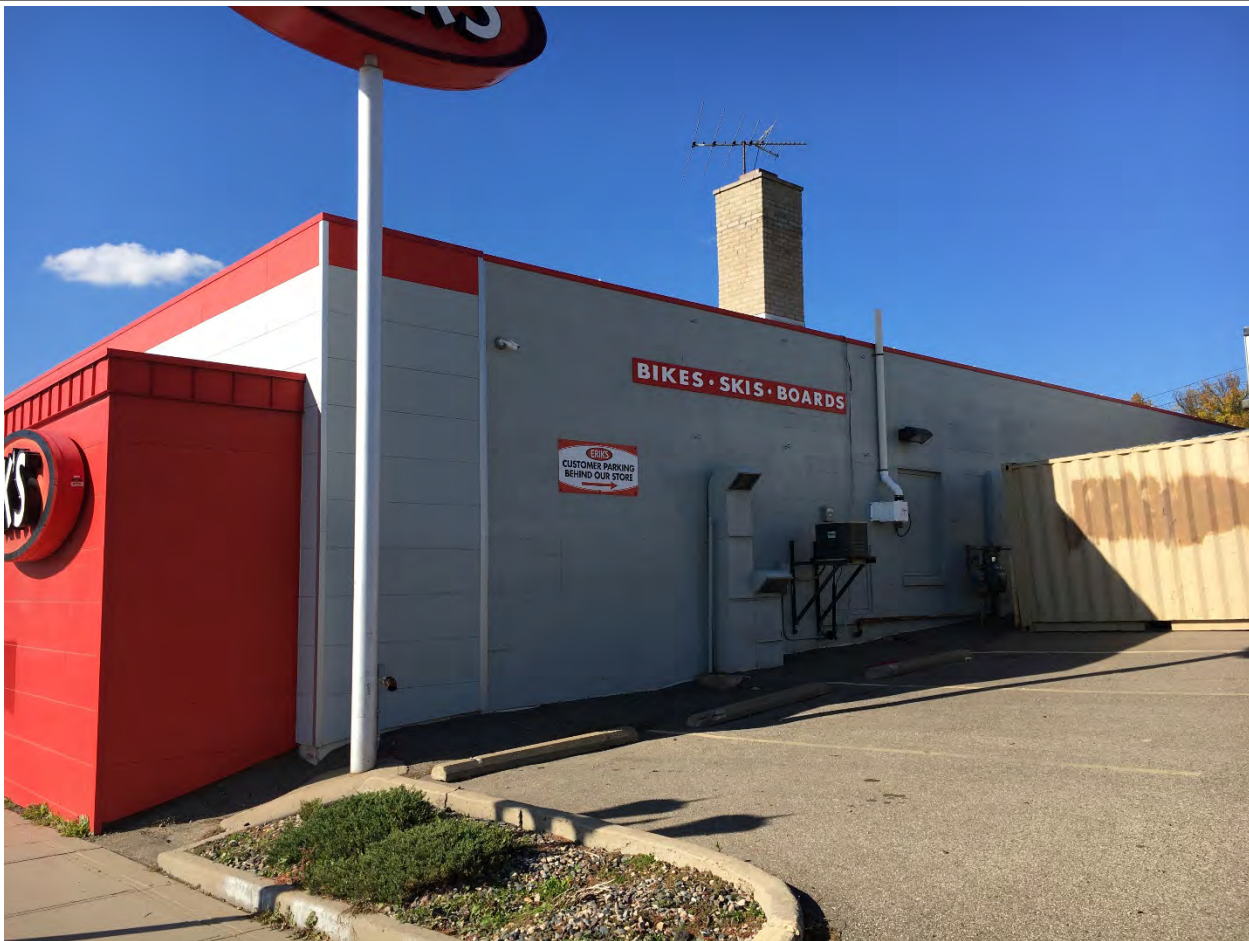
RA-SPC-11322, October 2021, east elevation, looking northwest.
