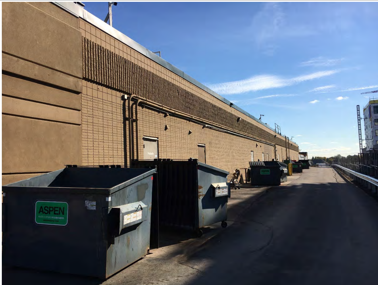
RA-SPC-11324, October 2021, west elevation, looking southeast.
