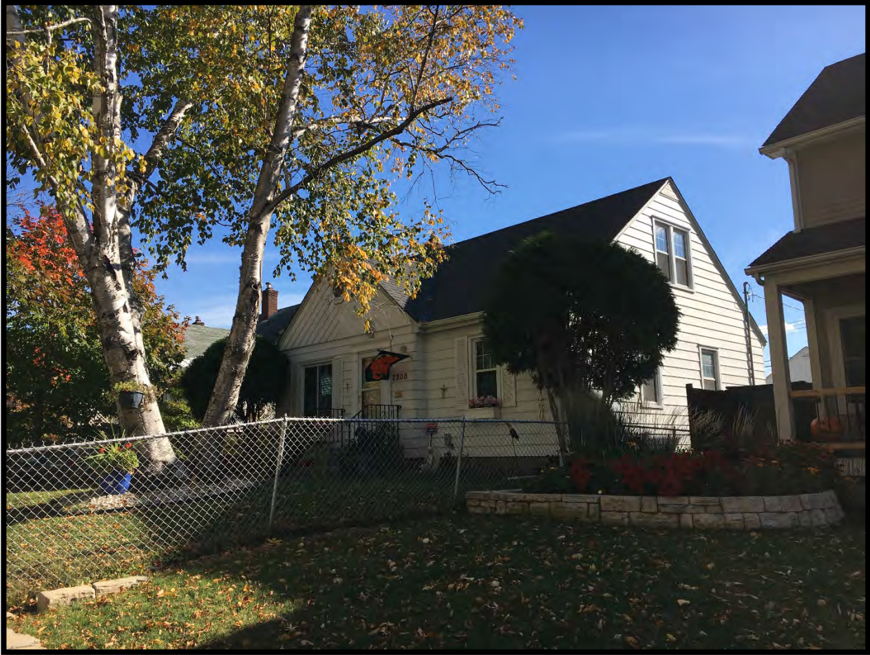
RA-SPC-11319, October 2021, north and west elevations, looking southeast.
