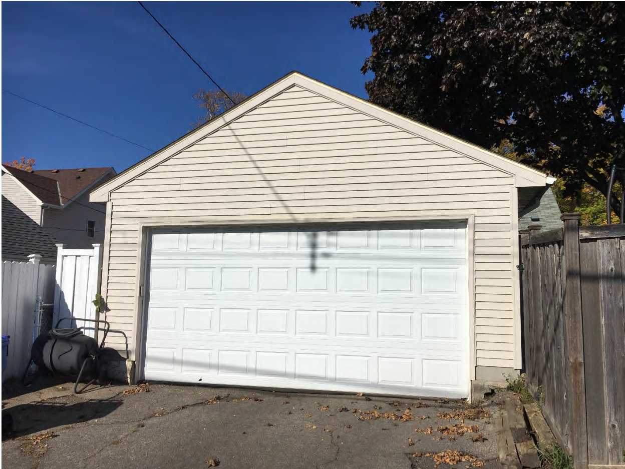
Garage at RA-SPC-11320, October 2021, south elevation, looking north.
