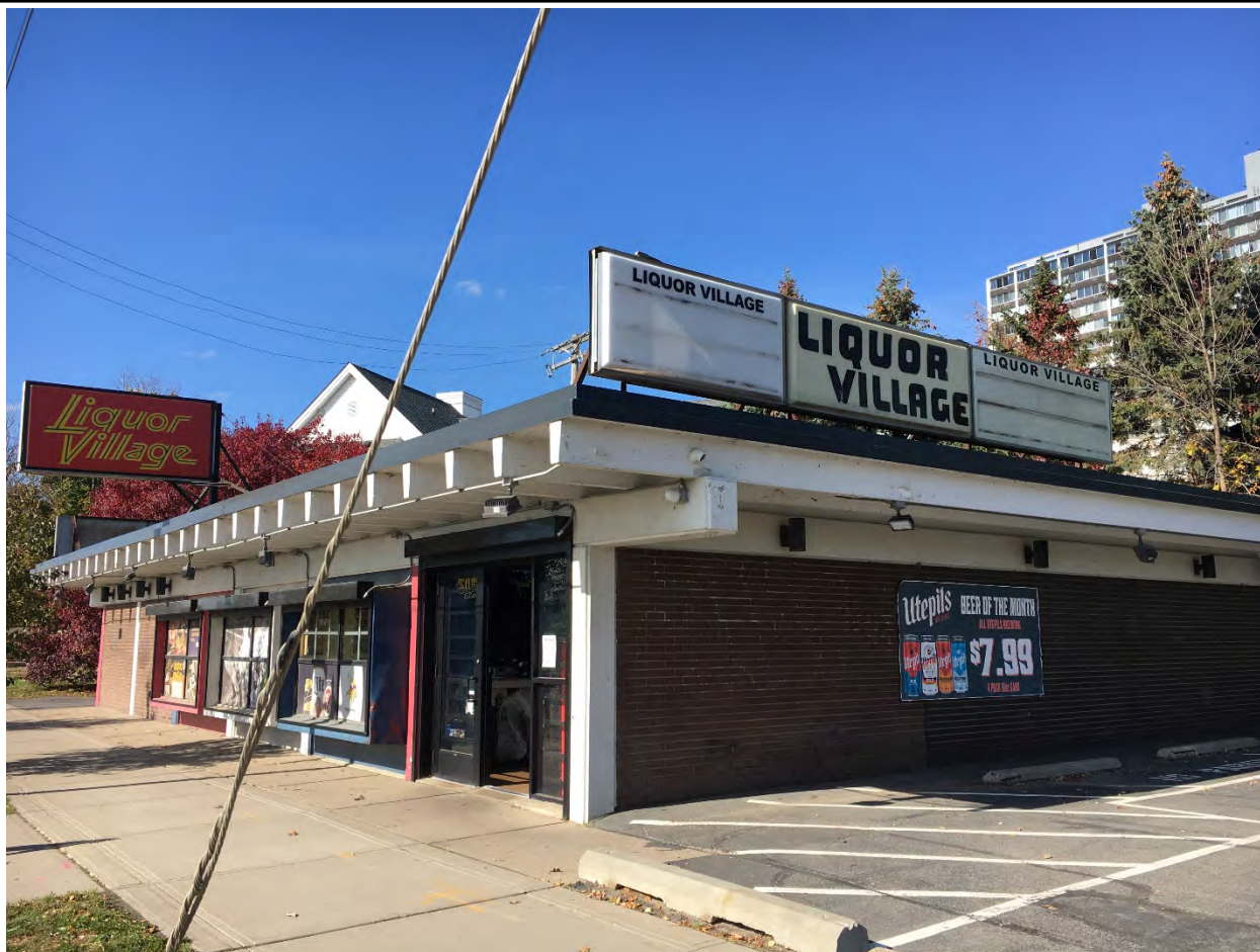
RA-SPC-11312, October 2021, east and south elevations, looking northwest.
