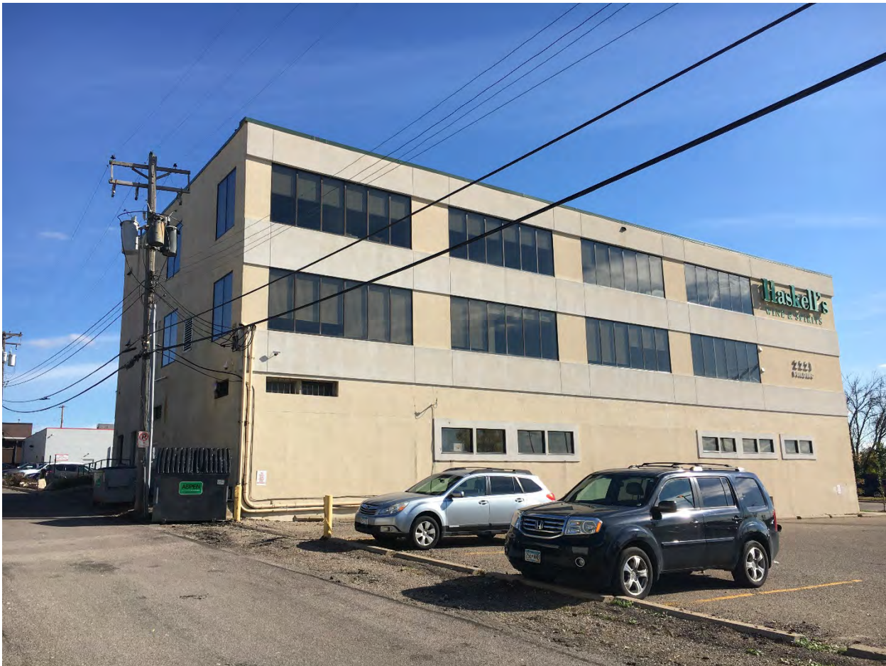
RA-SPC-11321, October 2021, north and west elevations, looking southeast.
