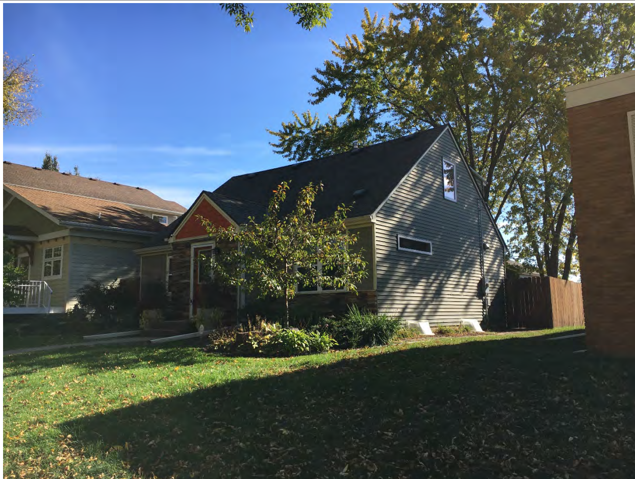
RA-SPC-11317, October 2021, west and north elevations, looking southeast.
