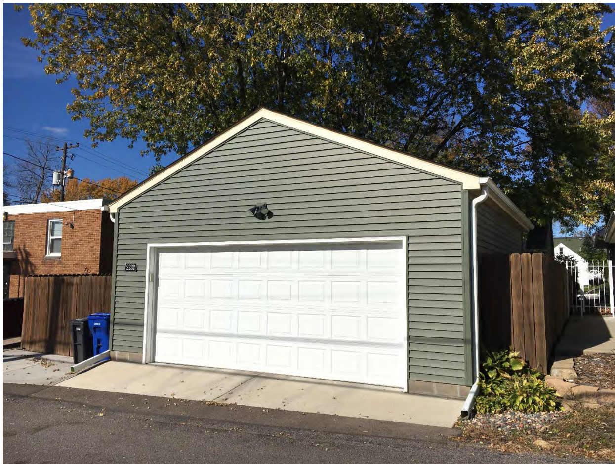
Garage at RA-SPC-11317, October 2021, south elevation, looking northwest.
