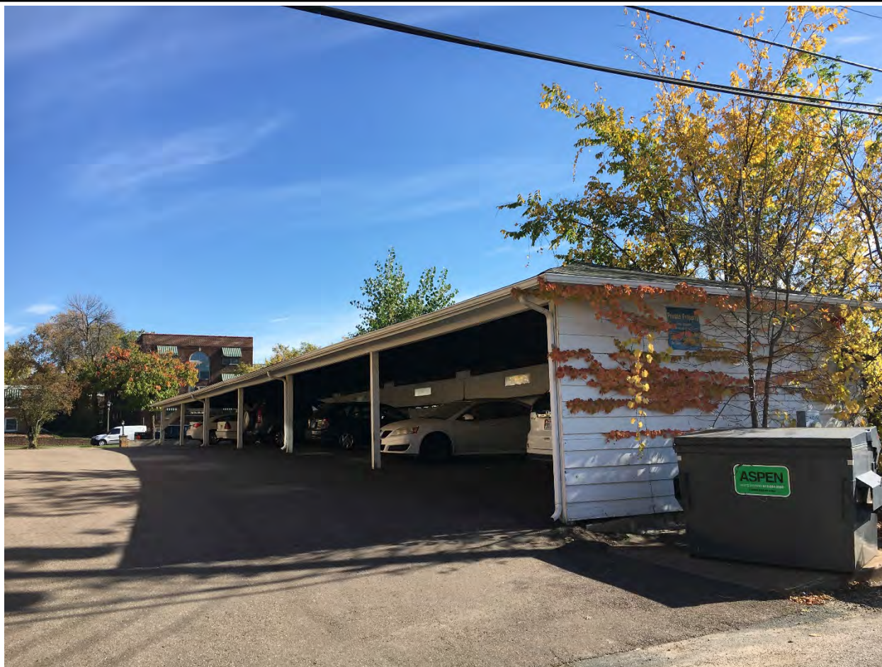
Carport at RA-SPC-11313, October 2021, west and north elevations, looking southeast.
