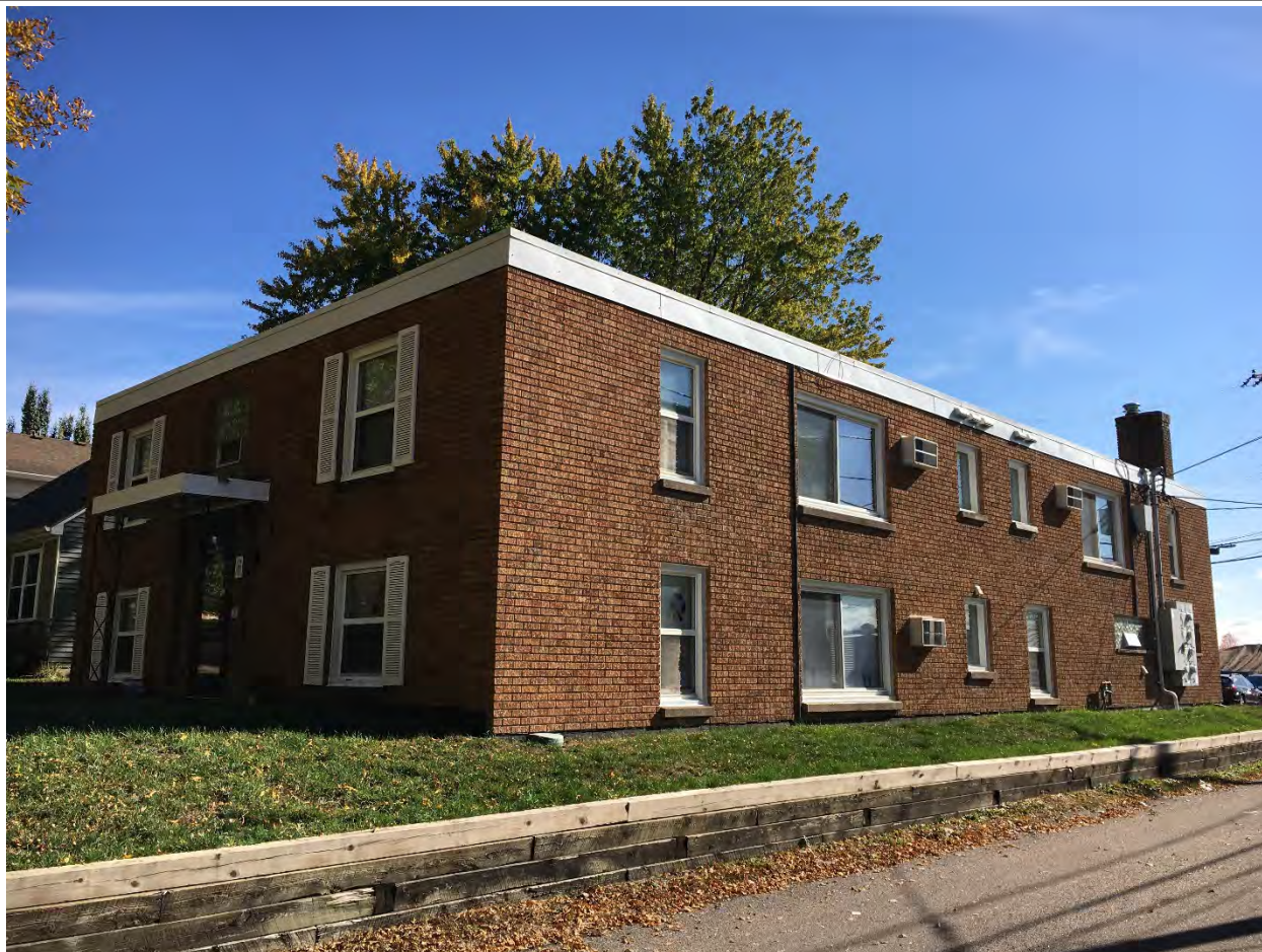
RA-SPC-11316, October 2021, north and west elevations, looking southeast.
