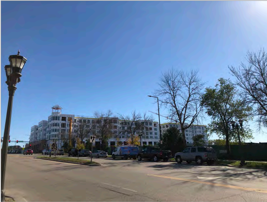
Figure 2. Looking Southeast from W. Ford Parkway towards Parcel A, with new housing development in the foreground.
