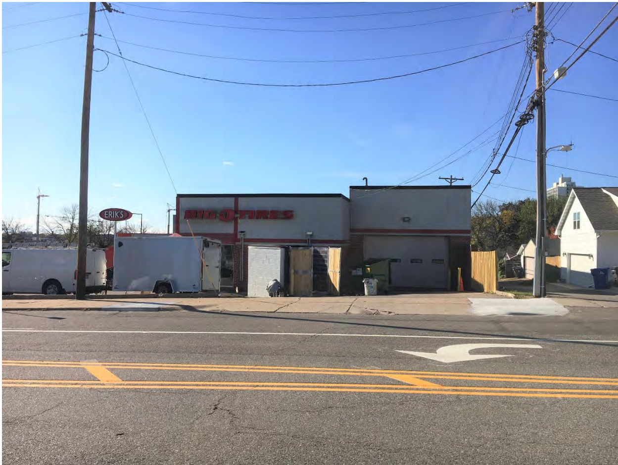
RA-SPC-11323, October 2021, east elevation, looking west.
