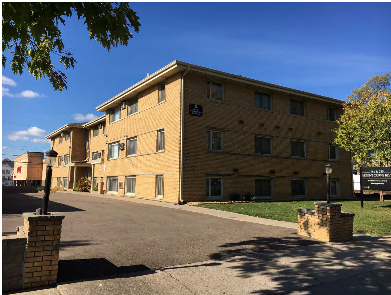
RA-SPC-11313, October 2021, south and east elevations, looking northwest.
