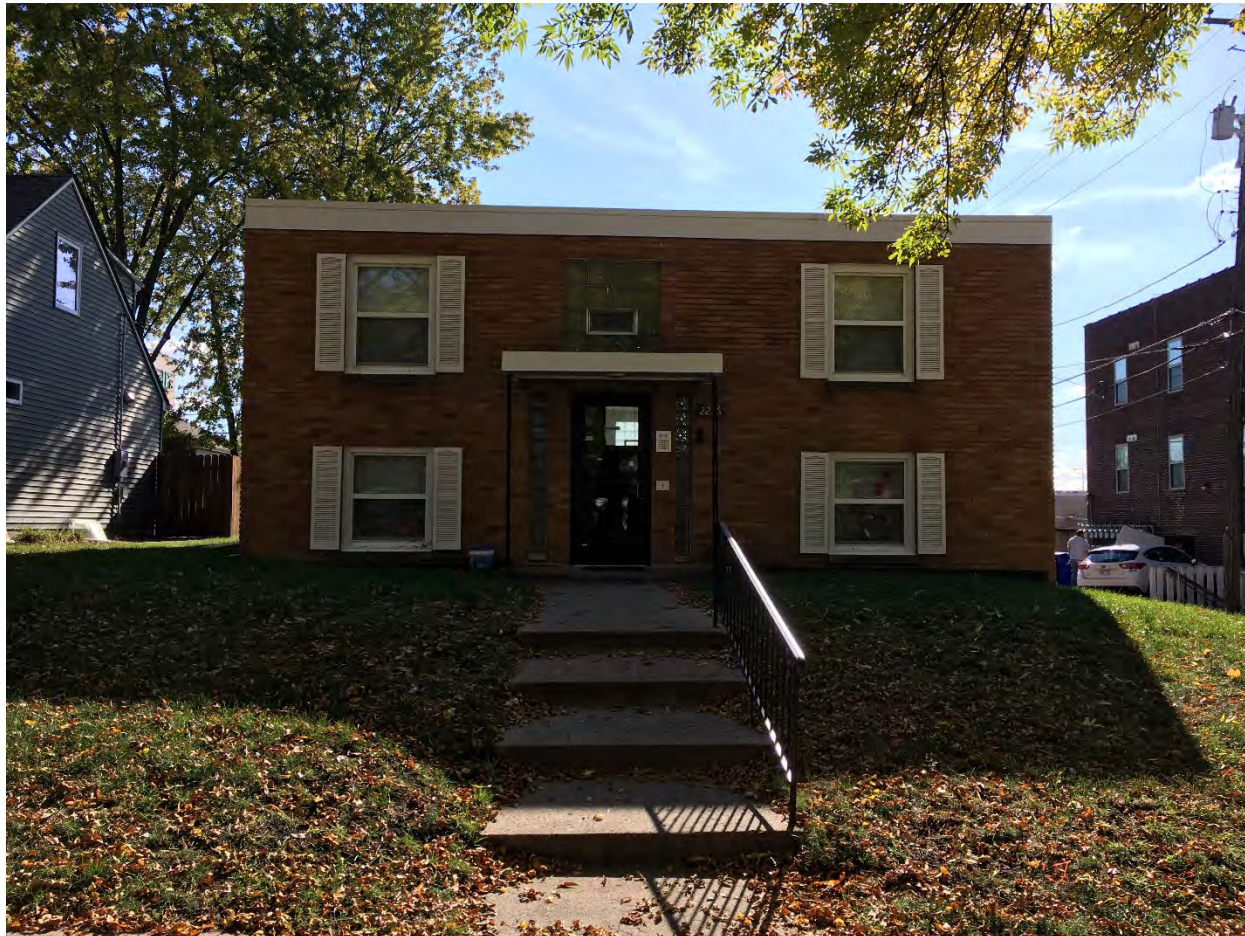
RA-SPC-11316, October 2021, north elevation, looking south.
