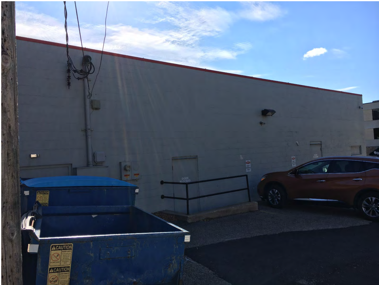
RA-SPC-11322, October 2021, north elevation, looking southwest.
