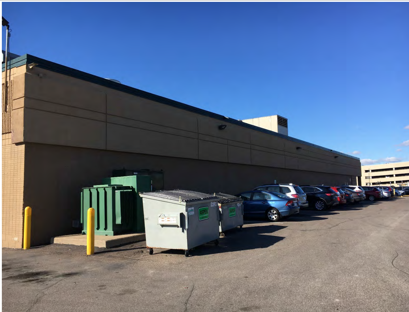
RA-SPC-11324, October 2021, east elevation, looking northwest.
