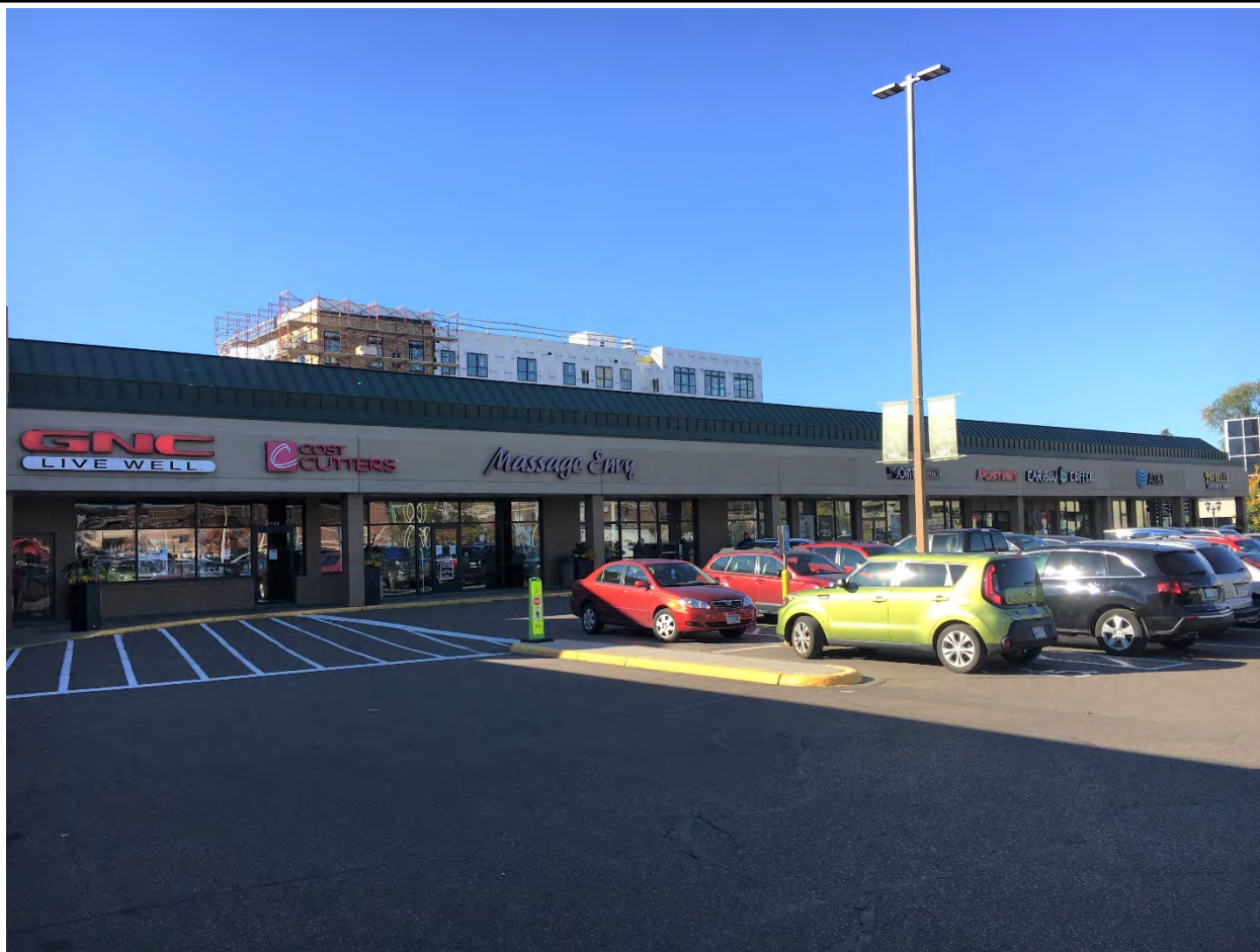
RA-SPC-11324, October 2021, east elevation, looking northwest.
