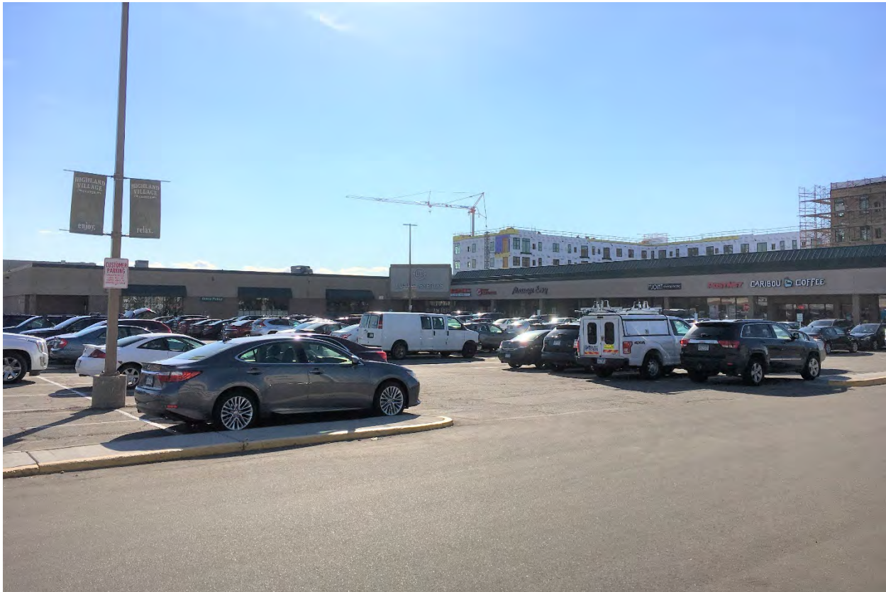
RA-SPC-11324, October 2021, east and north elevations, looking southwest.
