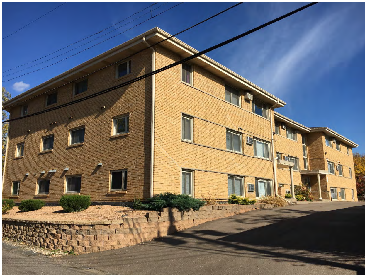
RA-SPC-11313, October 2021, south and west elevations, looking northeast.
