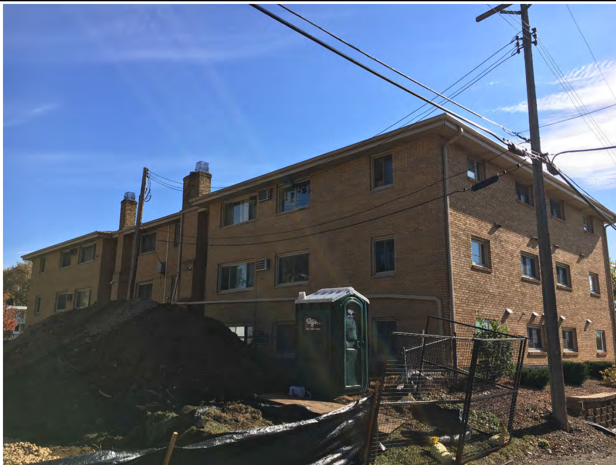
RA-SPC-11313, October 2021, north and west elevations, looking southeast.
