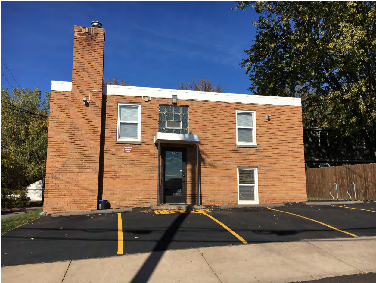
RA-SPC-11316, October 2021, south elevation, looking north.
