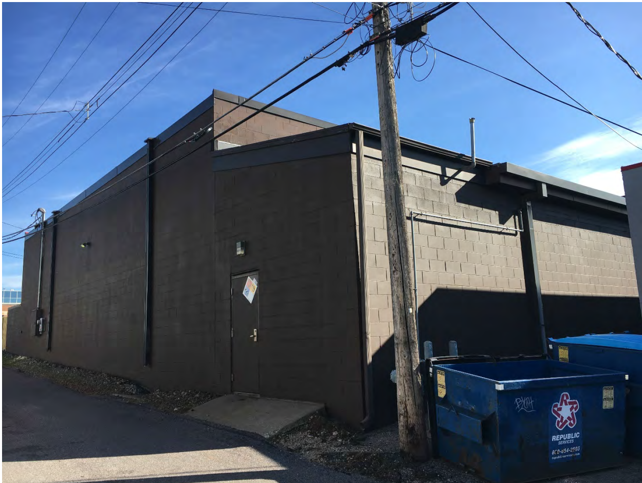
RA-SPC-11323, October 2021, north and west elevations, looking southeast.
