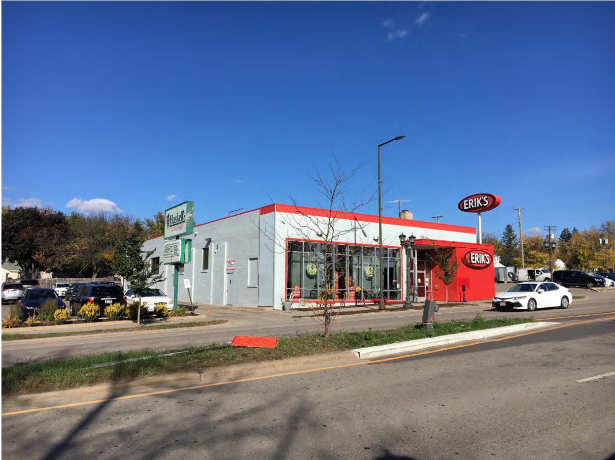
RA-SPC-11322, October 2021, south and west elevations, looking northeast.
