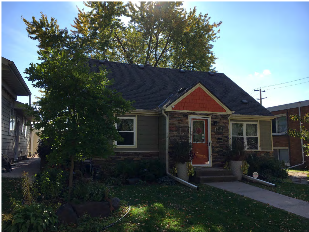
RA-SPC-11317, October 2021, north elevation, looking southwest.
