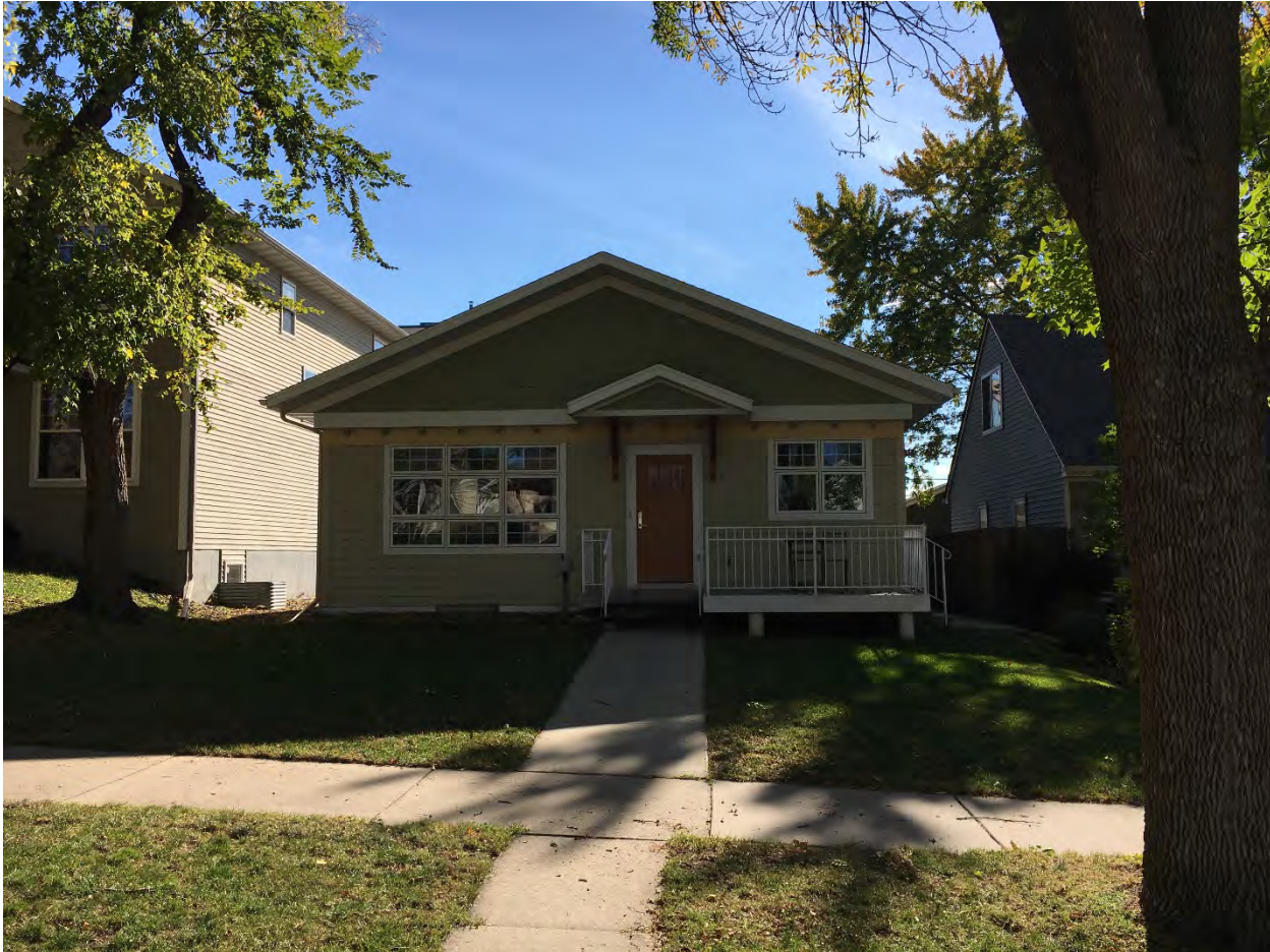
RA-SPC-11318, October 2021, north elevation, looking south.
