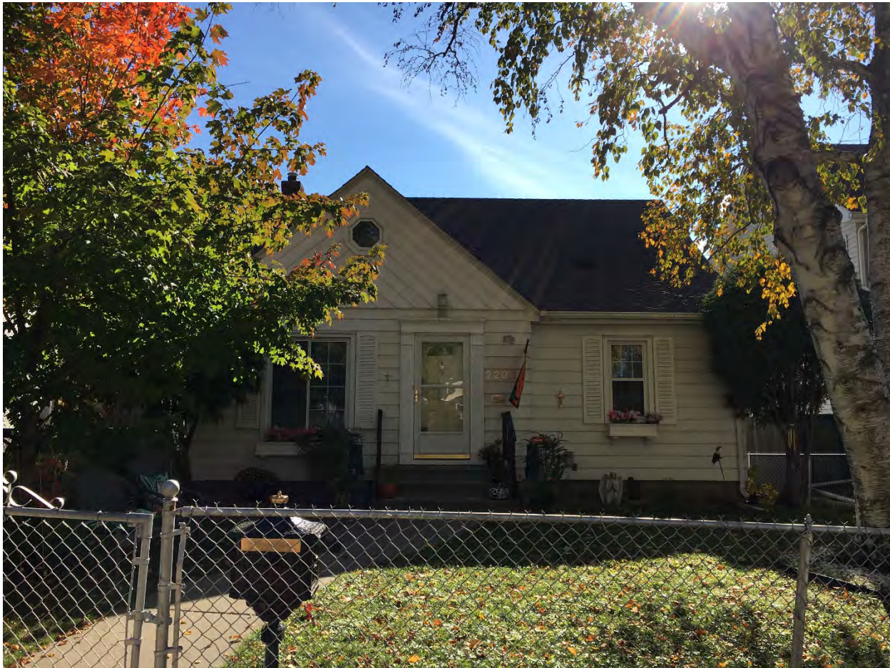
RA-SPC-11319, October 2021, north elevation, looking south.
