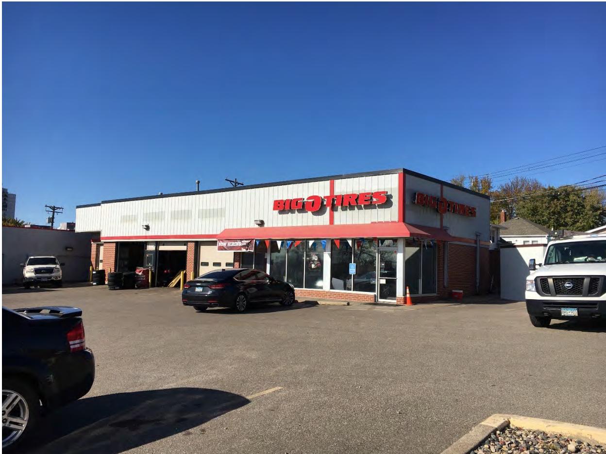
RA-SPC-11323, October 2021, east and south elevations, looking northwest.
