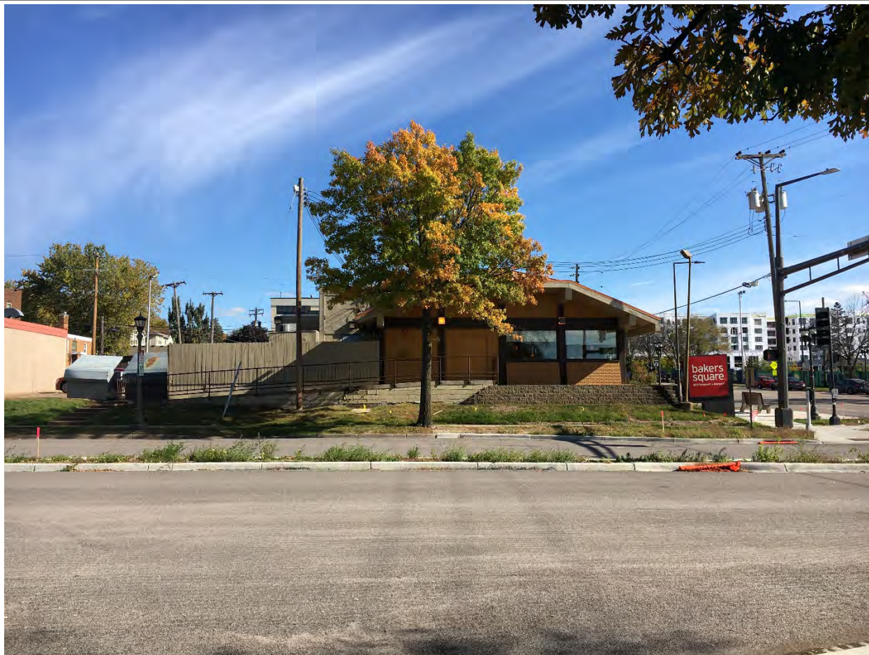
RA-SPC-11314, October 2021, west elevation, looking east.
