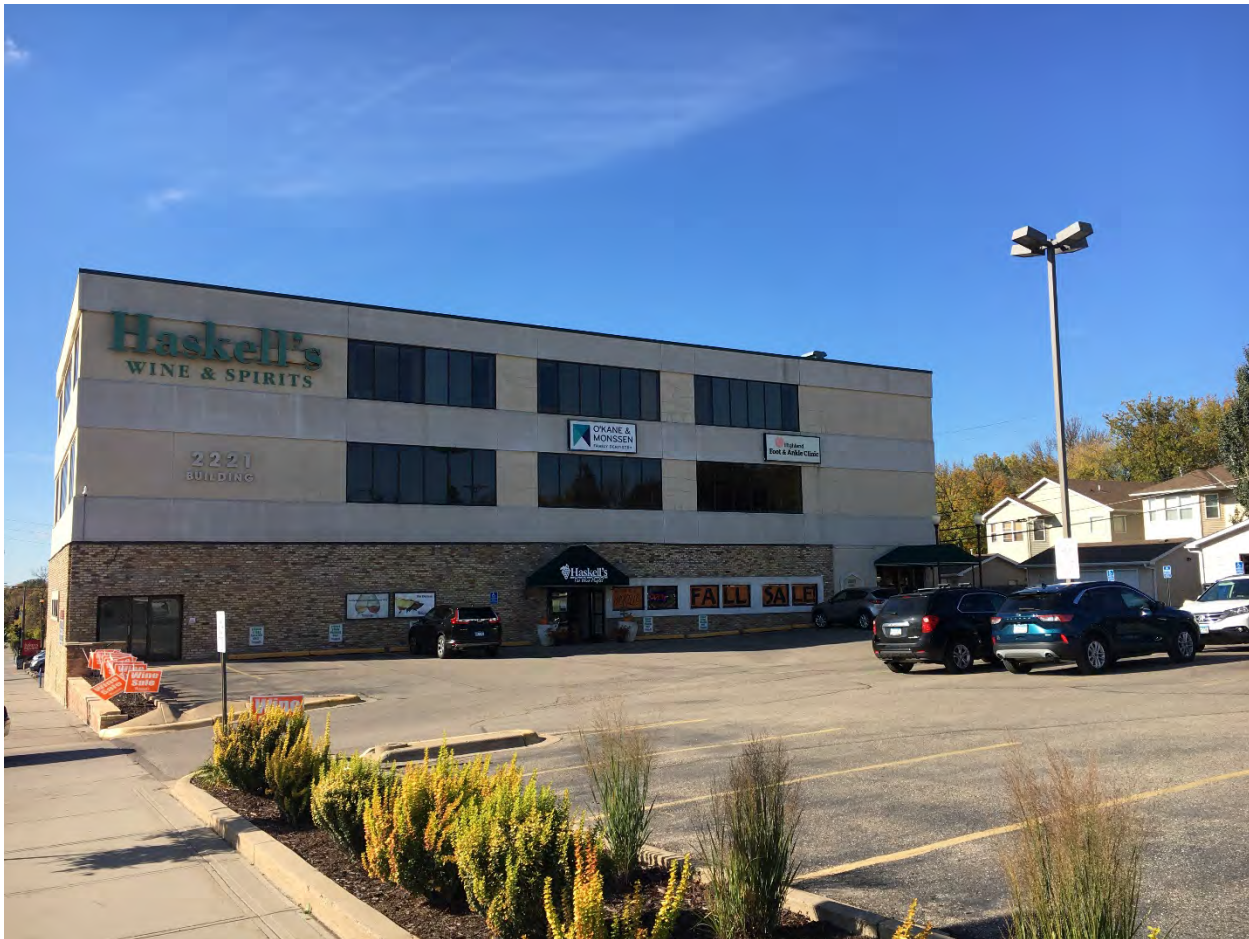
RA-SPC-11321, October 2021, east elevation, looking west.
