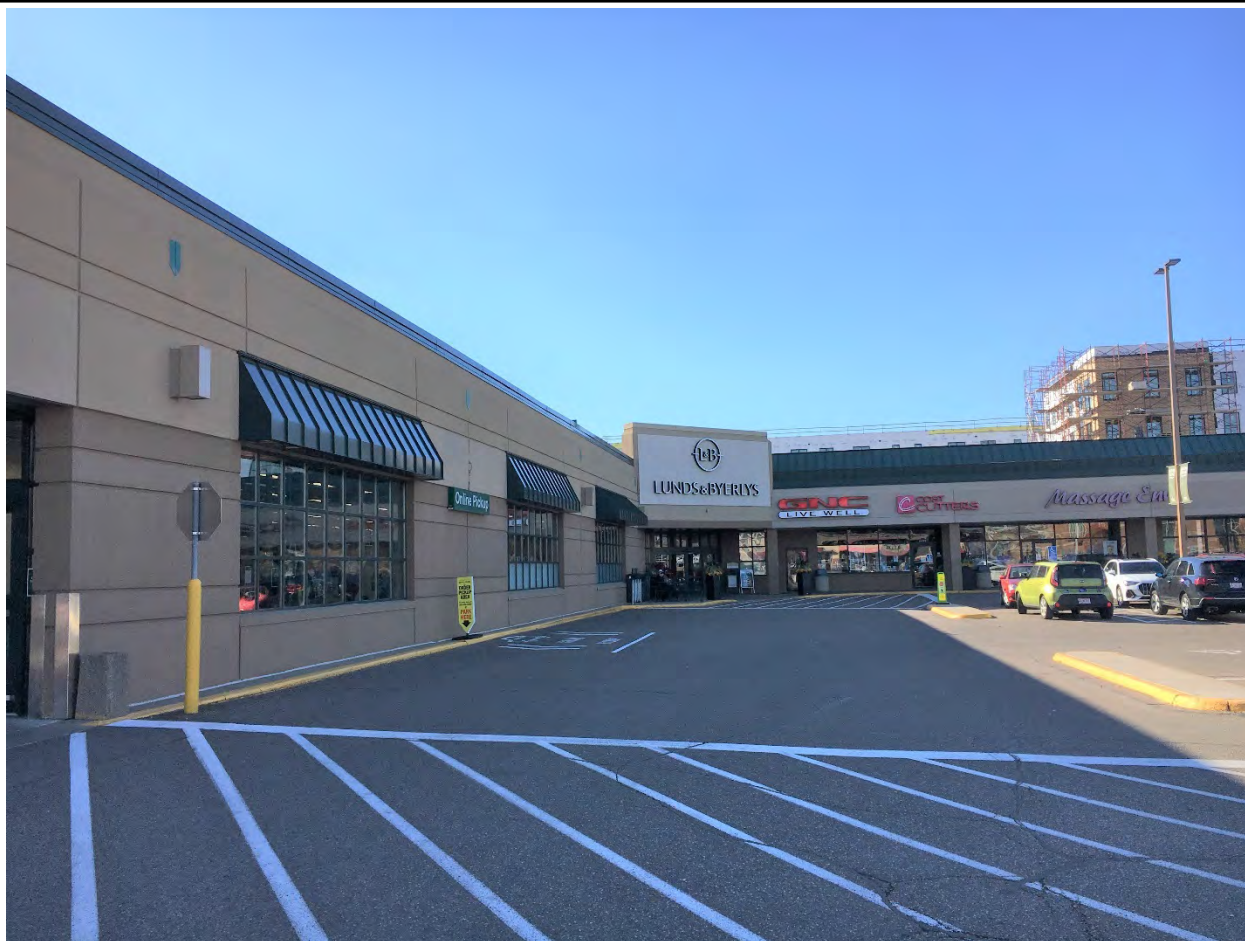
RA-SPC-11324, October 2021, north and east elevations, looking southwest.
