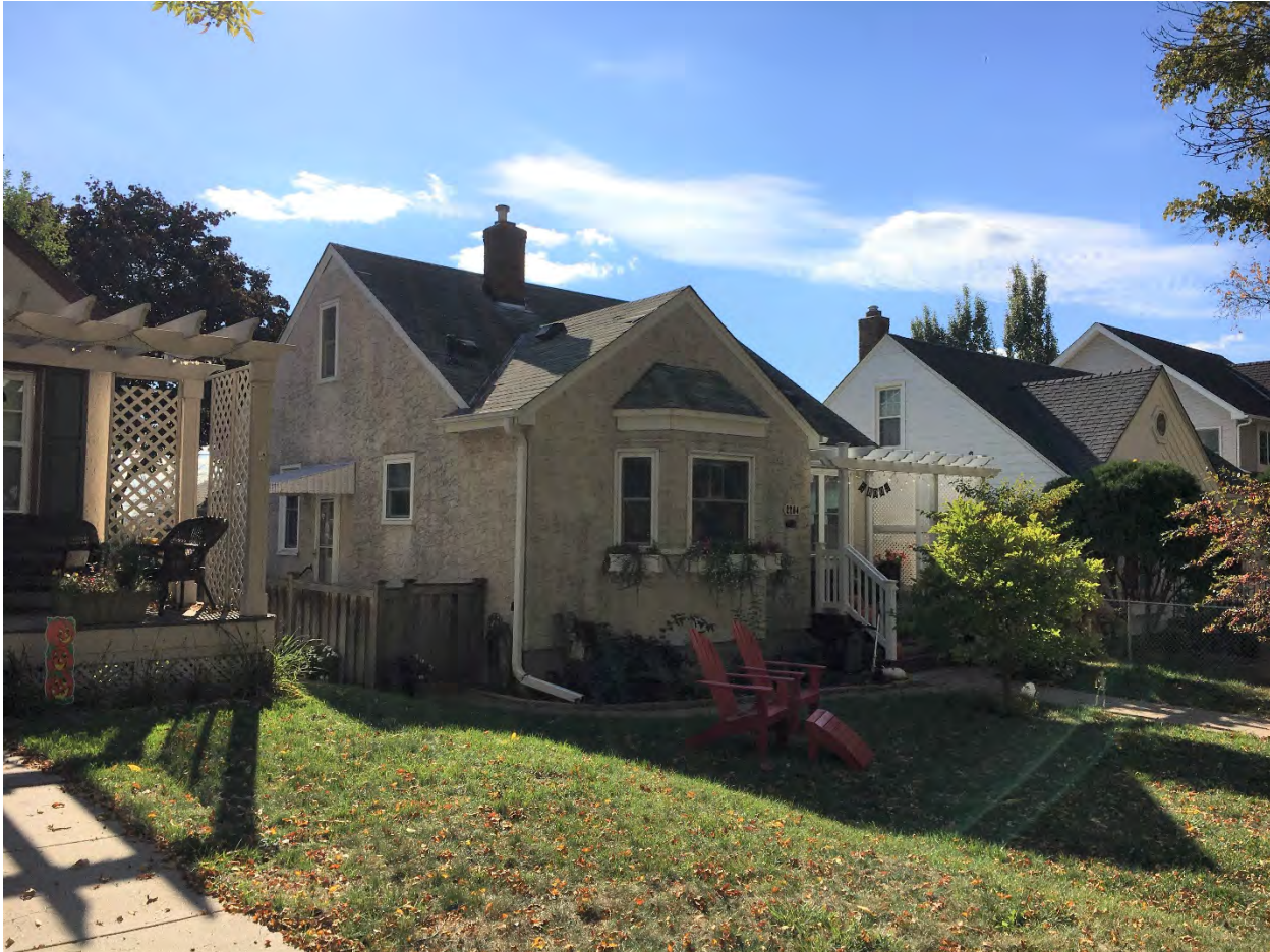
RA-SPC-11320, October 2021, north and east elevations, looking southwest.
