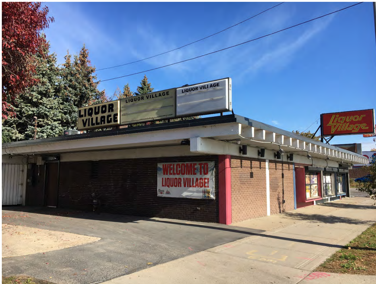
RA-SPC-11312, October 2021, west and south elevations, looking northeast.
