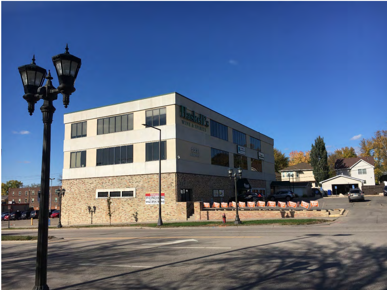
RA-SPC-11321, October 2021, south and east elevations, looking northwest.
