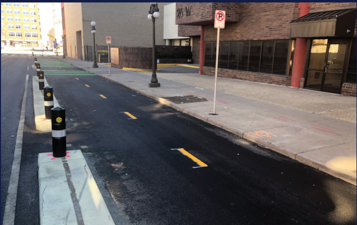
▲ 10th St downtown: Form-in-place curbs, bollards
