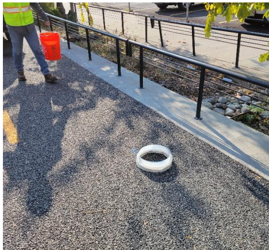
Photo 2-7: Permeable Pavement Infiltration Test
