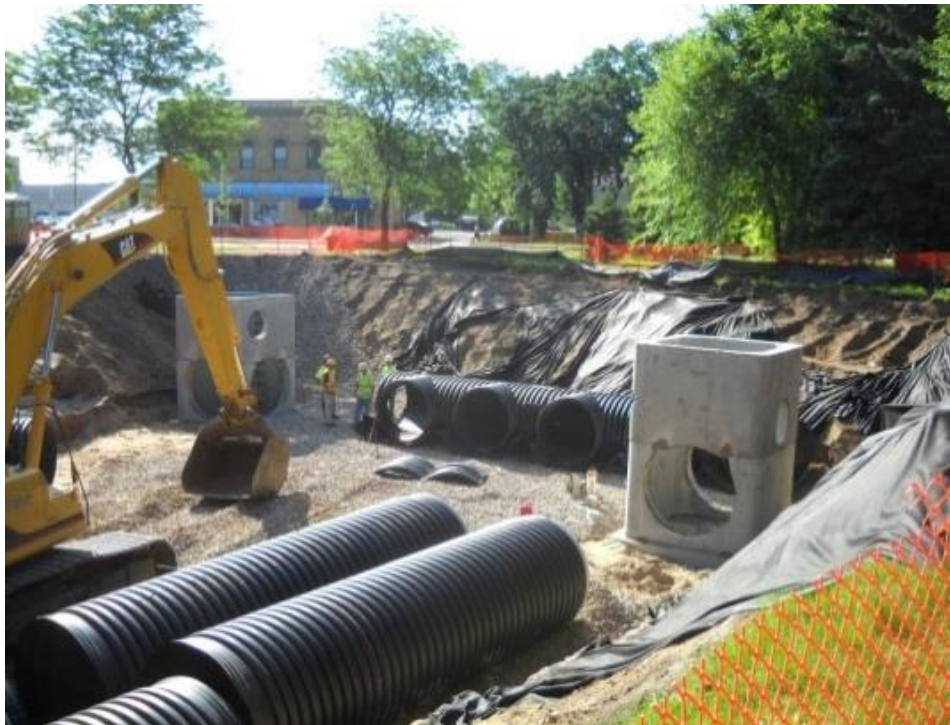
Photo 6-1: Hampden Park BMP Construction
