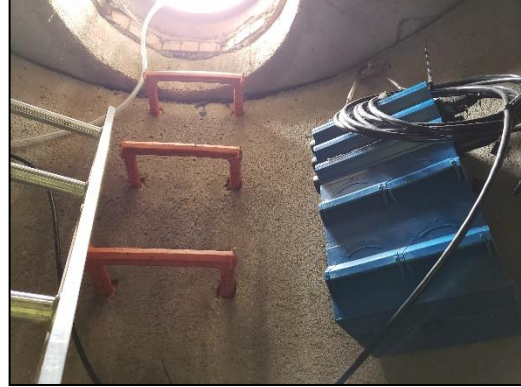
Photo 2-4: Flow Monitoring Equipment Install
