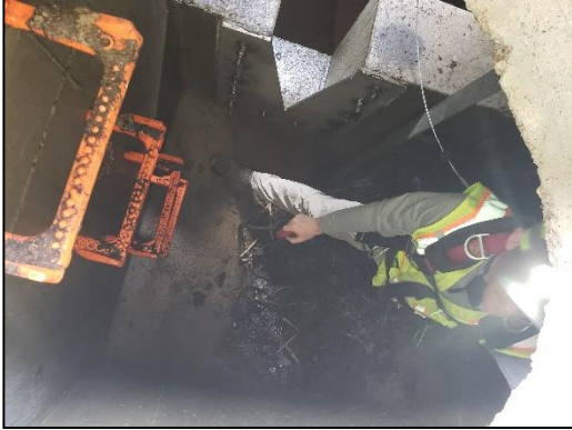
Photo 2-3: Flow Monitoring Module Install Process
