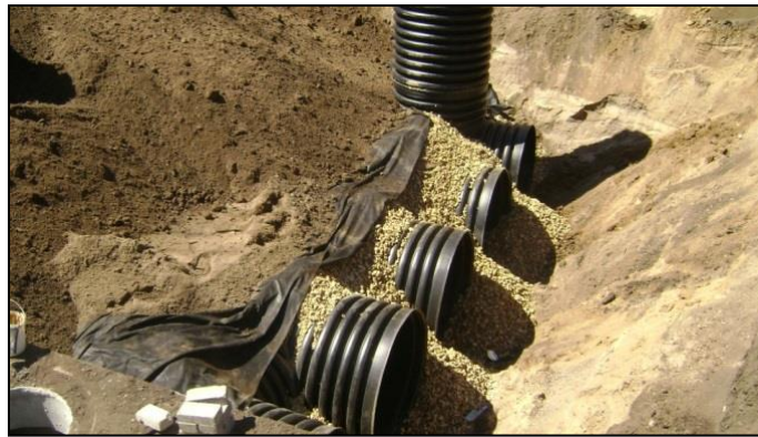
Photo 5-1: St. Albans 48” Perforated HDPE Installation
