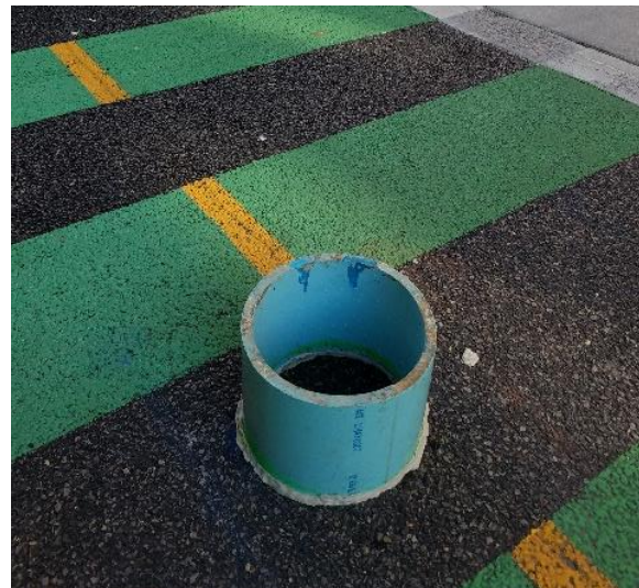
Photo 11-6: Jackson Street Infiltration Test
