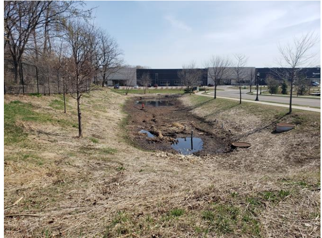
Photo 4-2: Rain Garden Located above Infiltration Chambers (Facing East)
