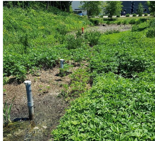
Photo 2-2: Beacon Bluff Rain Garden and In-Rock Wells
