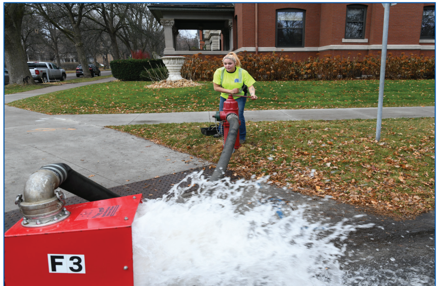
A worker flushes a water hydrant during annual testing.
