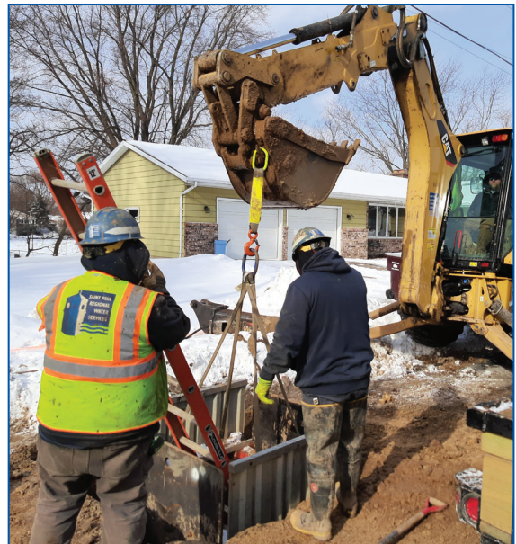
Crews prepare to replace lead water service lines.
