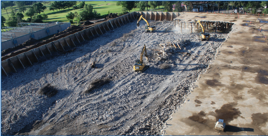
The 18-million-gallon Highland Reservoir was demolished in 2021.
