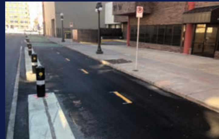
▲ 10th St downtown: Form-in-place curbs, bollards
