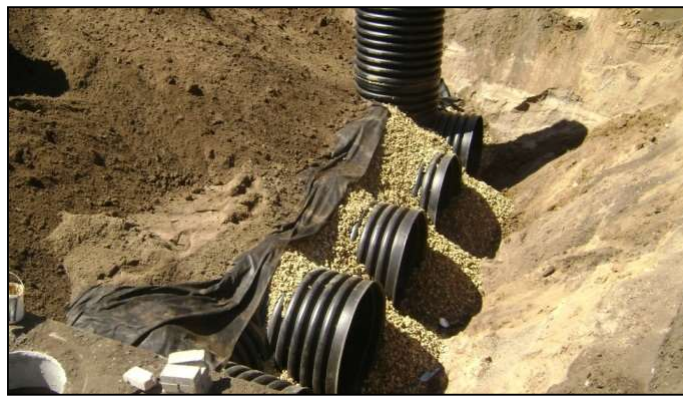
Photo 5-1: St. Albans 48" Perforated HDPE Installation
