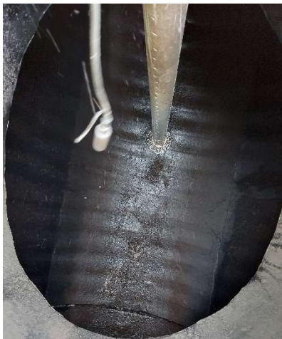
Photo 2-1: Infiltration Gallery Level Monitoring Enclosure
