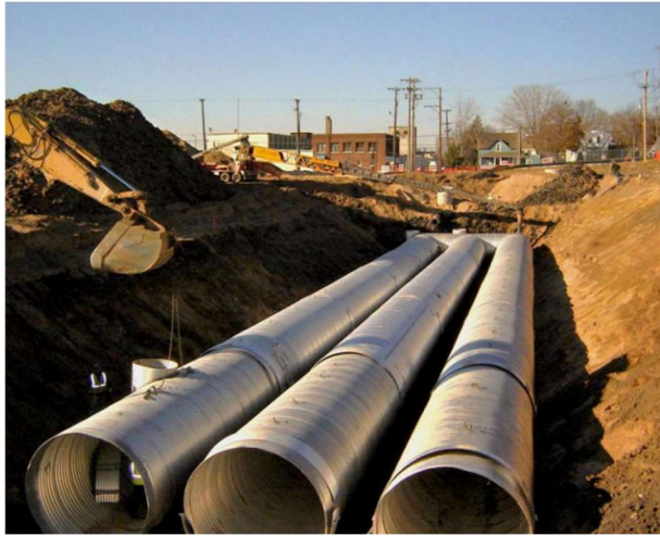
Photo 4-1: Underground Infiltration Chamber (Facing West)
