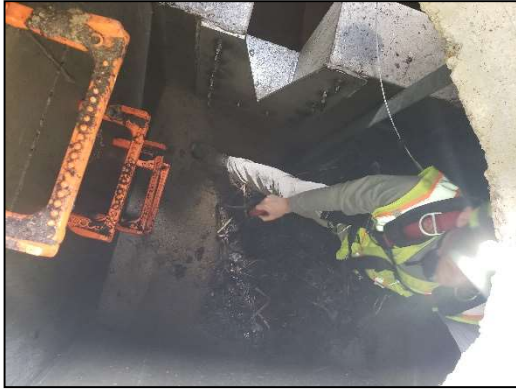
Photo 2-3: Flow Monitoring Module Install Process
