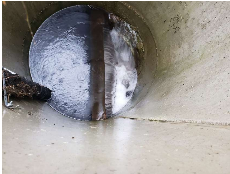
Photo 4-3: Water being conveyed back to the storm sewer from the underground chamber in the outlet control structure.
