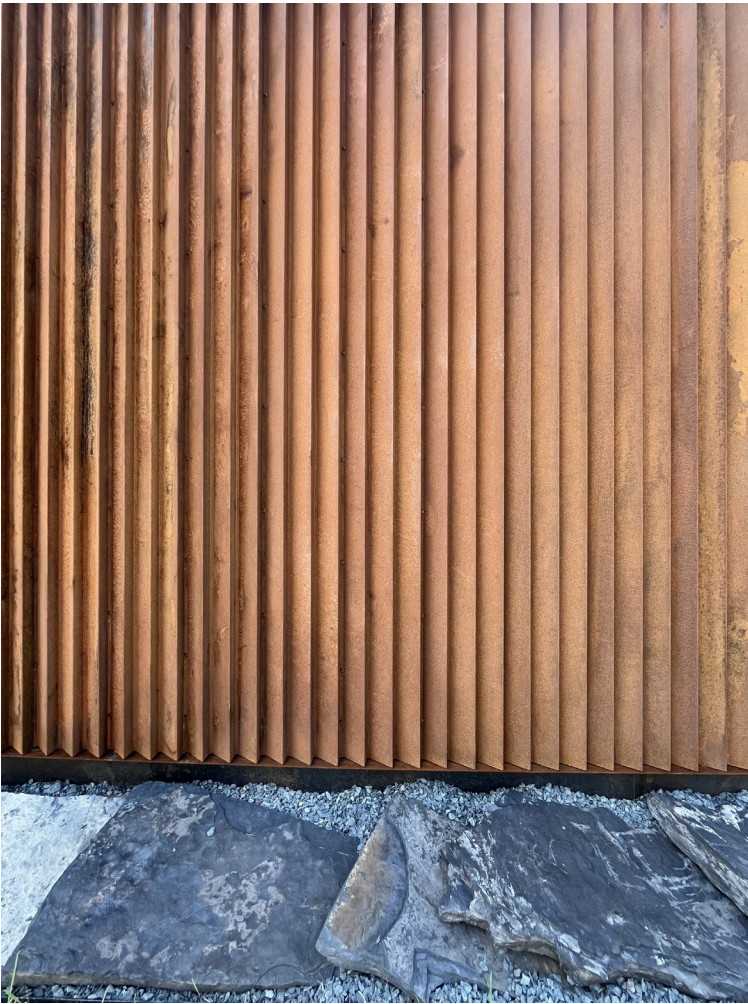
Coreten, Weathering Steel
