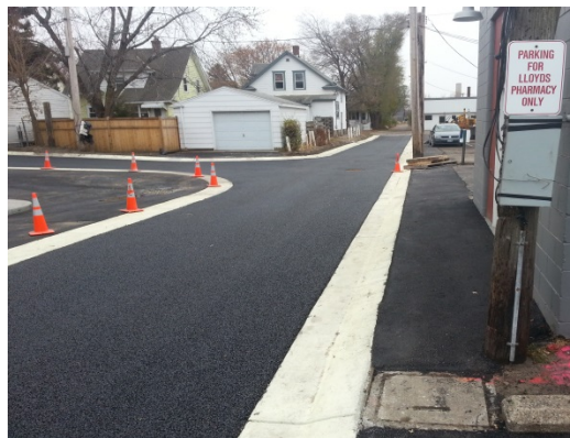
Photo 13-3: Hamline Midway Library porous asphalt (post-construction)
