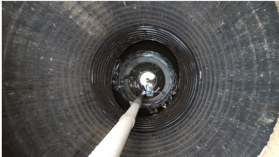
Photo 7-1: Arundel infiltration system access manhole and BMP level monitoring location
