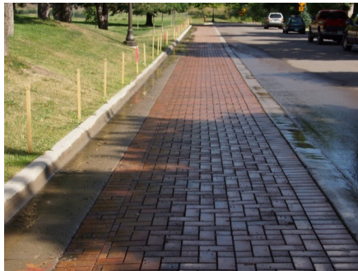
Photo 13-1: Victoria Street pavers
