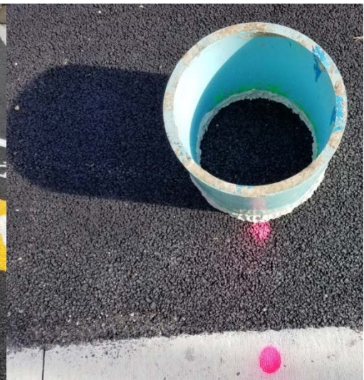
Photo 13-8: Location JS-8 Infiltration Testing
