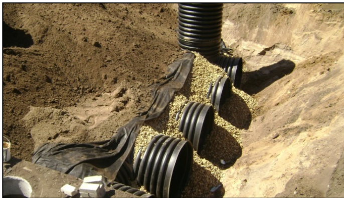
Photo 5-1: St. Albans 48" perforated HDPE installation
