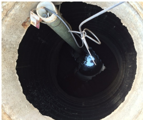
Photo 2-1: Infiltration gallery level monitoring enclosure
