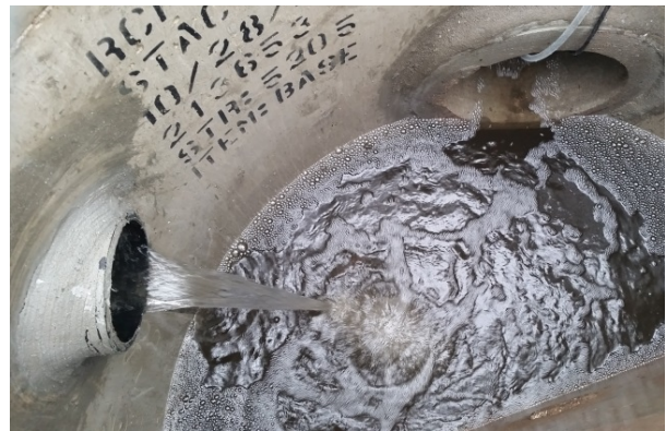
Photo 2-5: Jenks Pond 8" drain tile and outlet pipe within the outlet control structure
