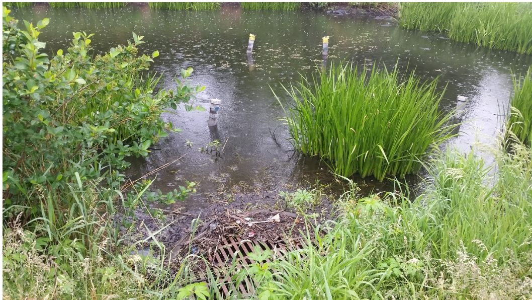
Photo 3-3: Rain garden and IR-32 (underground system) monitoring piezometers (yellow caps), and open grate overflow structure to underground chamber
