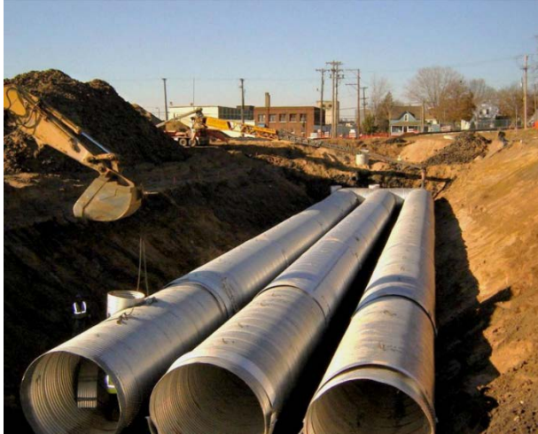
Photo 3-1: Underground infiltration chamber (Facing west)
