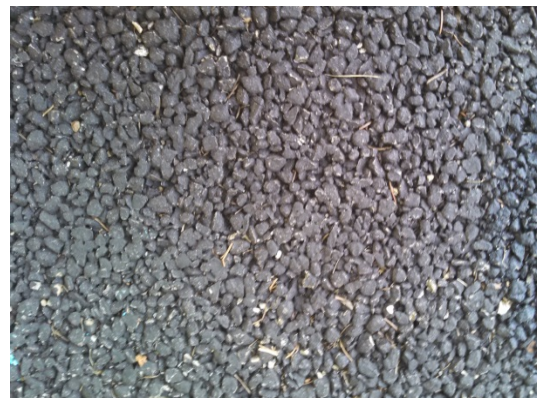
Photo-13-4: Hamline Midway Library porous asphalt
