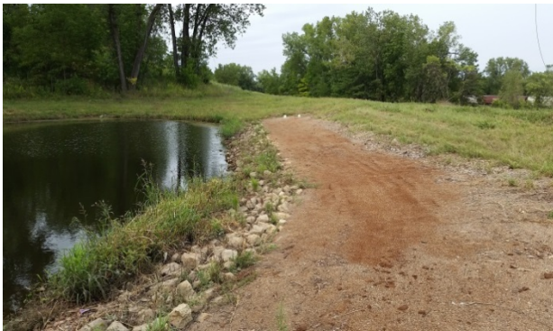
Photo 10-1: Magnolia Pond Iron-Enhanced Sand Bench Sand Bench
