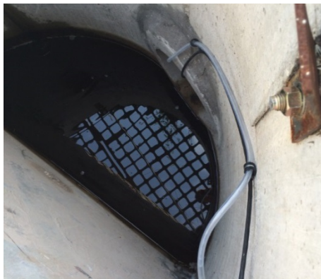
Photo 2-4: Jenks Pond outlet control structure
