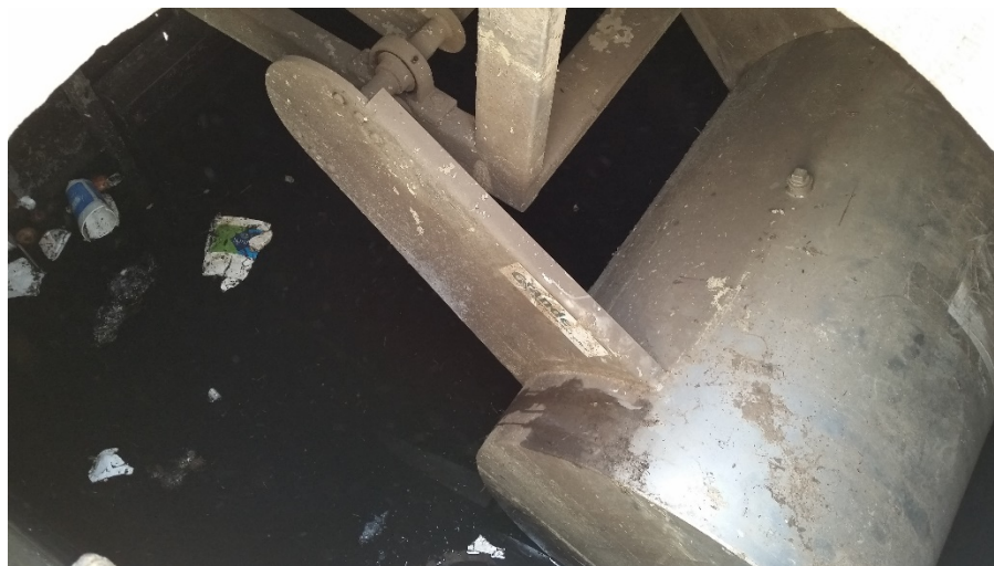
Photo 4-3: System gate valve and float
