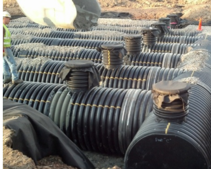
Photo 4-2: 60" Perforated HDPE pipes during system construction
