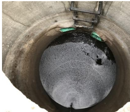
Photo 12-1: Discharge location from Sue Avenue to the 2- 12" infiltration trench pipes
