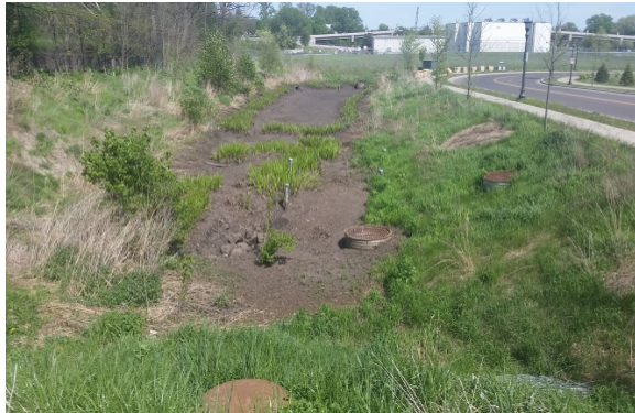
Photo 3-2: Rain garden located above storage chambers (Facing east)
