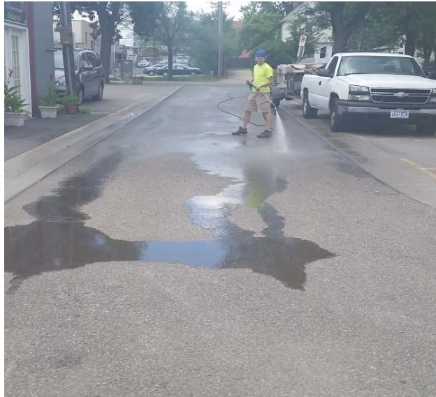
Photo 13-6: Pressure washing maintenance
