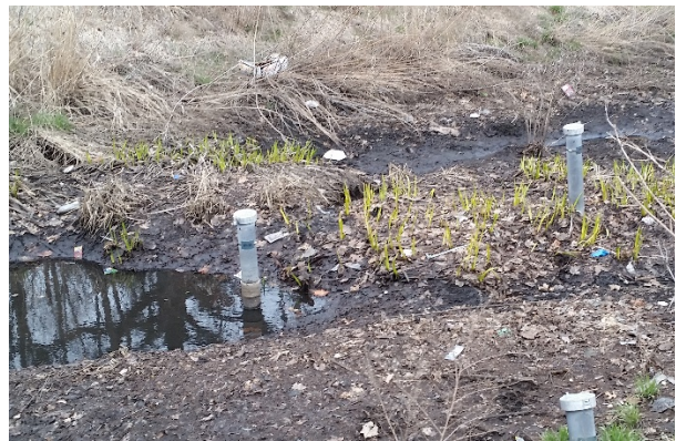
Photo 2-2: Beacon Bluff Rain Garden and in-rock permanent monitoring wells
