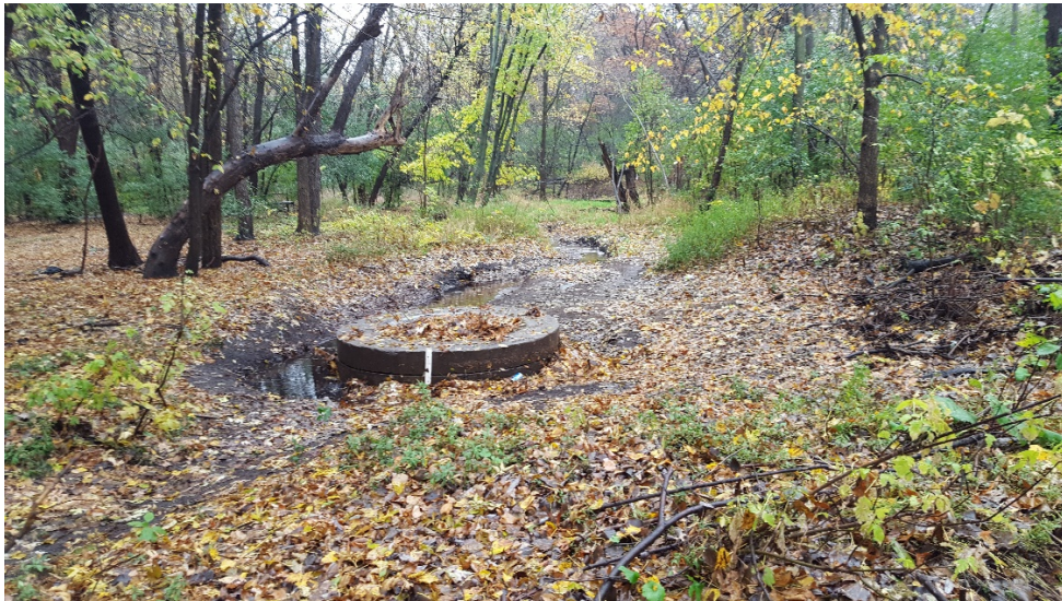
Photo 9-1: Level logger configuration and outlet control structure
