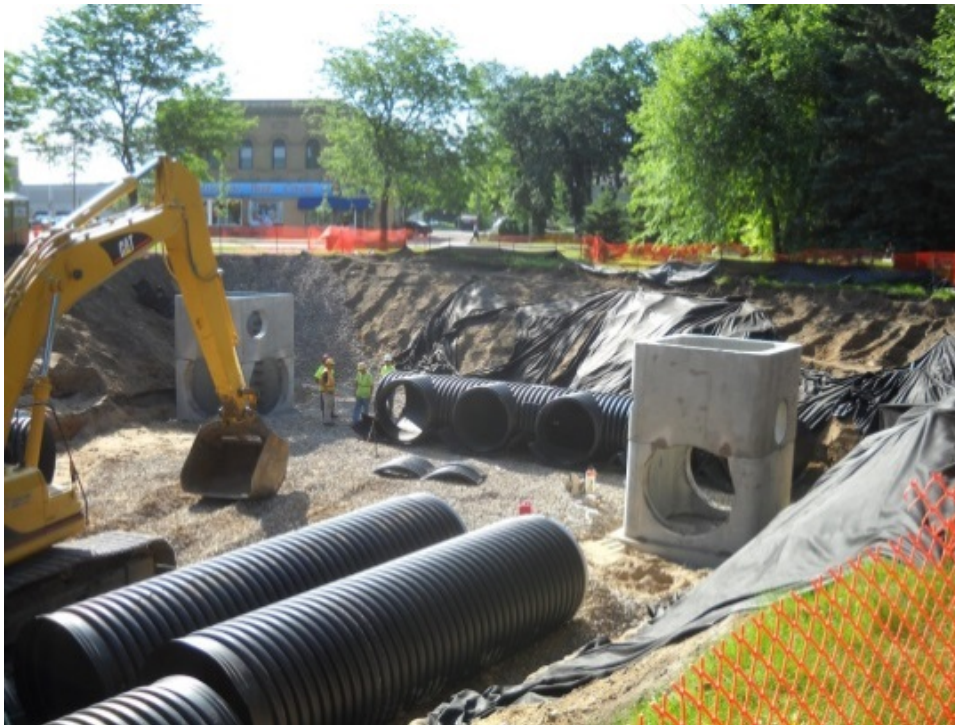
Photo 6-1: Hampden Park BMP Construction
