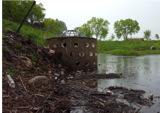
Photo 8-1: Flandrau-Hoyt Pond outlet control structure
