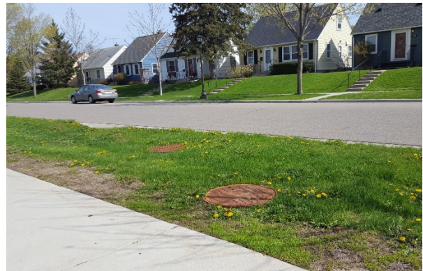
Photo 12-2: Infiltration Trench Monitoring Location (Wordsworth Avenue)
