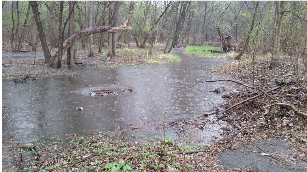
Photo 9-2: Sackett Park Pond outlet control structure – runoff exceeds channel bank and enters flood plain.
