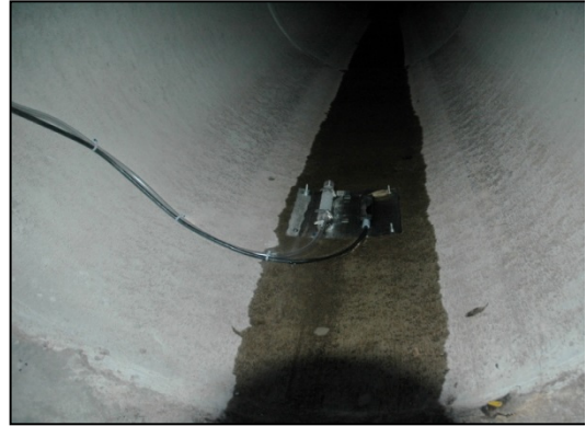
Photo 2-3: Flow sensor in upstream pipe in Beacon Bluff diversion structure
