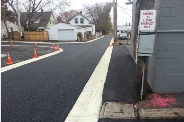
Photo 14-5: Hamline Midway Library porous asphalt (post-construction)
