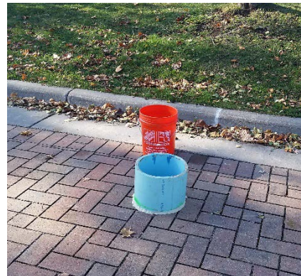
Photo 14-2: Victoria Street infiltration testing
