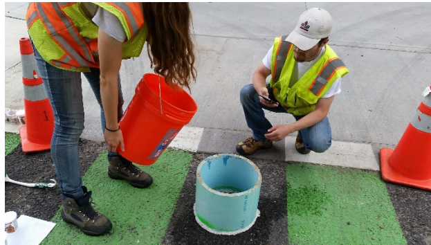
Photo 2-11: Permeable Pavement Infiltration Test
