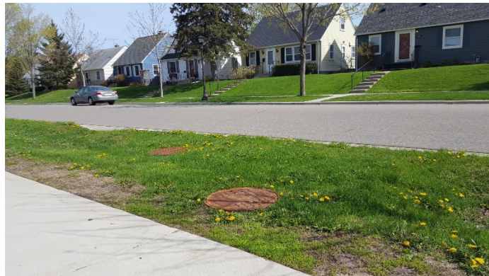
Photo 13-2: Infiltration Trench Monitoring Location (Wordsworth Avenue)
