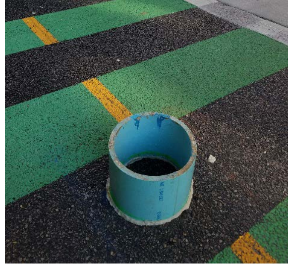
Photo 14-10: Jackson Street Infiltration Test
