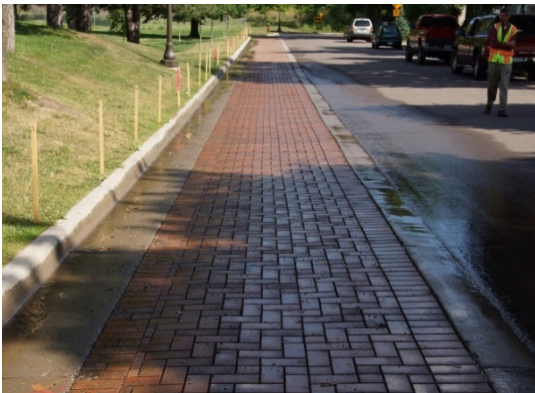
Photo 14-1: Victoria Street pavers
