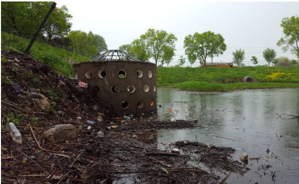
Photo 9-1: Flandrau-Hoyt Pond outlet control structure
