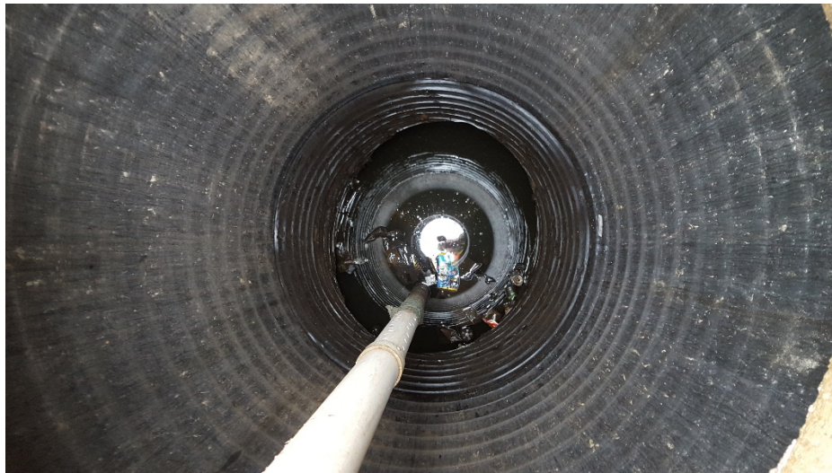
Photo 8-1: Arundel infiltration system access manhole and BMP level monitoring location
