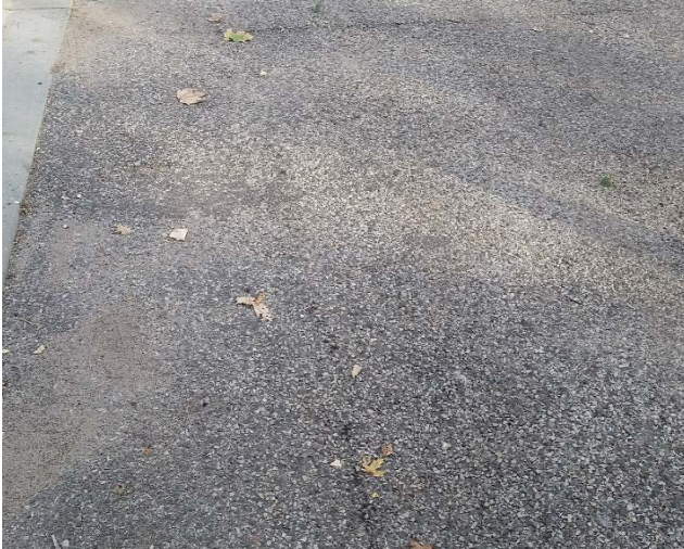
Photo 14-7: Near IR-4, compaction & heavy silt accumulation
