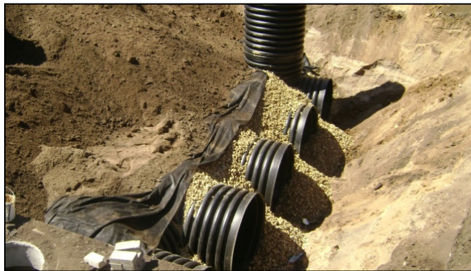
Photo 6-1: St. Albans 48" perforated HDPE installation
