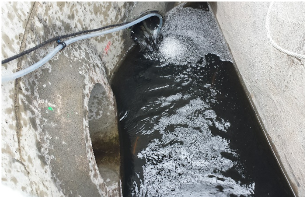
Photo 2-6: Jenks Pond 8" drain tile and outlet pipe within the outlet control structure
