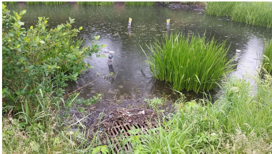
Photo 4-3: IR-31 (Rain garden) and IR-32 (underground system) monitoring piezometers (yellow caps), and open grate overflow structure to underground chamber
