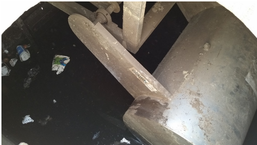
Photo 5-3: System gate valve and float
