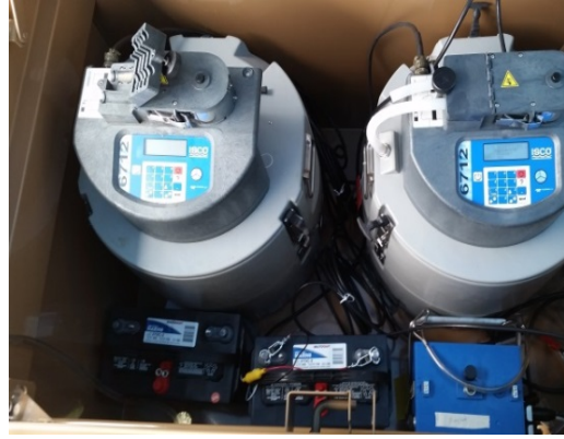
Photo 2-9: Maryland Pond sampler configuration
