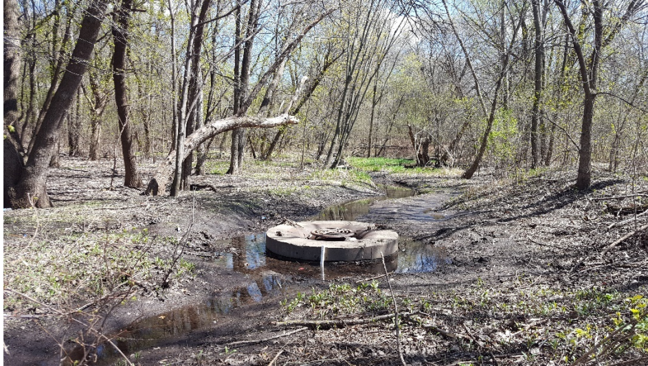
Photo 10-1: Level logger configuration and outlet control structure
