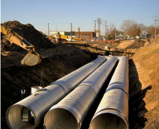
Photo 4-1: Underground infiltration chamber (Facing west)
