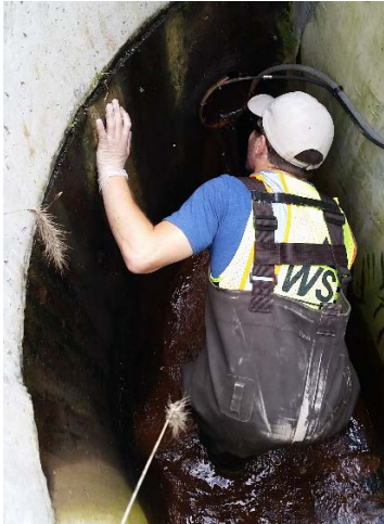
Photo 11-3: Maryland Pond sensor/intake inspection
