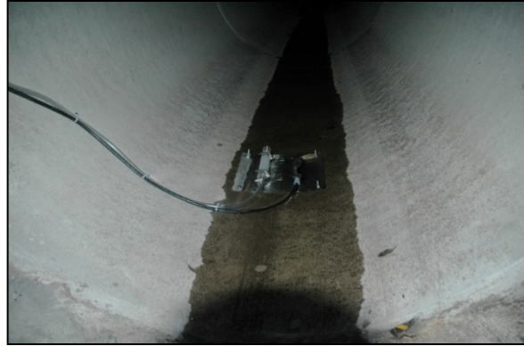
Photo 2-4: Flow sensor in upstream pipe in Beacon Bluff diversion structure
