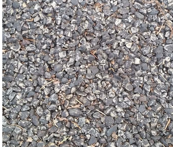
Photo 14-8: IR-6, less compaction & silt
