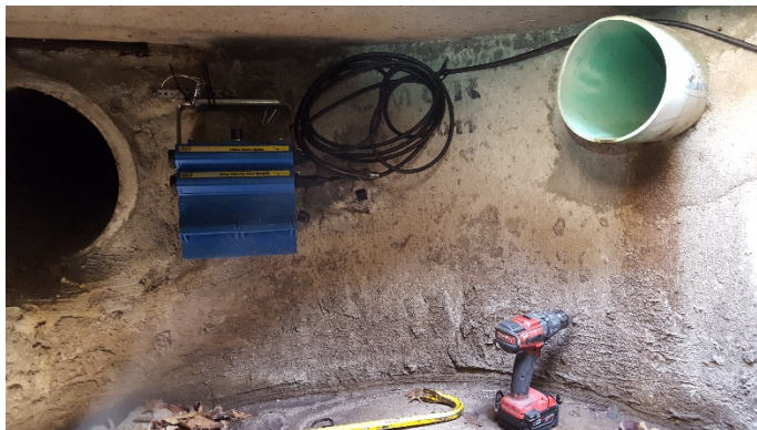
Photo 6-2: St. Albans flow meter installation at the University BMP inlet
