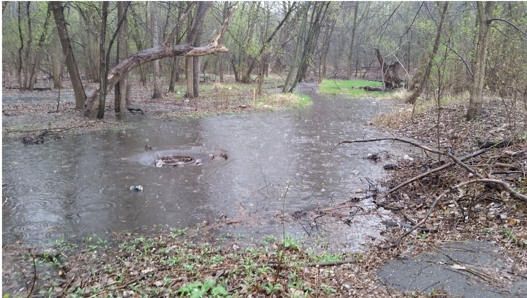
Photo 10-2: Sackett Park Pond outlet control structure – runoff exceeds channel bank and enters flood plain (4/19/2017).
