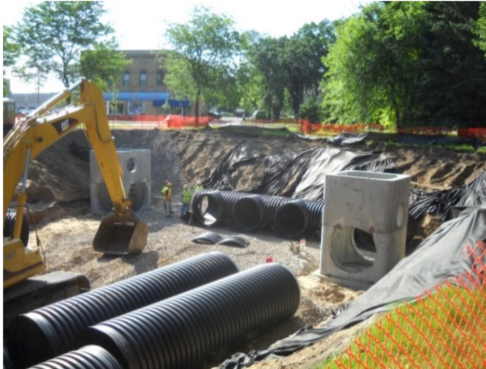
Photo 6-1: Hampden Park BMP Construction
