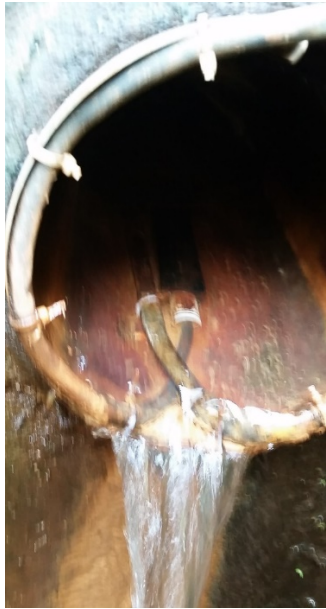
Photo 11-5: Iron Precipitate at drain tile outlet to OCS
