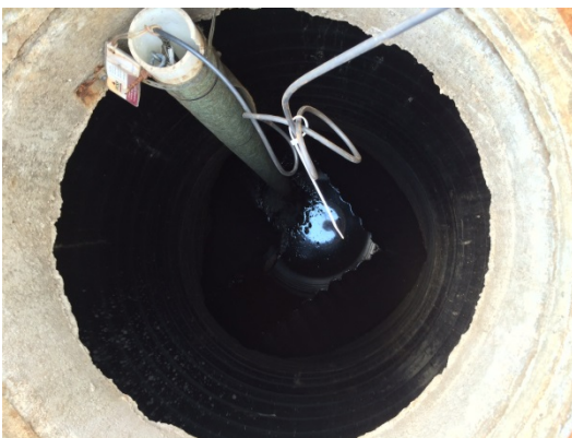
Photo 2-1: Infiltration gallery level monitoring enclosure
