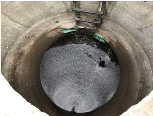
Photo 13-1: Discharge location from Sue Avenue to the 2- 12” infiltration trench pipes
