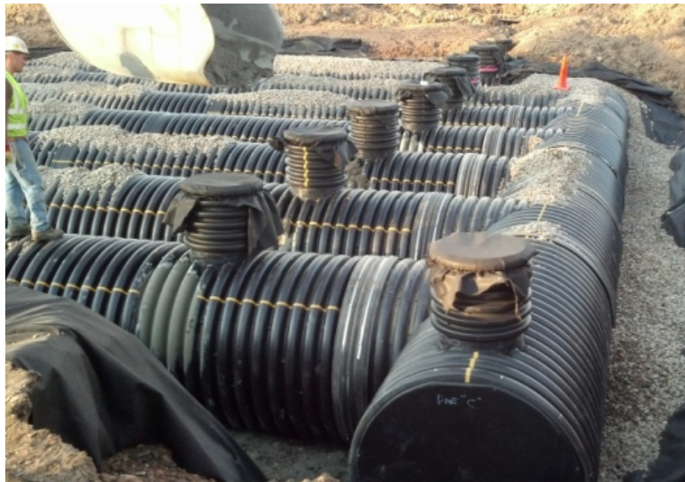
Photo 5-2: 60" Perforated HDPE pipes during system construction
