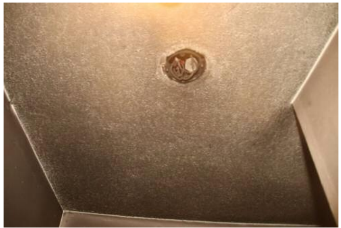
This rather small fire consumed most of the oxygen in the apartment and enough toxic smoke to kill the resident. The hardwired smoke alarm on the right had been disabled.
