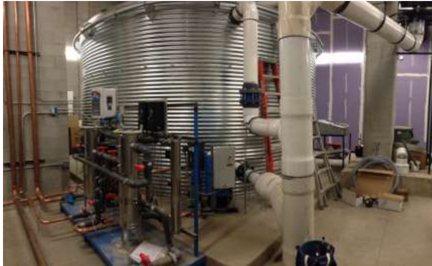
CHS field cistern. Photo courtesy of City of Saint Paul staff.
