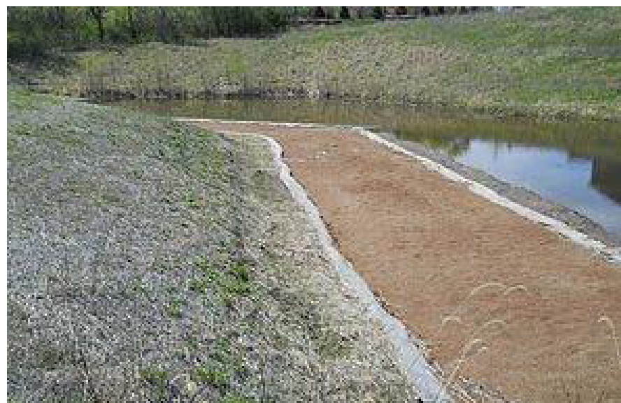
Figure 4: Iron-enhanced sand filter bench at Prior Lake, Minnesota
