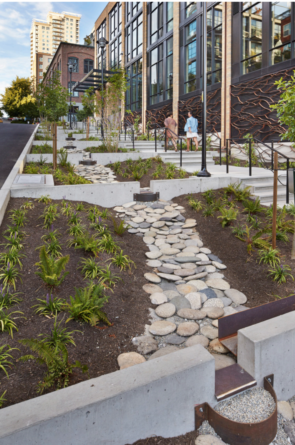
STORMWATER CHANNEL
