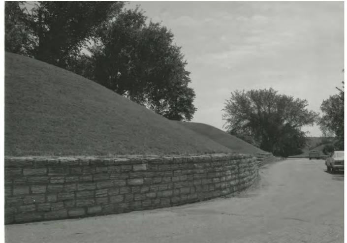
Figure 2.25. Stone retaining walls were constructed at the edges of the mounds in the 1930s by CCC/WPA. (Ramsey County Historical Society Cat.#1.2198, 1975 ca.).
