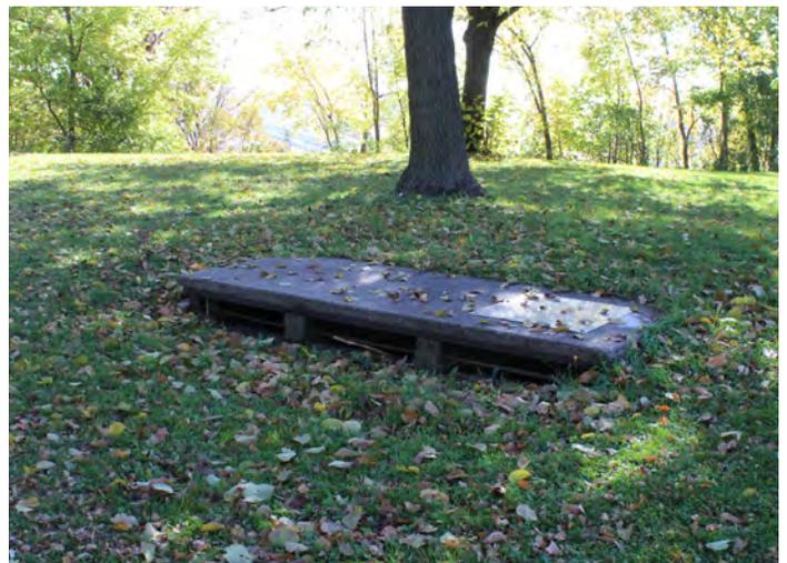
Figure 3.10. Inlet within the picnic area drains water from the perched wetland soils (QEA, 2018).
