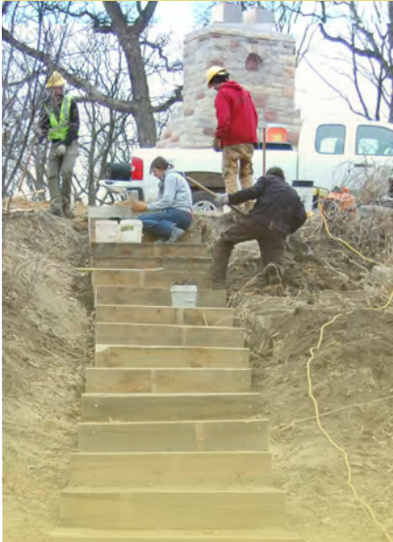
Installing the timber staircase. Photo: City of Saint Paul
