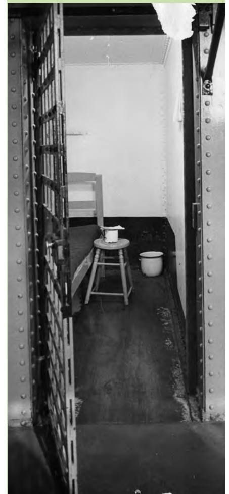
Workhouse cell circa 1950. Note the slop bucket in the corner. Photo: Minnesota Historical Society
