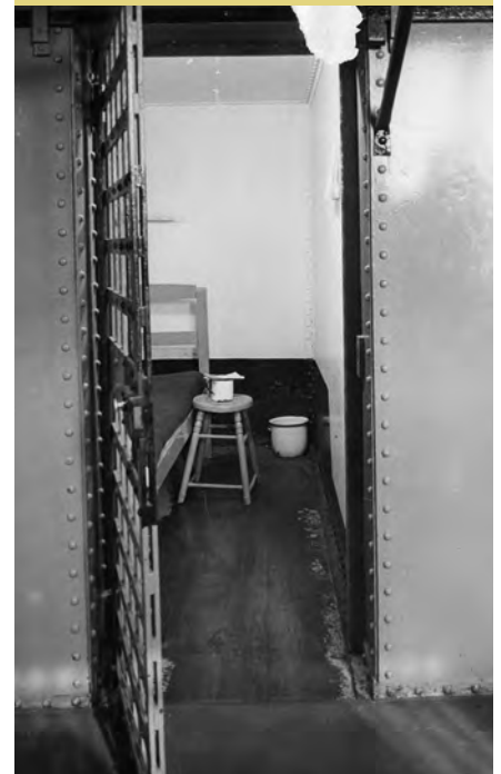
Workhouse cell circa 1950. Note the slop bucket in the corner. Photo: Minnesota Historical Society
