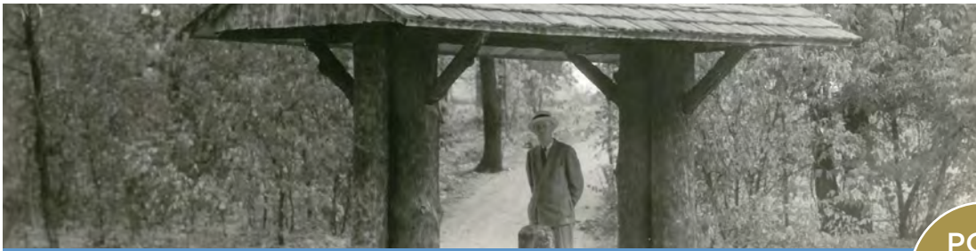
W. LaMont Kaufman at fireplace entrance gate, circa 1936. Photo: City of Saint Paul
