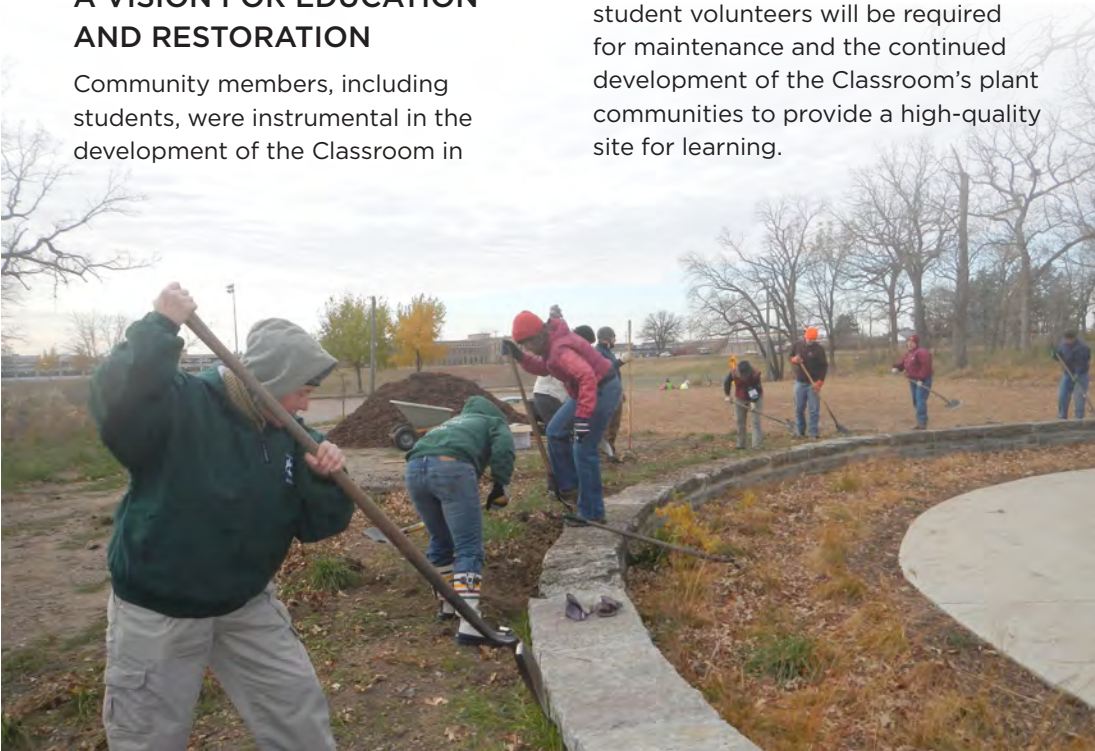
Volunteers helped restore the Joyce Kilmer Memorial Fireplace. Photo: City of Saint Paul
