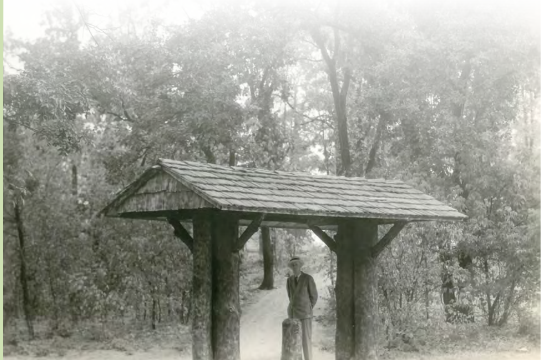
W. LaMont Kaufman at fireplace entrance gate, circa 1936. Photo: City of Saint Paul
