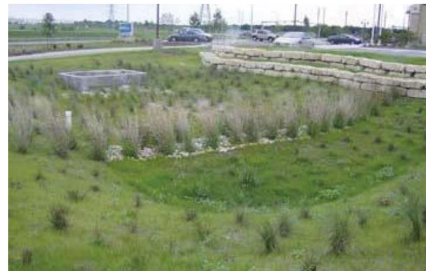
Figure 3: Typical bio-filtration basin
