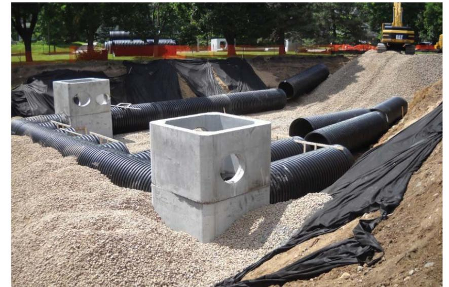
Figure 2: Large scale underground infiltration BMP at Hampden Park
