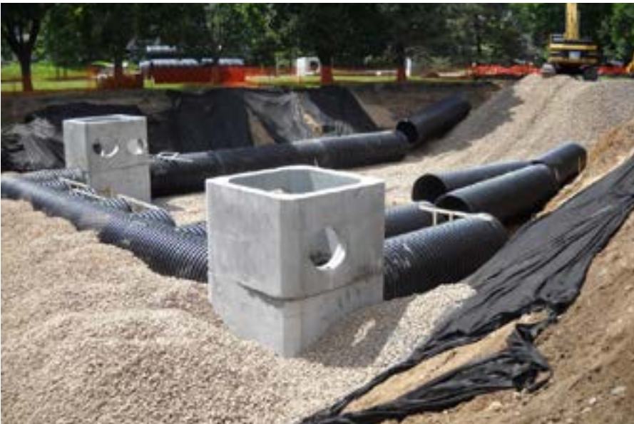
Figure 2: Large scale underground infiltration BMP at Hampden Park
