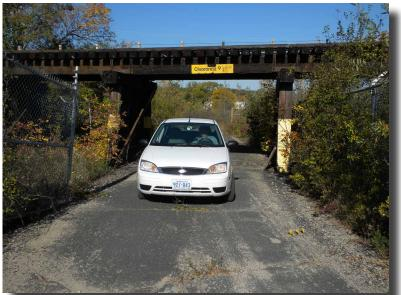
Existing RR bridge - provides important connection for pedestrians/bicycles between park. Maintain access, but important to note low clearance (9') does not allow fire access to southern side of Victoria Park. Explore utilizing at-grade crossing to SW for emergency vehicular access.
