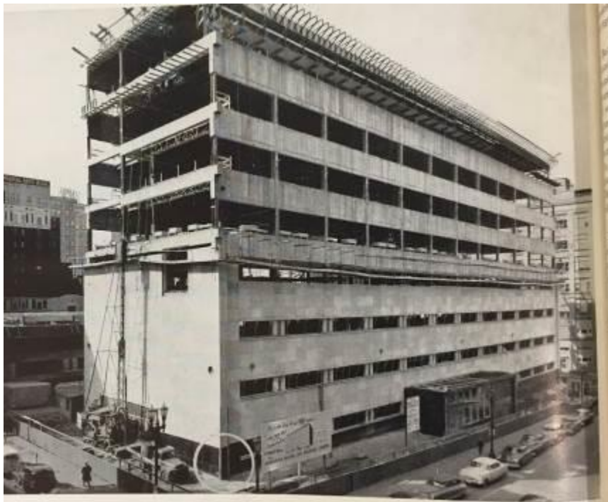
Figure 15. Construction photos documenting Minnesota Mutual. Application (Official Publication of the Minnesota Mutual Life Insurance Company Saint Paul, Minnesota) , March 1954 (steel) and October 1954 (concrete). Minnesota Historical Society Collections.
