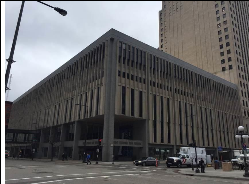
First National Bank of Saint Paul Addition 332 Minnesota Street Haarstick, Lundgren and Associates 1971
