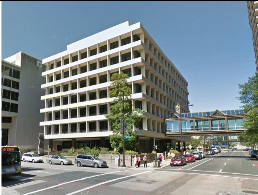
Farm Credit Banks Building 375 Jackson Street Bergstedt, Wahlberg and Wold 1967
